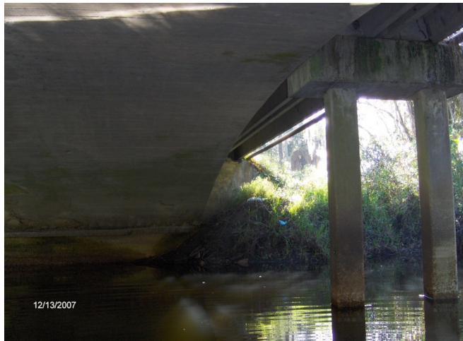
Figure 4 – Arch widened from below
