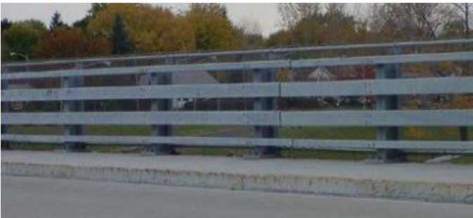
Figure 9.6 Metal Tube Bridge Rails (Steel, Aluminum)
