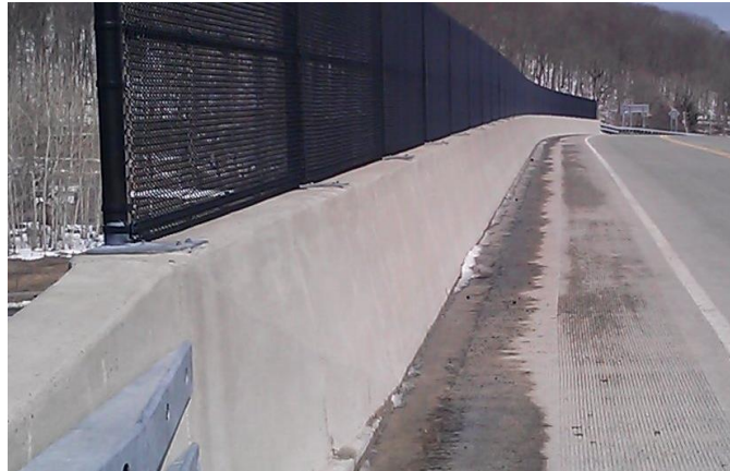
Figure 9.10 Single Slope Concrete Barrier
