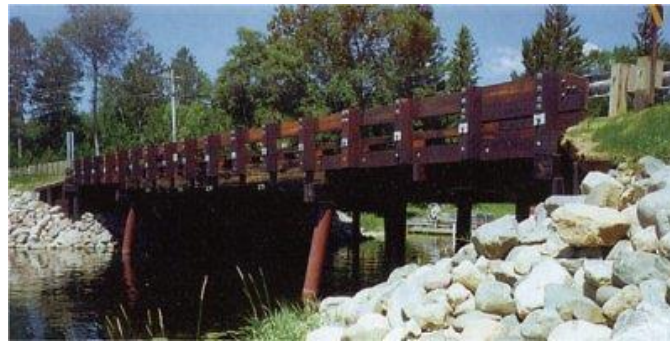
Figure 9.11 Timber Bridge Railing (Wood)
