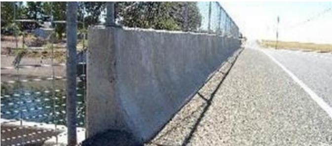
Figure 9.8 New Jersey Barrier (Concrete)
