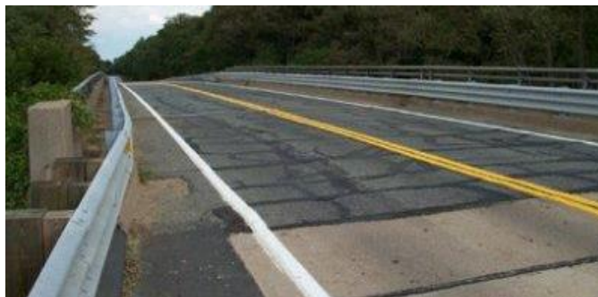
Figure 9.5 Thrie Beam Bridge Railing (Steel)
