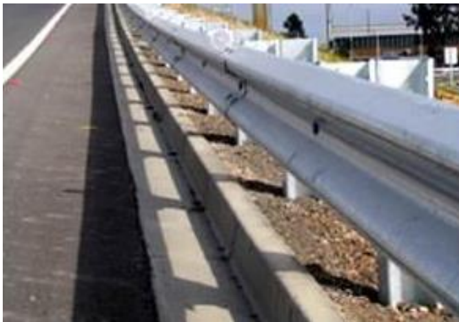
Figure 9.2 Metal Beam Guard Rail
