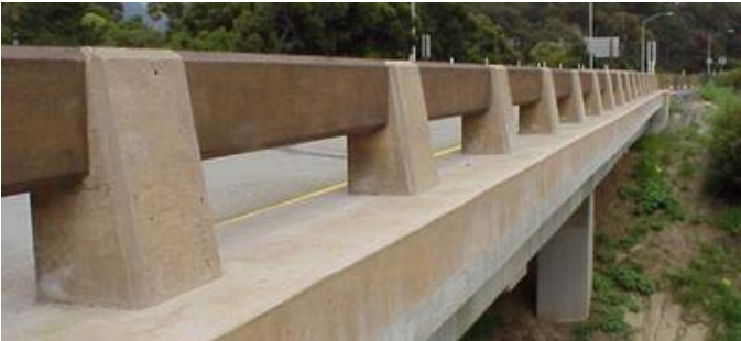
Figure 9.7 Vertical Concrete Parapet (Open or Closed) (Concrete)
