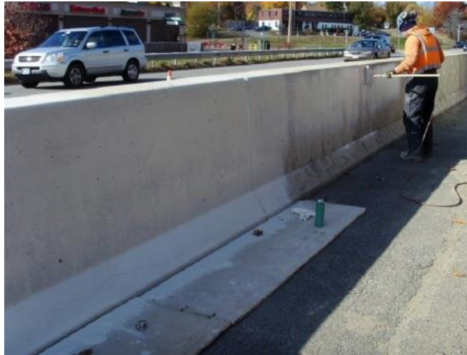
Figure 9.13 Application of Elastomeric Paint on Alkali-Silica Reactivity-Affected Barrier
