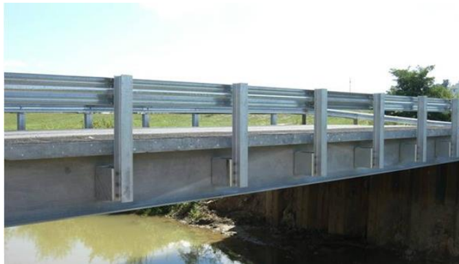
Figure 9.4 W-Beam Bridge Railing (Steel)
