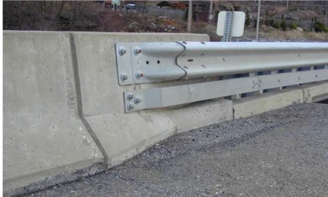
Figure 9.1 Jersey Barrier and Guard Rail
