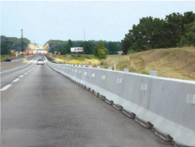
Figure 9.9 F-Shape Barrier
