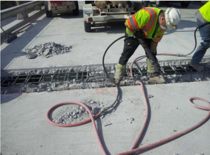
Figure 8.7 Conflicts with Bottom Shear Studs and K bars in Diaphragms
