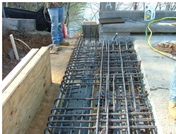
Figure 8.38 Construction Photo of Backwall Rebar
