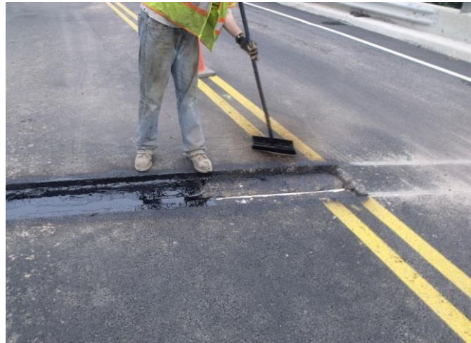
Figure 8.24 Asphaltic Plug Joint with Binder Placed Atop Backer Rod Prior to Bridging Plate Installation
