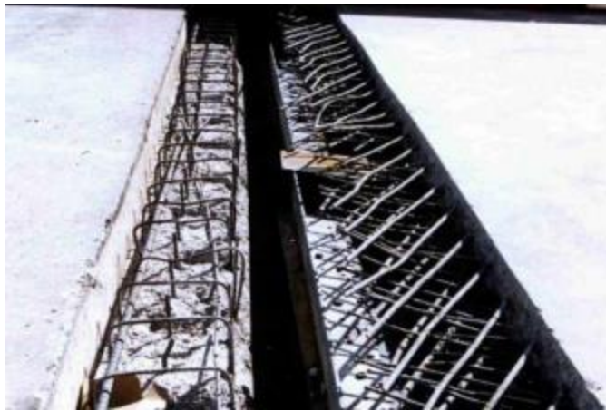
Figure 8.32 Saw Cut and Remove Concrete to Create Block-Out
