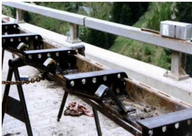
Figure 8.33 Rehab Plates and Add Anchors
