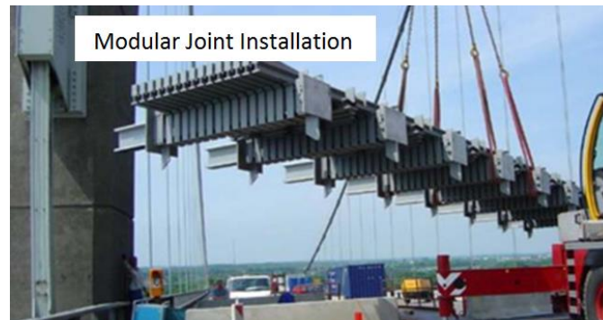
Figure 8.11 Installation of Modular Expansion Joint
