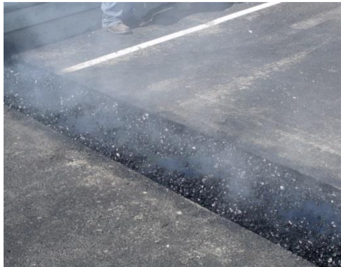
Figure 8.25 Plug Installation Showing Coated Aggregate and Binder
