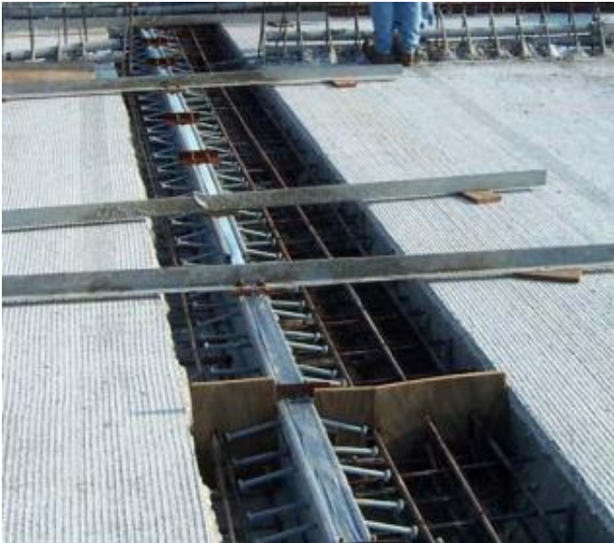
Figure 8.29 New Strip Seal Joint
