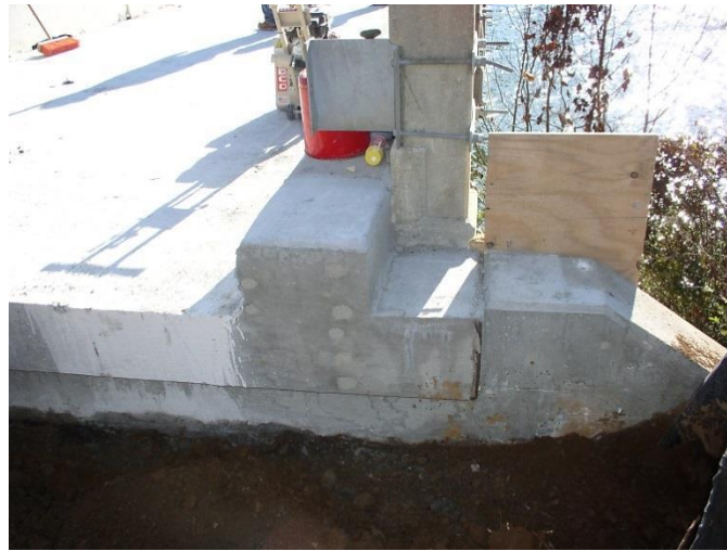
Figure 8.39 Construction Photo of Completed Slab over Backwall at Bridge Railing
