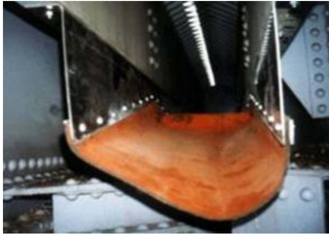
Figure 8.17 Finger Joint Trough Assembly
