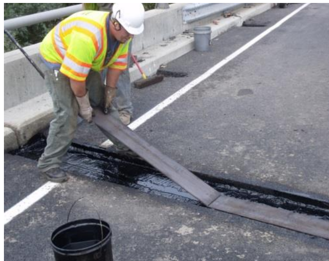
Figure 8.26 Bridging Plate Installation
