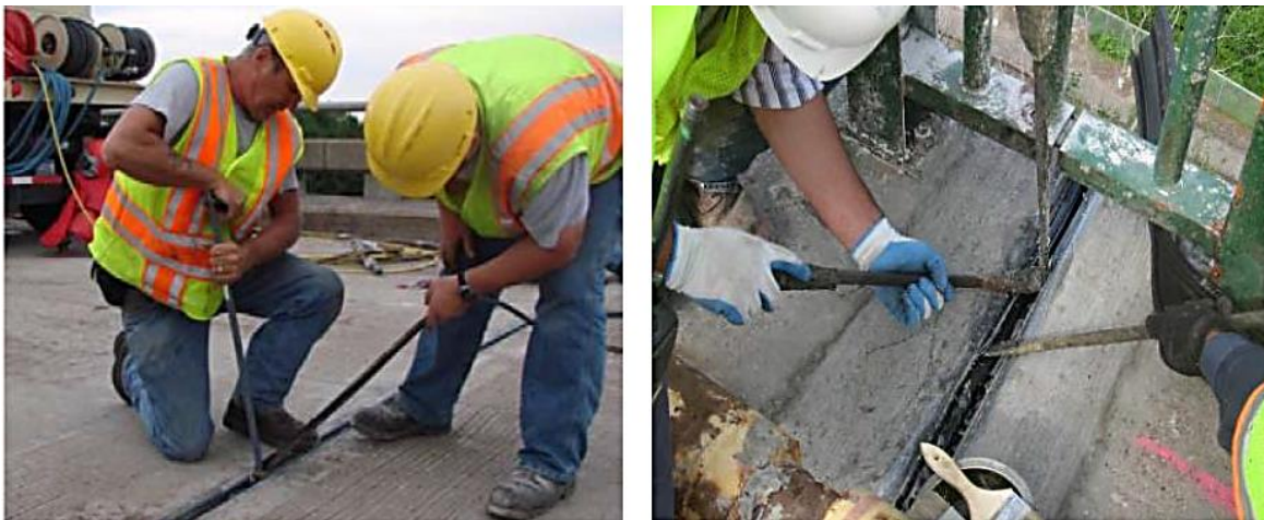
Figure 8.28 Removing the Old Gland (left) and Installation of New Gland (right)
