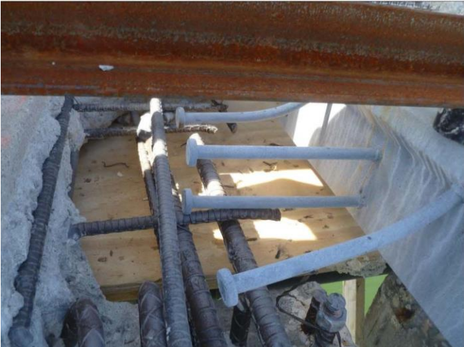
Figure 8.8 Bent Shear Studs
