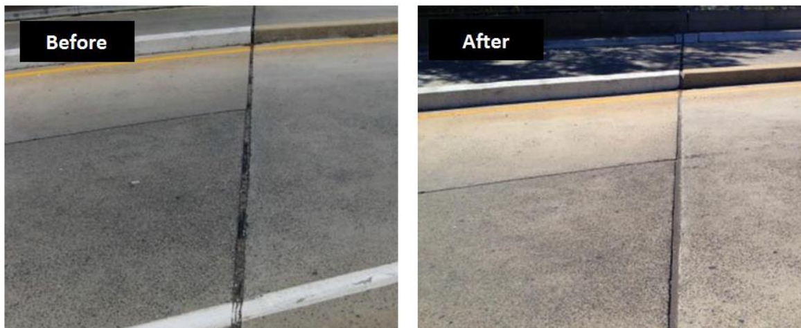
Figure 8.19 Before (left) and After (right) Photos of Silicone Sealant Installation
