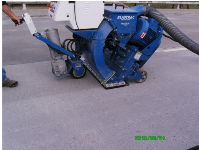
Figure 7.32 Preparing the Deck with Shot Blasting (Courtesy of Kwikbond Polymers)
