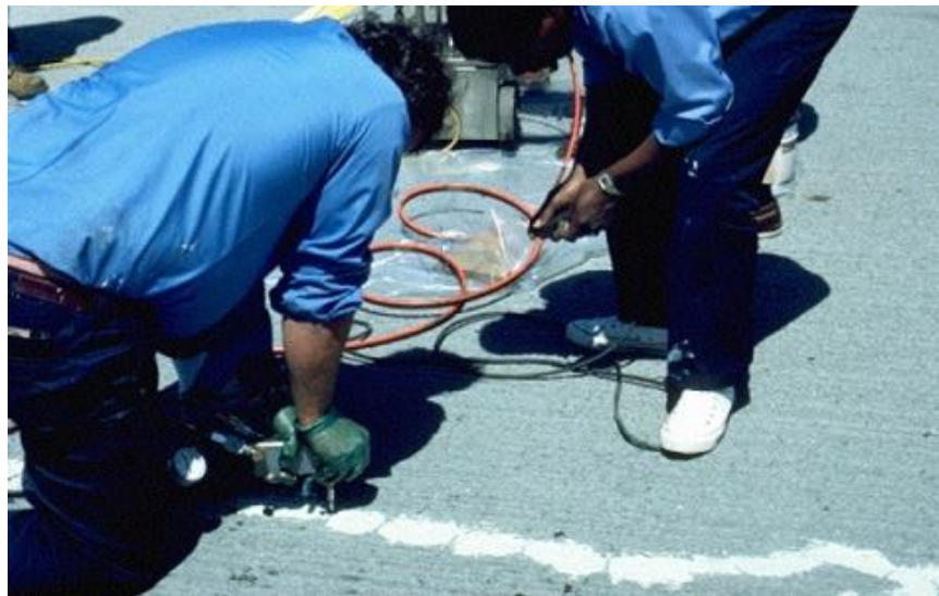
Figure 7.11 Epoxy Injection Repair (Courtesy of Virginia DOT)
