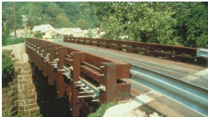
Figure 7.48 Stress-Laminated Deck with Stressing Bolts Shown
