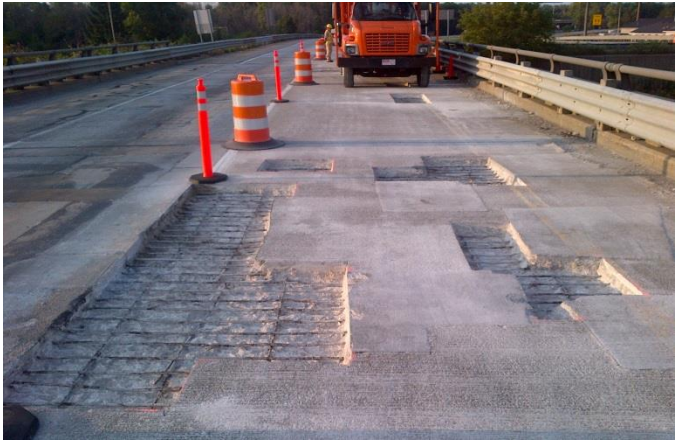
Figure 7.22 Prepared Patch Areas (Courtesy of MDOT)
