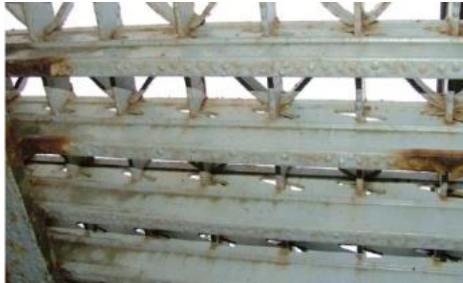
Figure 7.39 Slotted Grid Deck
