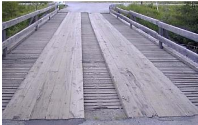
Figure 7.50 Typical Timber Deck Runners
