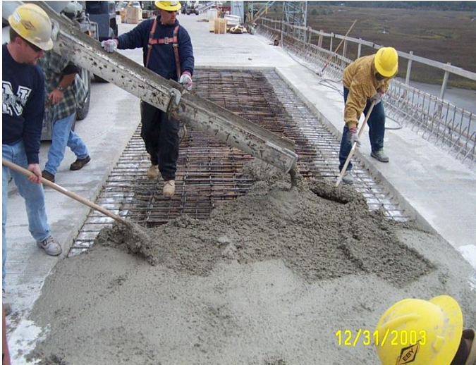
Figure 7.23 Concrete Placement
