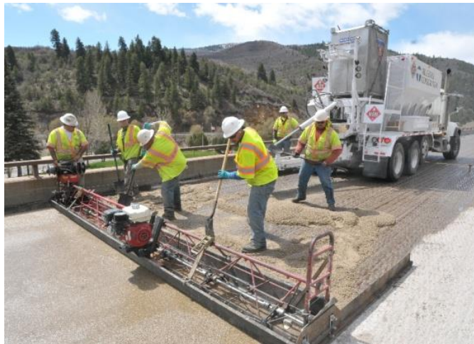
Figure 7.29 Placing the New Polyester Concrete (Courtesy of Truesdell Construction)
