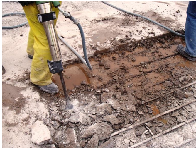
Figure 7.19 Concrete Removal (Courtesy of MDOT)
