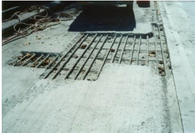
Figure 7.35 Localized Repair Area
