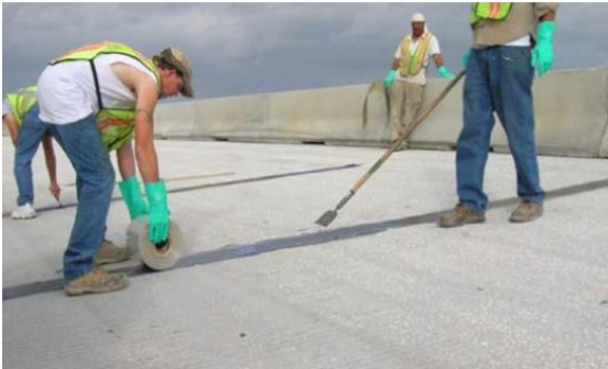
Figure 7.12 Surface Epoxy Sealing with Optional Fabric (Courtesy of Virginia DOT)
