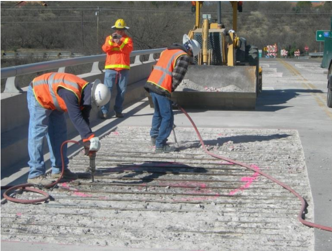
Figure 7.27 Removing the Delaminated Concrete (Courtesy of Kwikbond Polymers)
