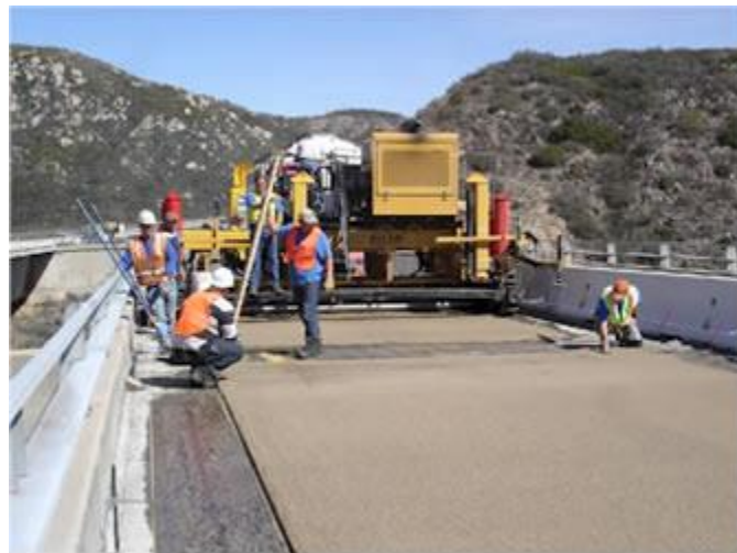
Figure 7.33 Placing the Concrete Overlay (Courtesy of Truesdell Construction)
