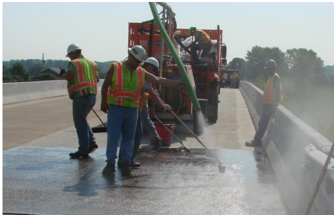
Figure 7.15 Broadcasting Sand (Aggregate) (Courtesy of MDOT)
