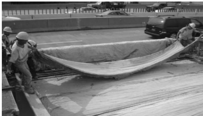
Figure 7.30 Curing the Concrete
