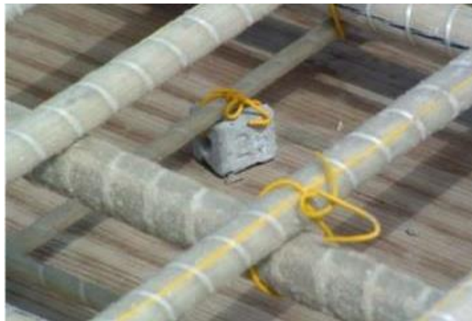
Figure 7.5 FRP Deck Bars (Courtesy of Hughes Bros)
