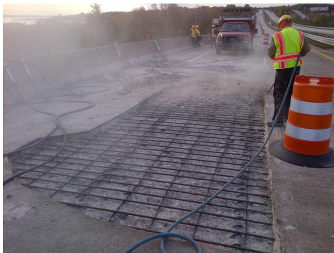
Figure 7.21 Cleaning with Compressed Air (Courtesy of MDOT)
