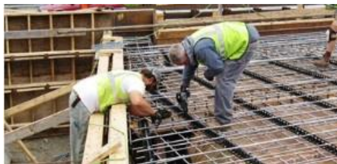
Figure 7.3 Stainless Steel Reinforcing (Courtesy of FHWA)
