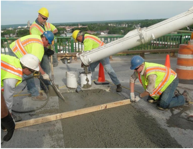
Figure 7.24 Vibration and Finishing (Courtesy of MDOT)
