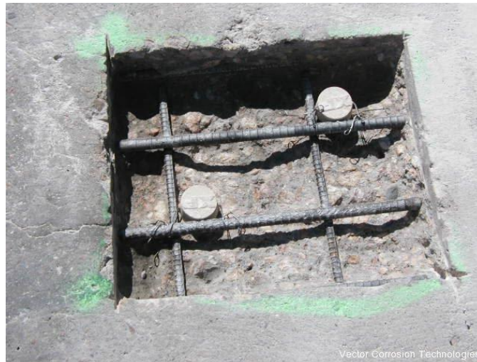
Figure 7.36 Placement of Galvanic Anodes (Courtesy of Vector Corrosion Technologies)
