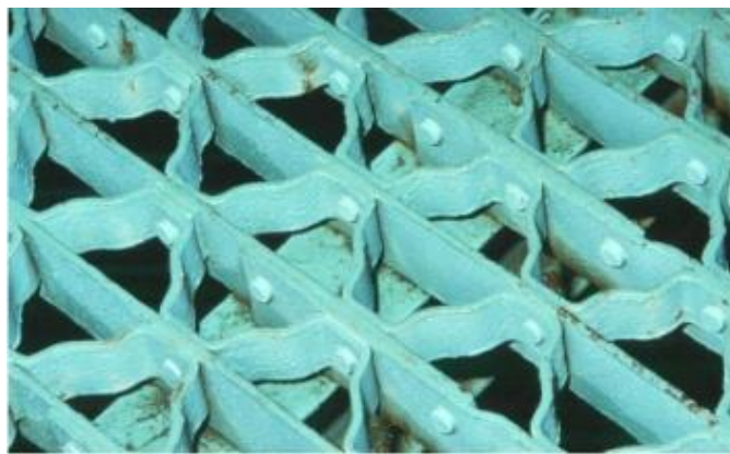
Figure 7.38 Riveted Steel Grid Deck
