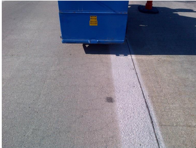
Figure 7.13 Shot Abrading Deck Preparation (Courtesy of MDOT)
