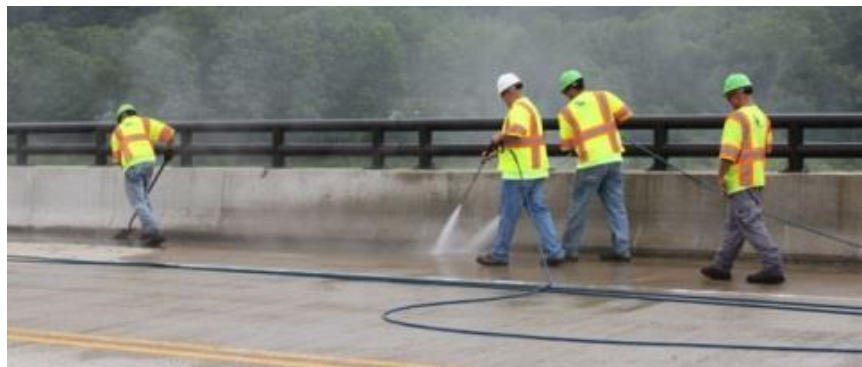
Figure 7.10 Bridge Washing (Courtesy of DBI Services)
