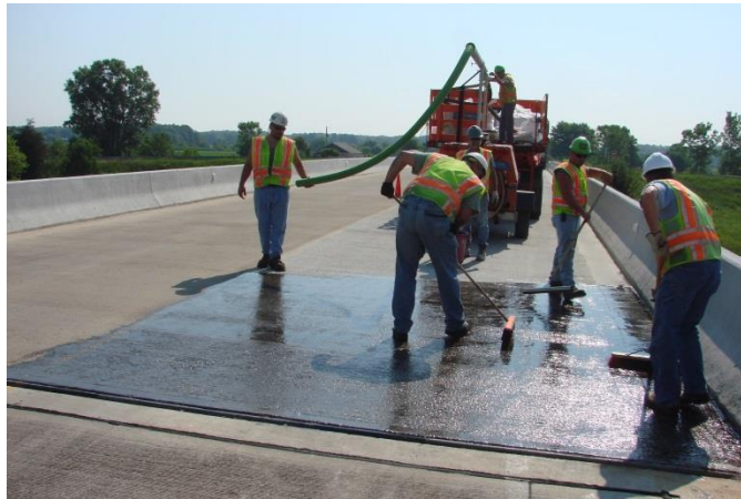
Figure 7.14 Sealer Application (Courtesy of MDOT)
