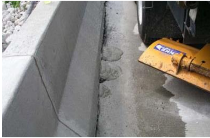
Figure 6.11 Mudjacking Slurry Blowing Out at Barrier (Courtesy of Missouri DOT)
