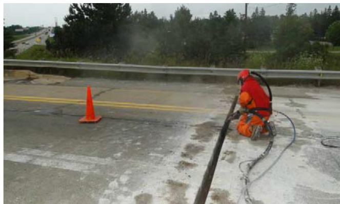
Figure 6.21 Sandblasting the Vertical Surfaces of the Joint Opening (Courtesy of MDOT)
