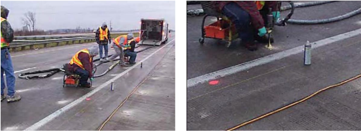
Figure 6.12 Injecting Expansive Polyurethane under Approach Slab (Courtesy of Iowa DOT)
