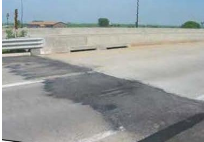
Figure 6.8 Asphalt Ramp Placed at the Approach Slab
