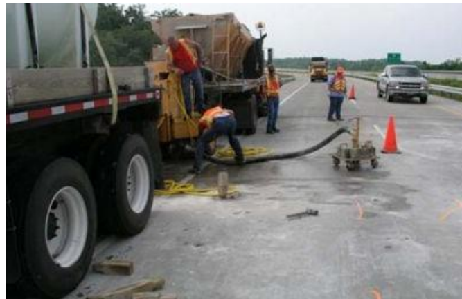
Figure 6.10 Mudjacking Slurry Pumped Under Approach Slab (Courtesy of Missouri DOT)
