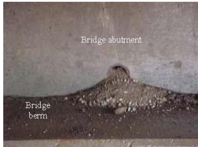
Figure 6.7 Weepholes Filled with Backfill Material (Courtesy of Iowa DOT)
