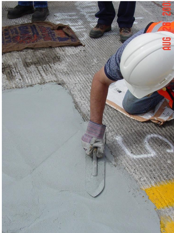
Figure 5.68 Trowel Finish on a Deck Patch
