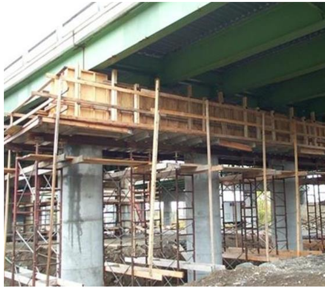
Figure 5.49 Forming for a Pier Cap Repair
