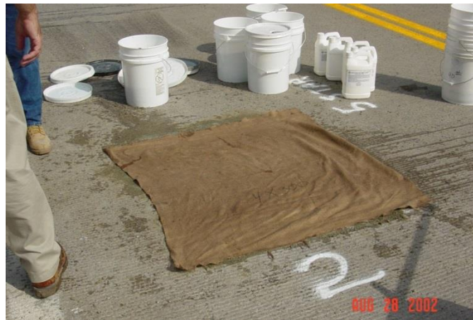
Figure 5.70 Wet Cure of a Small Deck Patch Using Pre-Soaked Burlap
