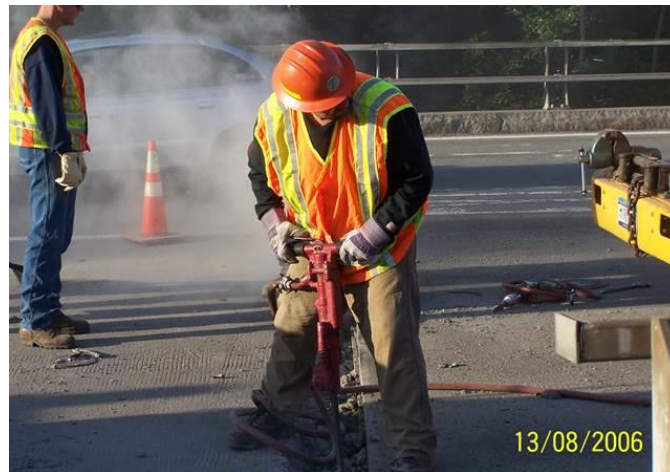
Figure 5.42 Hammering Concrete
