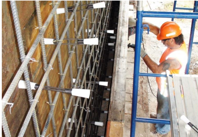
Figure 5.47 Forming for a Wingwall Repair
