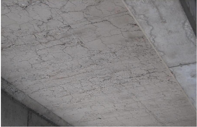
Figure 5.9 Map Cracking
