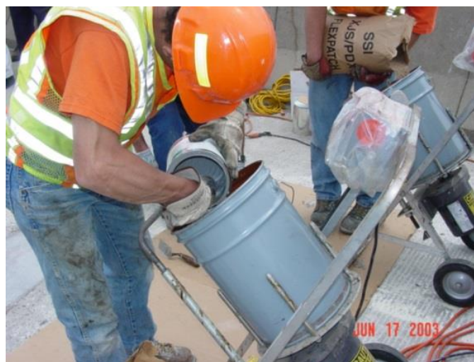
Figure 5.56 Power Mixers for Larger Patches
