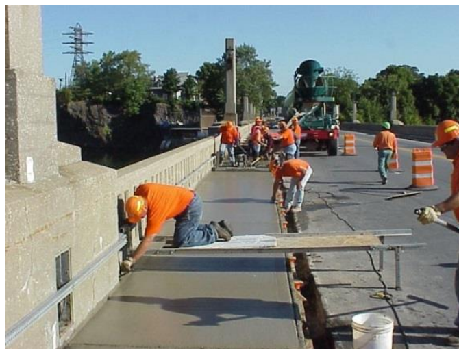
Figure 5.69 Using a Bridge for Concrete Finishing
