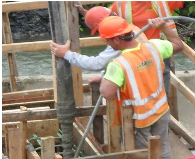
Figure 5.52 Pumping with Elephant Trunk and Consolidating with Vibrator
