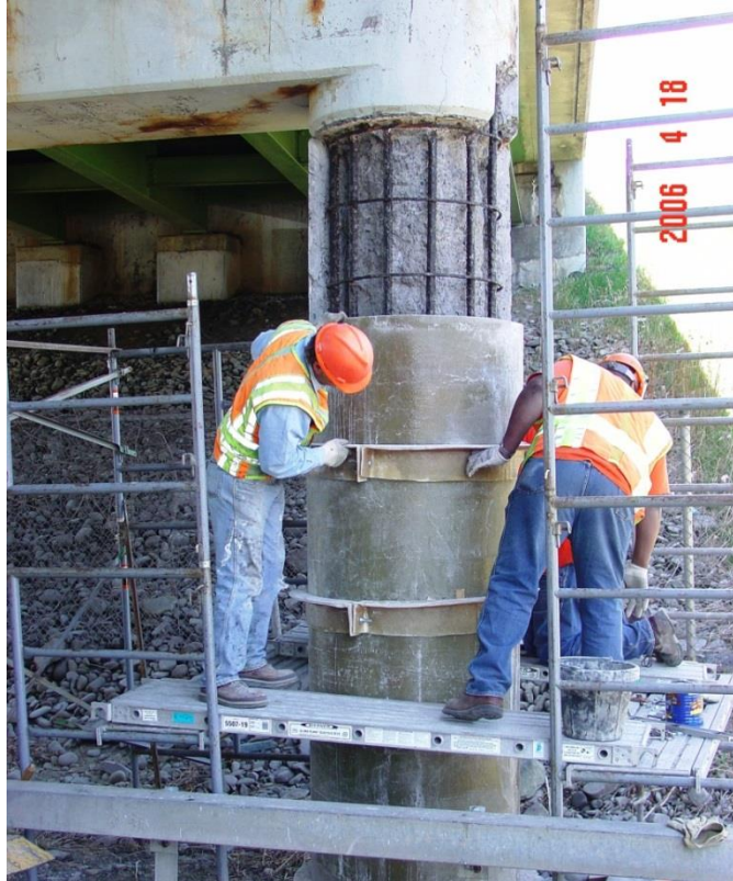
Figure 5.48 Manufactured Forms for Columns
