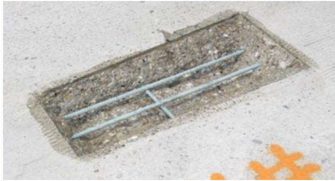
Figure 5.41 Saw cut Around Reinforcing Steel with Concrete Removed on an Angle
