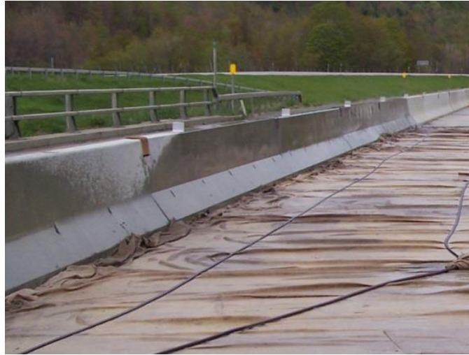
Figure 5.72 Wet Cure with Pre-Soaked Burlap for a Large Deck Repair
