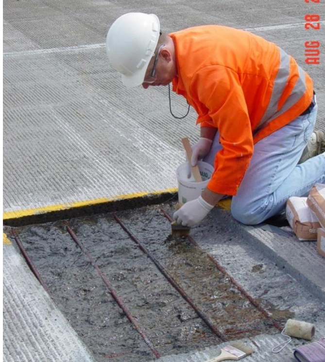
Figure 5.57 Priming a Patch with Polymer
