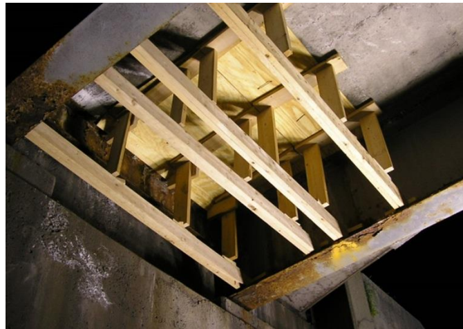
Figure 5.50 Forming for Deck Repair
