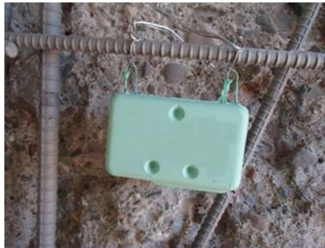
Figure 5.46 Sacrificial Anode Secured to Rebar
