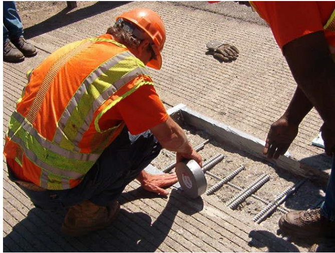
Figure 5.59 Taping the Perimeter for a Clean Look
