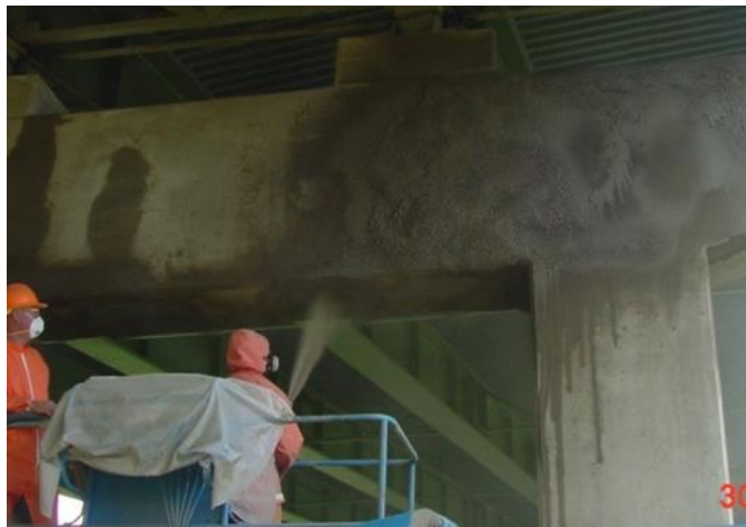
Figure 5.63 Shotcrete Repair of a Pier
