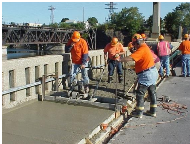
Figure 5.67 Use of a Screed to Finish Elevation on a Sidewalk
