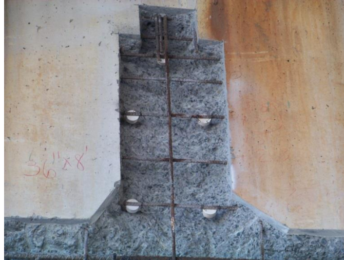
Figure 5.53 Galvanic Anodes Placed into a Patch of a Pier Cap
