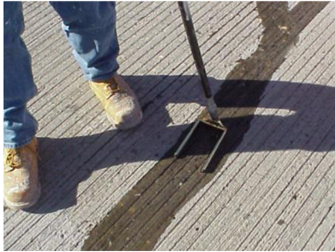
Figure 5.73 Modified Squeegee to Contain Low Viscosity Polymer
