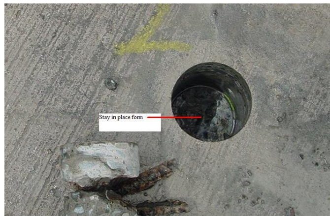
Figure 5.29 Example of Core Removal
