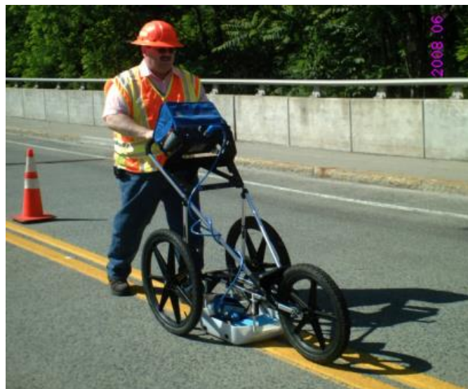
Figure 5.25 Worker Performing GPR Testing
