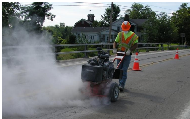
Figure 5.75 Routing Longitudinal Cracks
