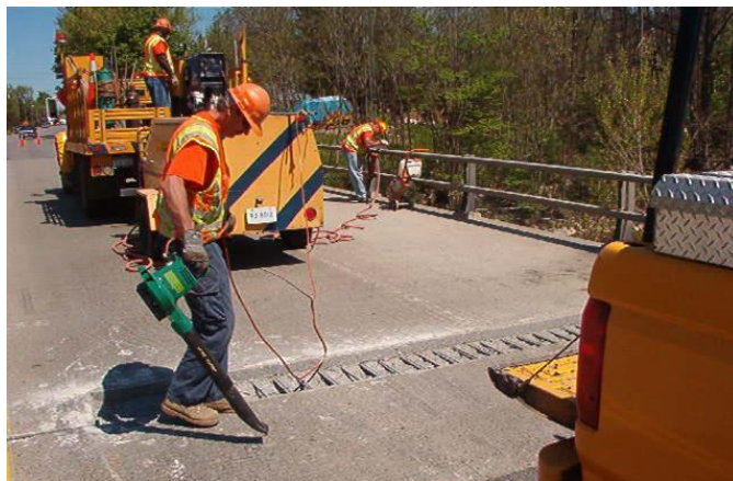
Figure 5.58 Using a Leaf Blower to Clean Surfaces
