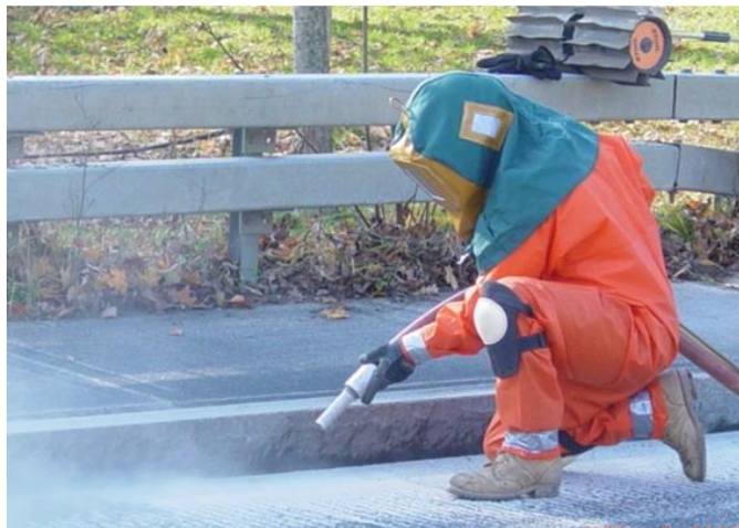
Figure 5.36 Abrasive Blast Cleaning Along the Curb Line
