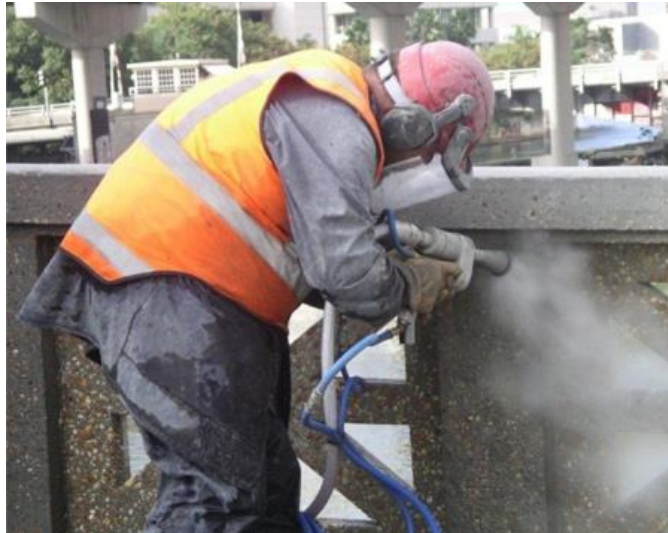
Figure 5.37 Abrasive Blast Cleaning a Concrete Barrier
