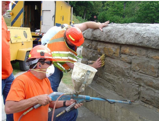
Figure 5.66 Re-Pointing a Laid-Up Stone Parapet With a Small Volume Shotcrete Tool
