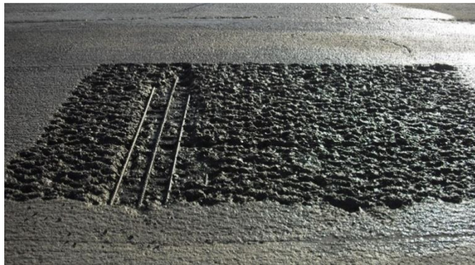
Figure 5.44 Hydrodemolition Test Section
