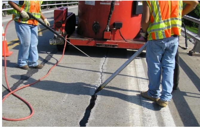
Figure 5.76 Placing Crack Sealing into "Working Cracks"
