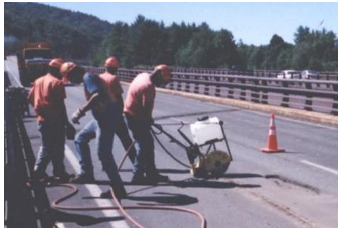
Figure 5.40 Saw cut and Removal of Deck Cover Concrete
