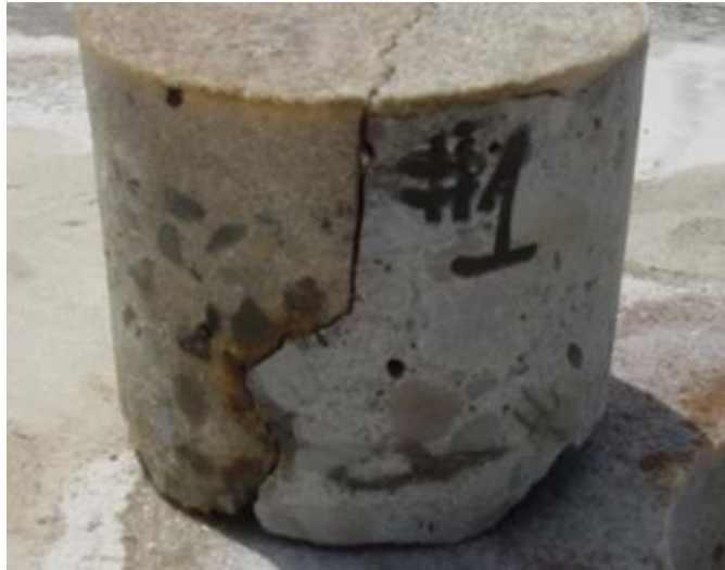
Figure 5.30 Core of Repaired Concrete at Perimeter of Patch
