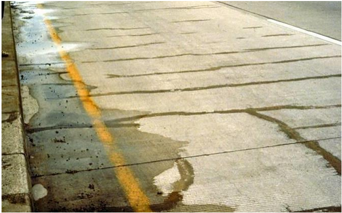
Figure 5.7 Plastic Shrinkage
