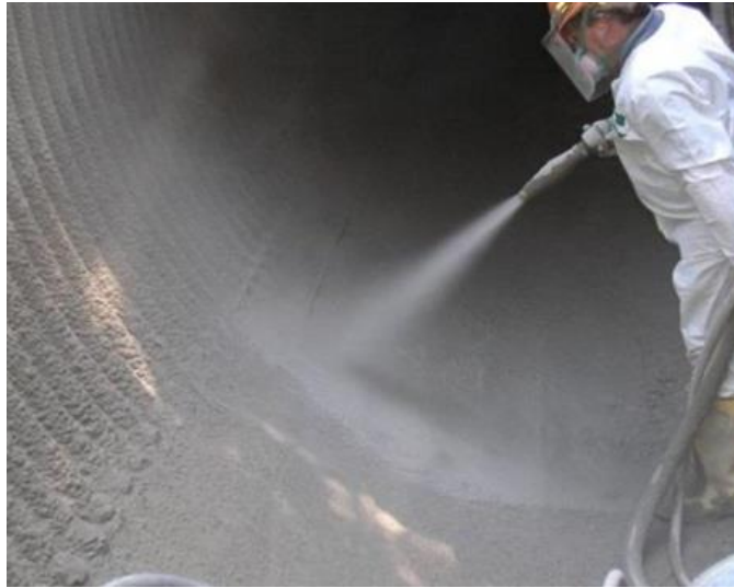
Figure 5.62 Shotcrete Repair of an Invert of a Corrugated Metal Culvert
