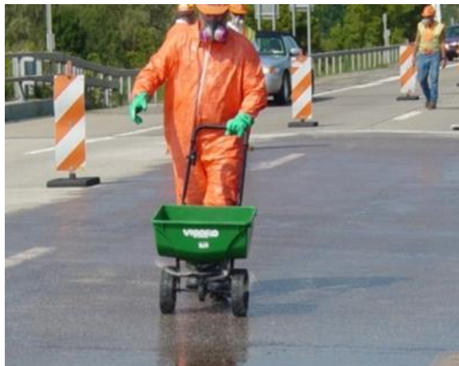
Figure 5.77 Spreading Mortar Sand onto Topical Crack Sealer
