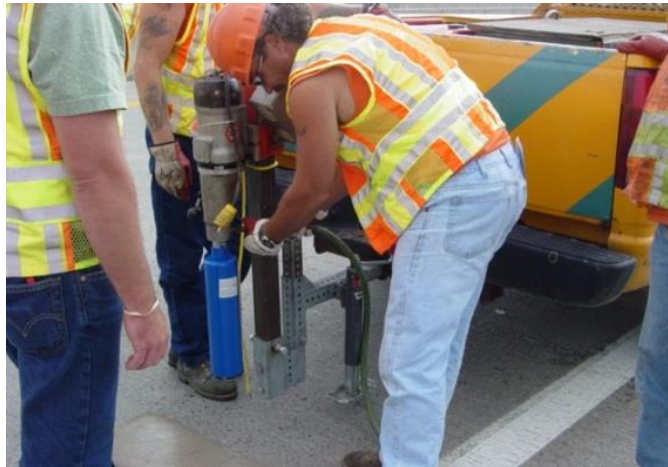
Figure 5.31 Coring Rig Anchored to Trailer Hitch
