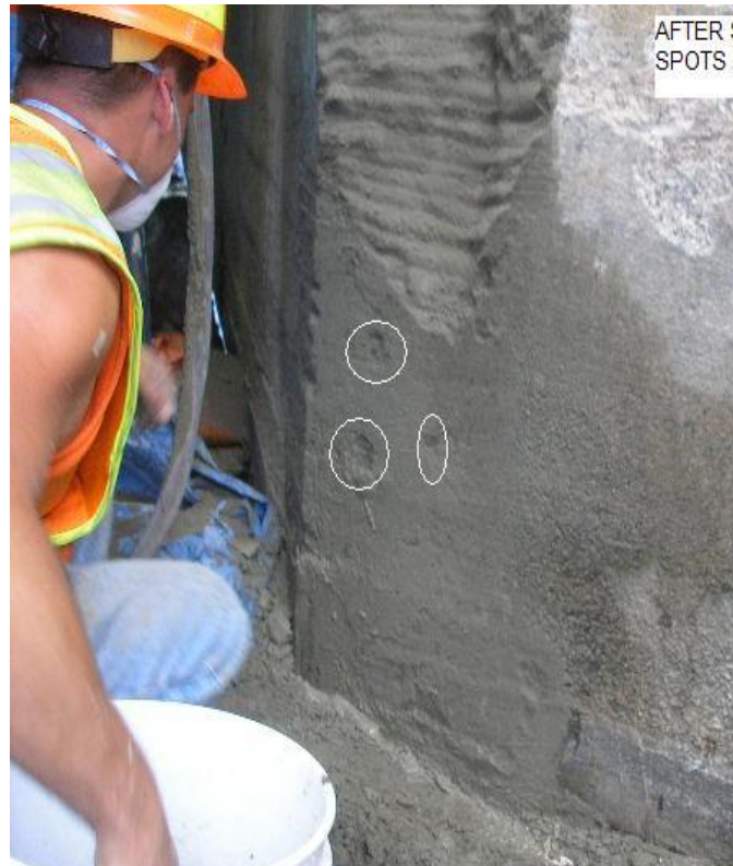
Figure 5.64 Repair "Bug-Holes" after Placing Shotcrete
