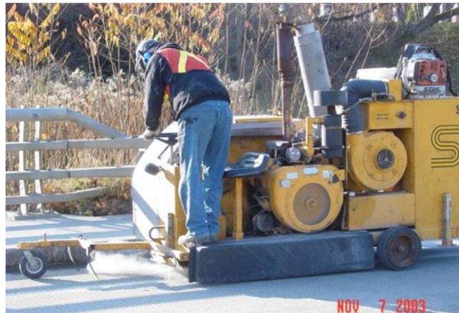
Figure 5.38 Shotblasting a Bridge Deck
