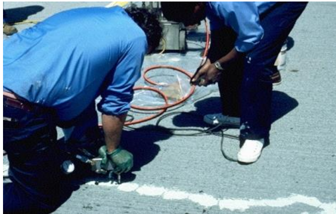
Figure 5.78 Epoxy Injection Repair (Horizontal Surface)
