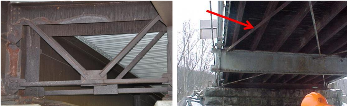
Figure 4.18 Secondary Structural Member Examples in a Superstructure
