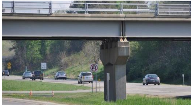
Figure 4.23 Structurally Non-redundant Multiple Span Bridge
