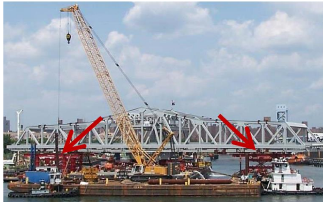
Figure 4.19 Pre-Fabricated Steel Truss on Barges
