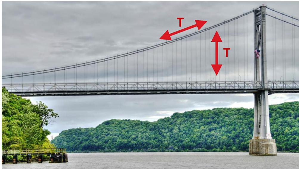
Figure 4.3 Axial Tension in a Suspension Bridge
