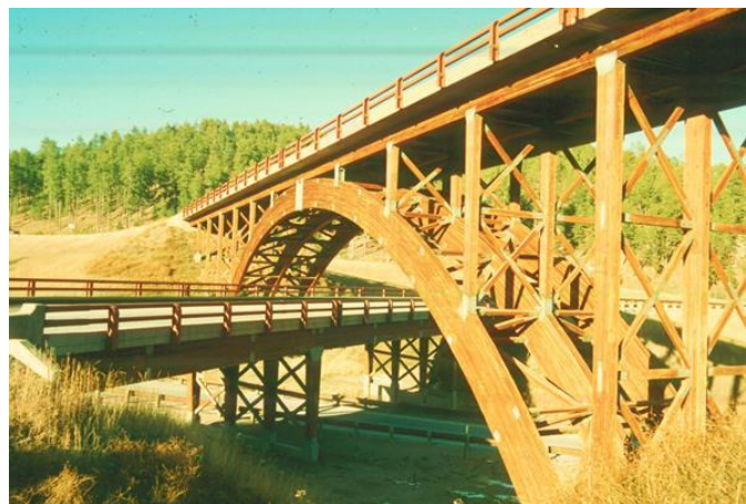
Figure 3.58 Glulam Deck Arch Bridge
