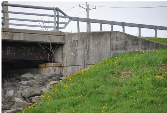
Figure 3.36 Example of a Wingwall
