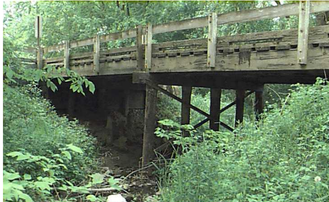
Figure 3.49 Timber Multi-Girder Bridge
