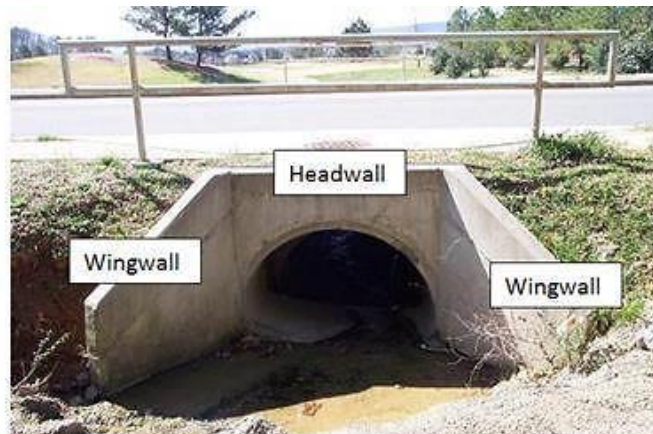
Figure 3.60 Reinforced Concrete Culvert Headwall and Wingwalls
