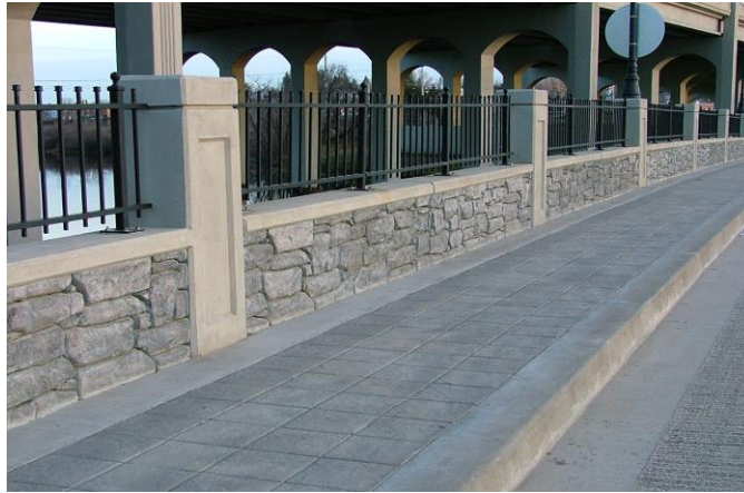
Figure 3.9 Bridge Sidewalk Using Stamped Concrete for Aesthetics and Concrete Curb
