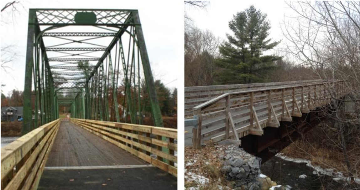
Figure 3.22 Nail-Laminated Decks. Pre-Fabricated (left) and Site-Constructed (right)
