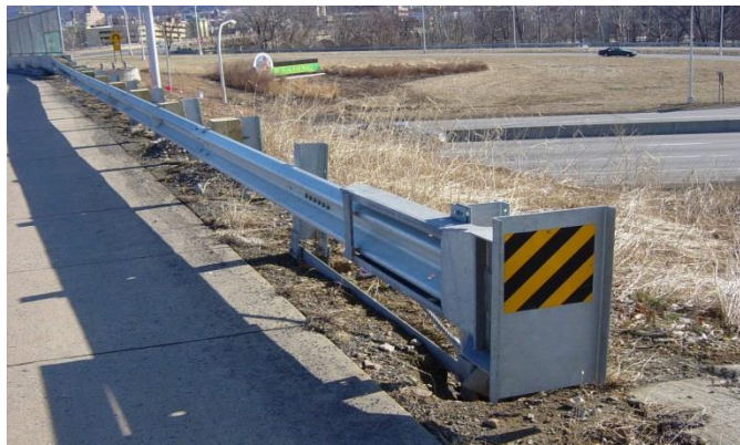
Figure 3.12 Example of an Approach Guardrail End Treatment
