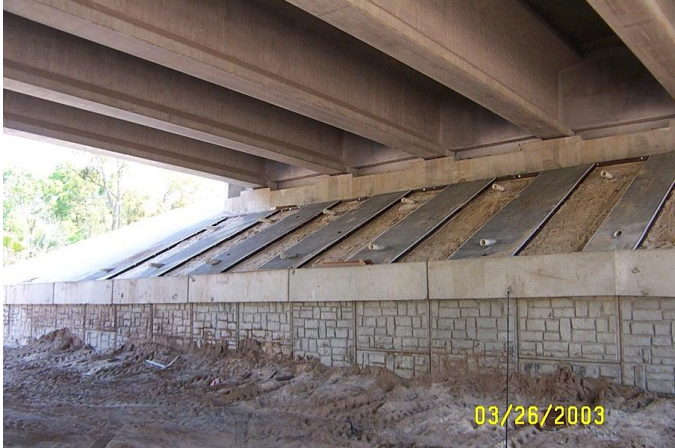
Figure 3.32 Example of a Shorter Abutment
