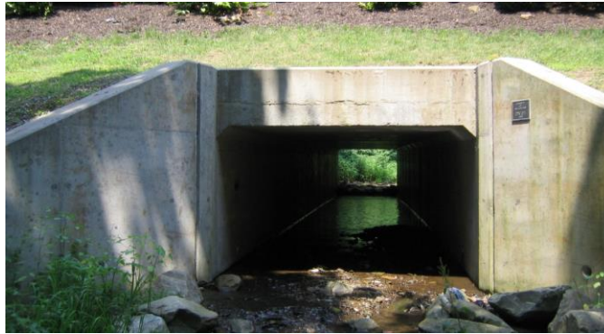
Figure 3.67 Concrete Box Culvert
