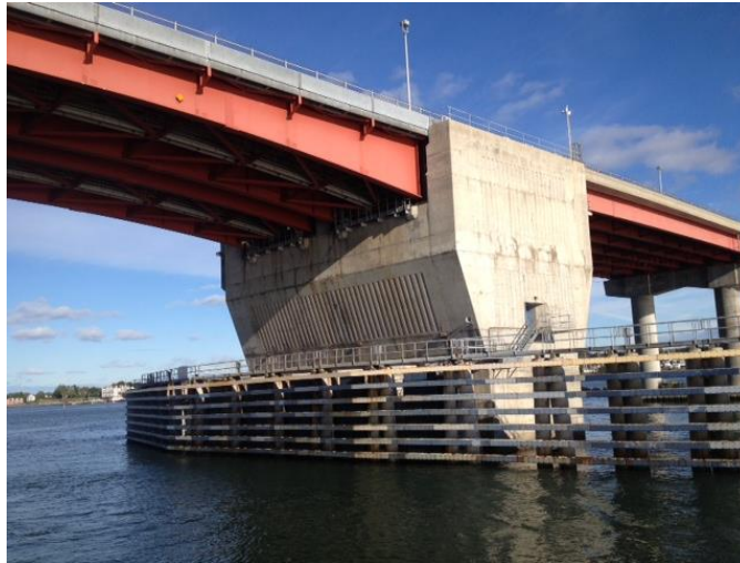
Figure 3.45 A Bridge Fender System
