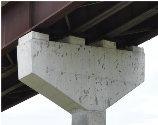
Figure 3.41 Hammerhead Pier
