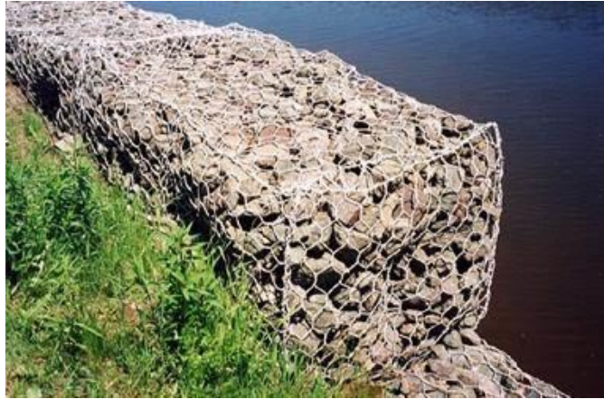
Figure 3.47 An Example of a Gabion Basket Serving as Slope Protection
