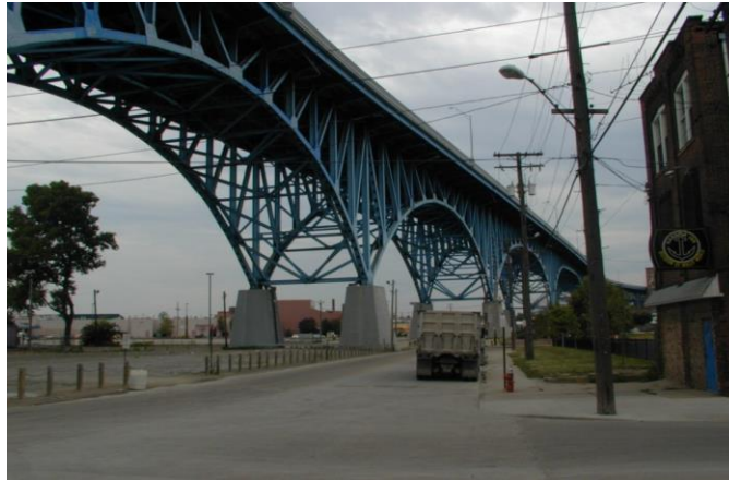
Figure 3.54 Deck Truss Bridge
