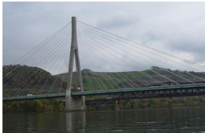
Figure 3.73 Cable-Supported Bridge: Cable Stayed
