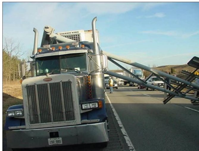
Figure 3.76 Failed Ancillary Sign Structure
