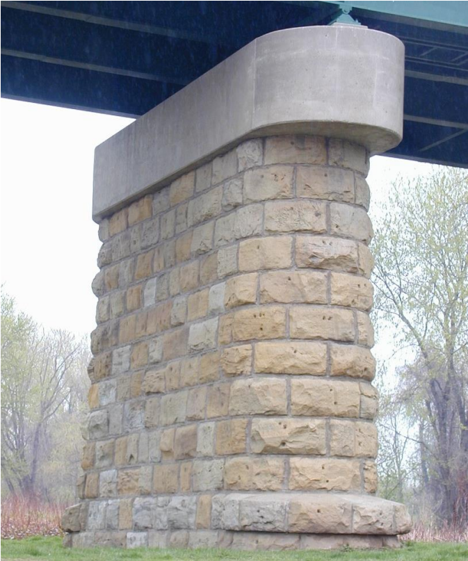
Figure 3.39 Solid Shaft Pier
