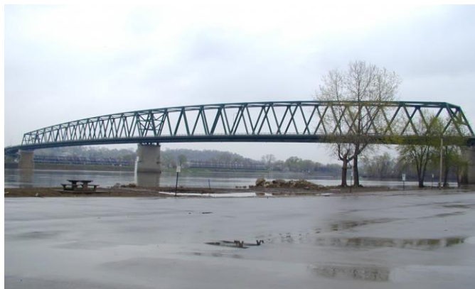
Figure 3.55 Through Truss Bridge
