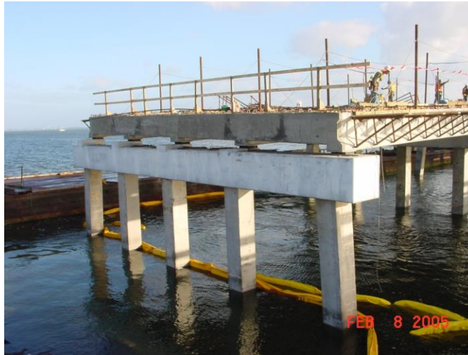
Figure 3.42 Concrete Cap as Part of Pile Bent Structure
