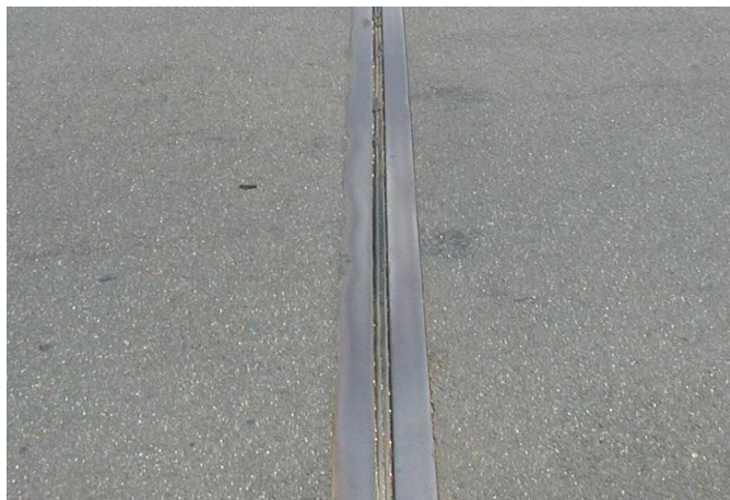
Figure 3.6 Top View of an Armored Compression Seal
