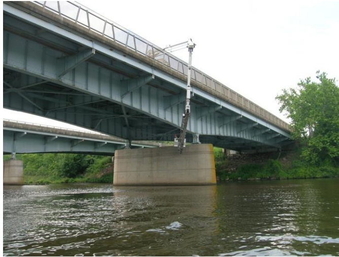
Figure 3.51 2-Girder Steel Bridge
