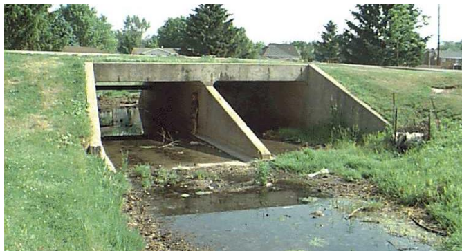
Figure 3.68 Multicell Concrete Box Culvert
