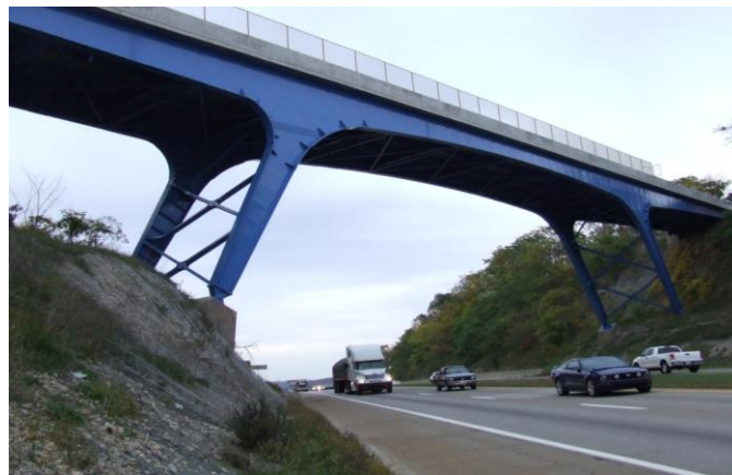
Figure 3.53 Example of a Rigid Frame Bridge
