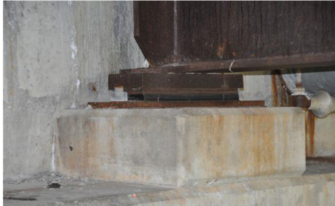
Figure 3.29 Elastomeric Bearing
