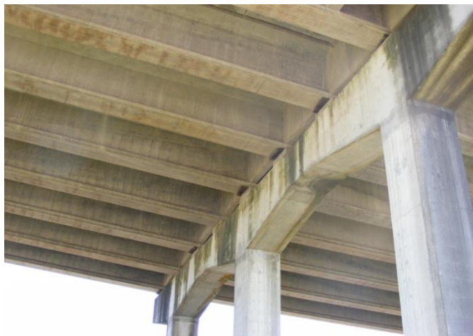
Figure 3.50 Prestressed Concrete Multi-Girder Bridge
