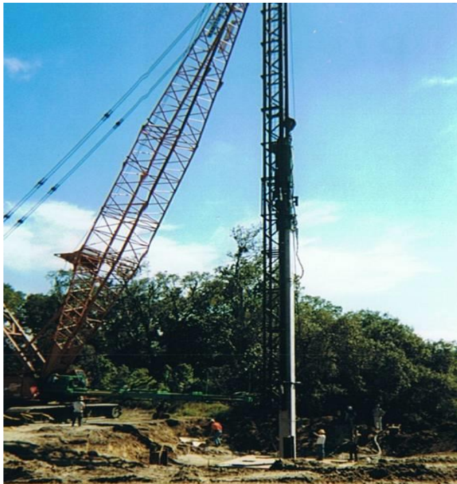
Figure 3.43 Lead-on Pile Driver
