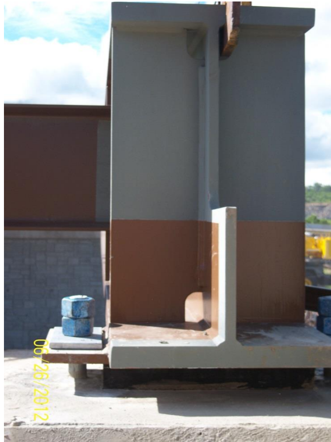
Figure 3.15 Bearing Stiffener
