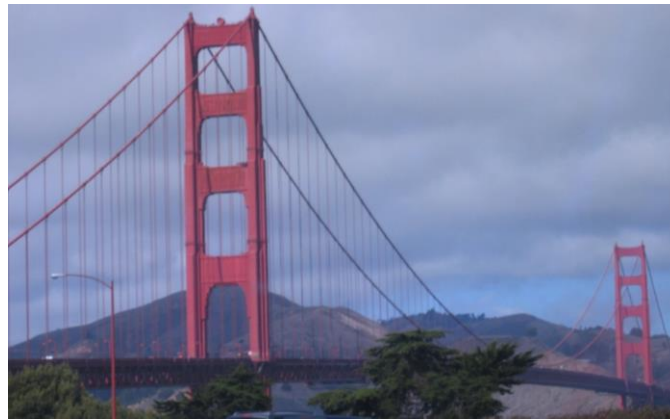
Figure 3.71 Cable-Supported Bridge: Suspension Cables and Suspenders
