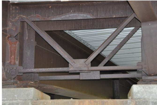
Figure 3.27 Diaphragm (K-bracing)
