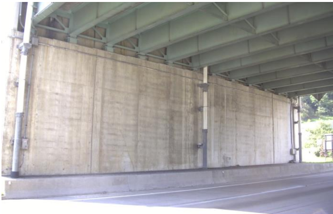
Figure 3.31 Abutment Supporting Superstructure End
