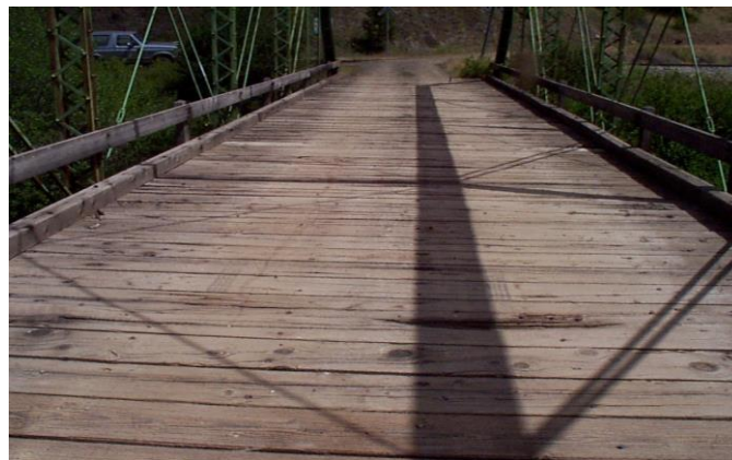
Figure 3.3 Timber Plank Deck
