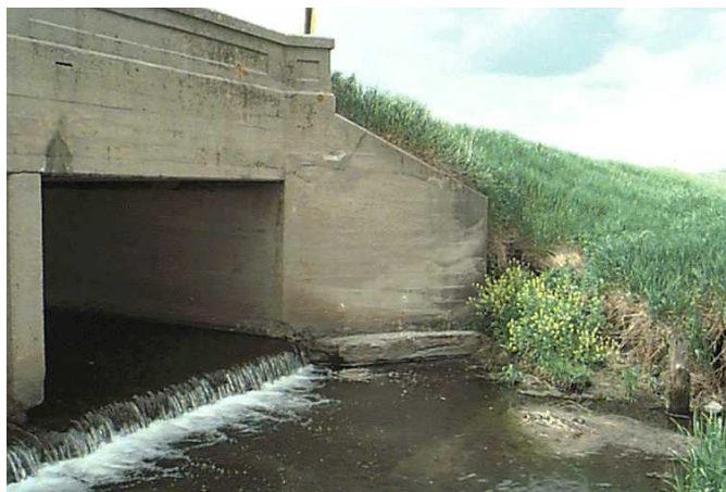
Figure 3.64 Cast-In-Place Concrete Headwall and Wingwall
