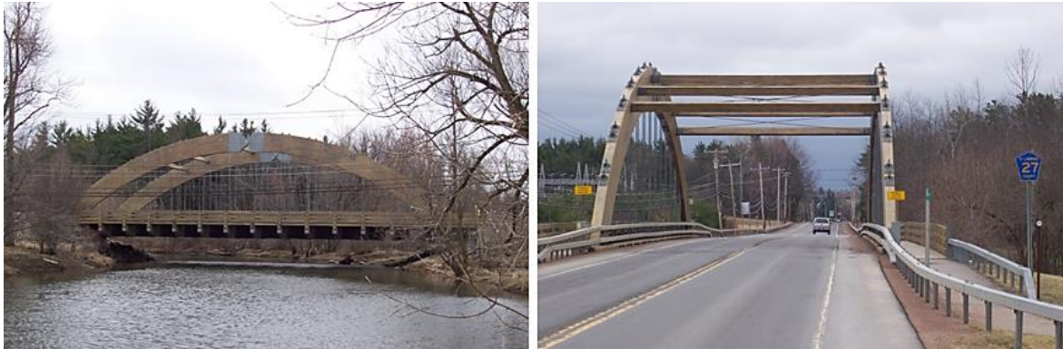
Figure 3.57 Glulam Suspension Arch Bridge
