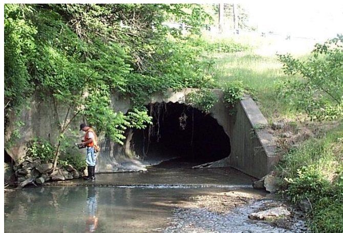
Figure 3.61 Culvert End Projection
