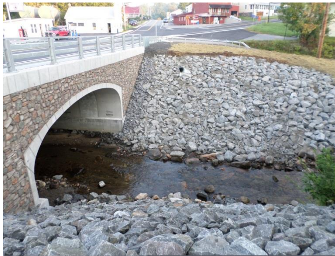
Figure 3.48 Riprap Used for Slope Protection
