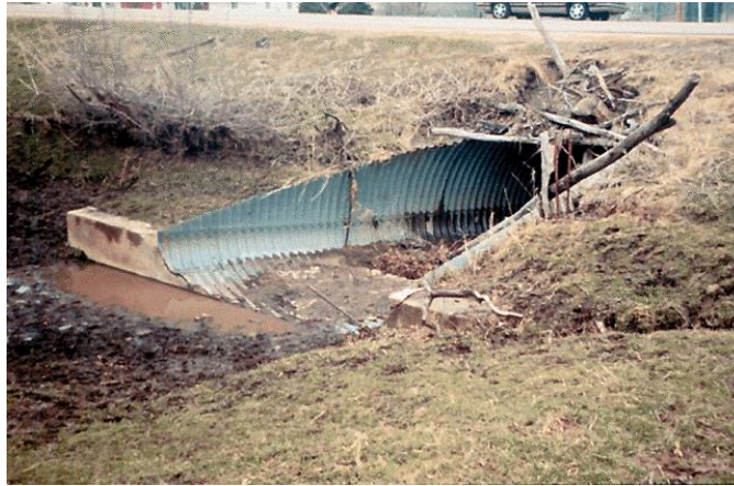
Figure 3.62 Culvert Mitered End
