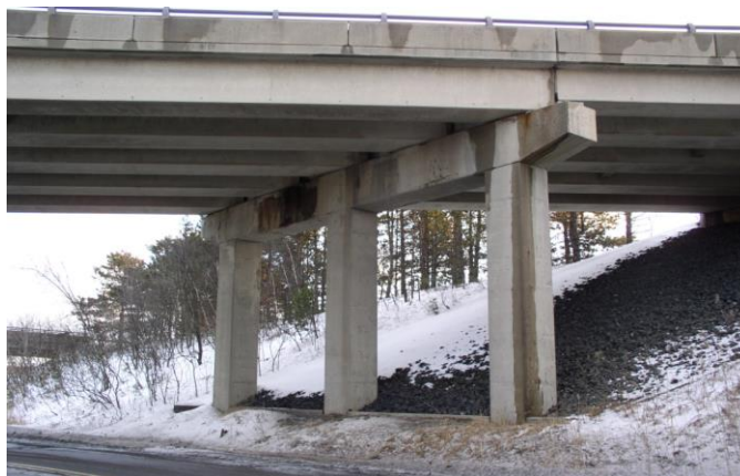
Figure 3.37 Piers Support the Superstructure
