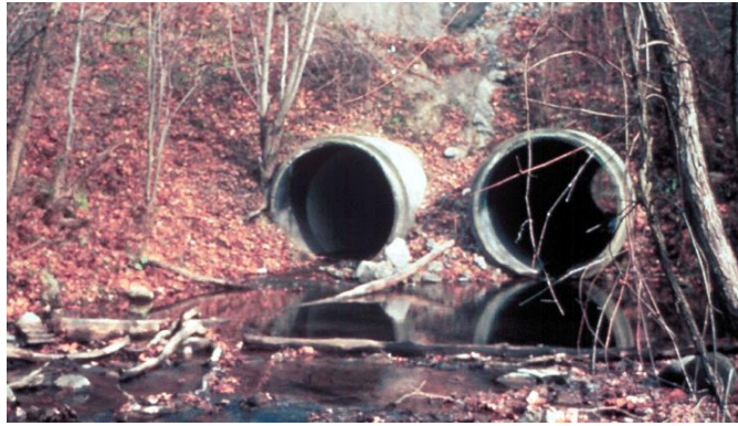
Figure 3.69 Twin Concrete Pipe Culvert
