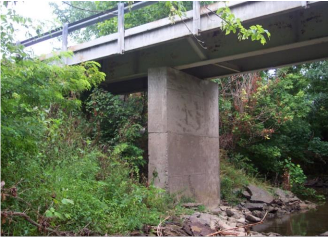
Figure 3.38 Solid Shaft Pier
