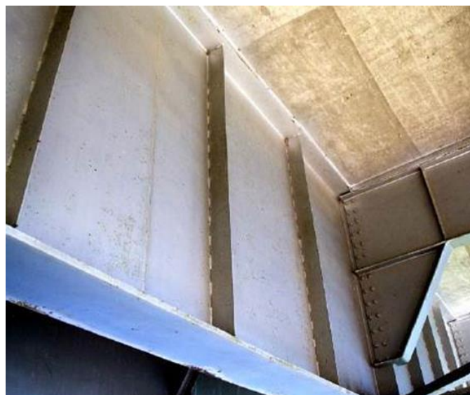
Figure 3.16 Intermediate Stiffeners
