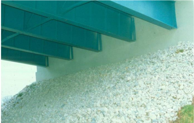
Figure 3.33 Example of an Integral Abutment
