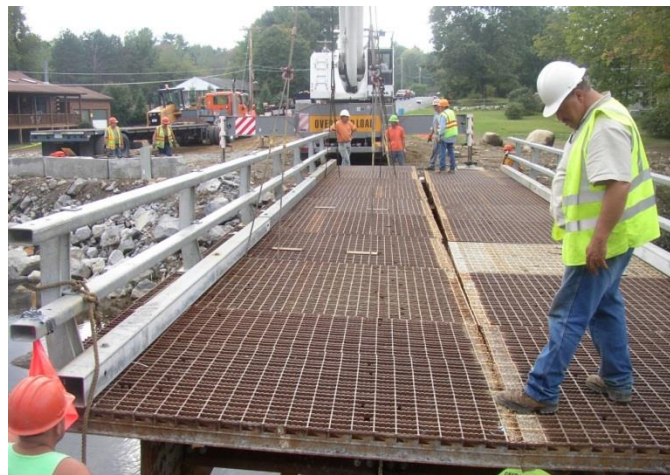
Figure 21.6 Steel Girder Temporary Bridge with Steel Deck and Steel Bridge Rail
