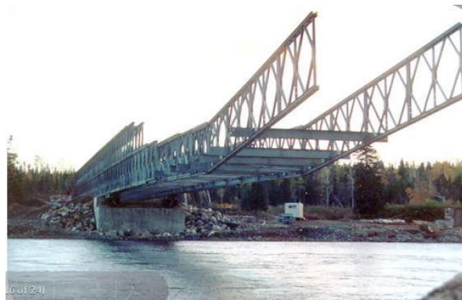
Figure 21.3 Installation of Panelized Truss with Launching Nose
