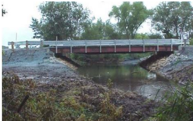
Figure 21.8 Single Span Rail Car Bridge
