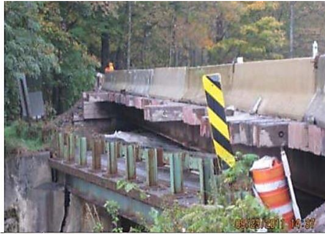
Figure 21.5 Steel Girder Temporary Bridge
