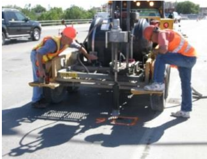
Figure 20.6 Concrete Deck Coring Equipment
