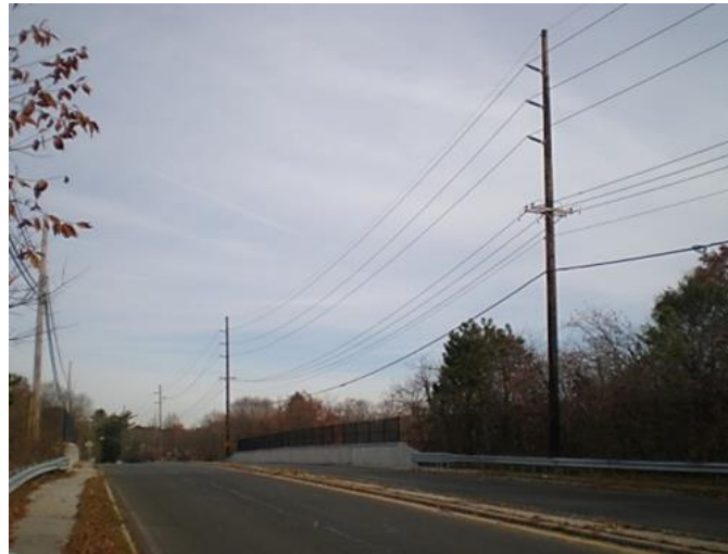
Figure 19.5 Example of Overhead Lines Near Bridge Structures
