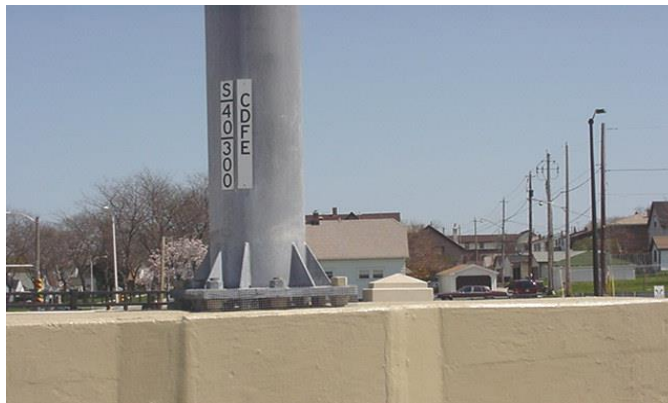
Figure 19.19 Example of Sign Structure Identification
