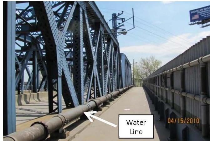
Figure 19.4 Water Line Crossing Mounted to Bridge
