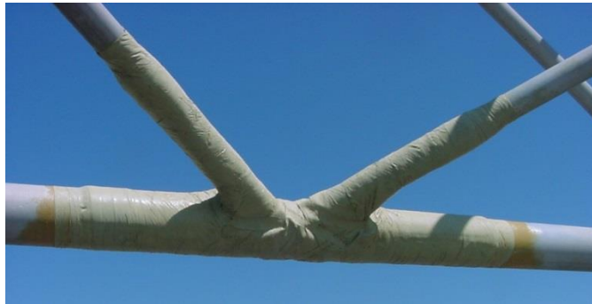
Figure 19.31 FRP Repair of Cracked Secondary Truss Connection
