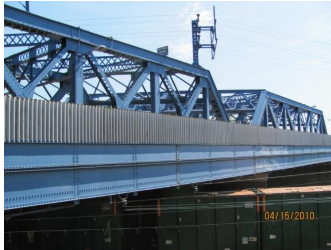
Figure 19.2 Visible Electric Lines Above and Under a Bridge Structure
