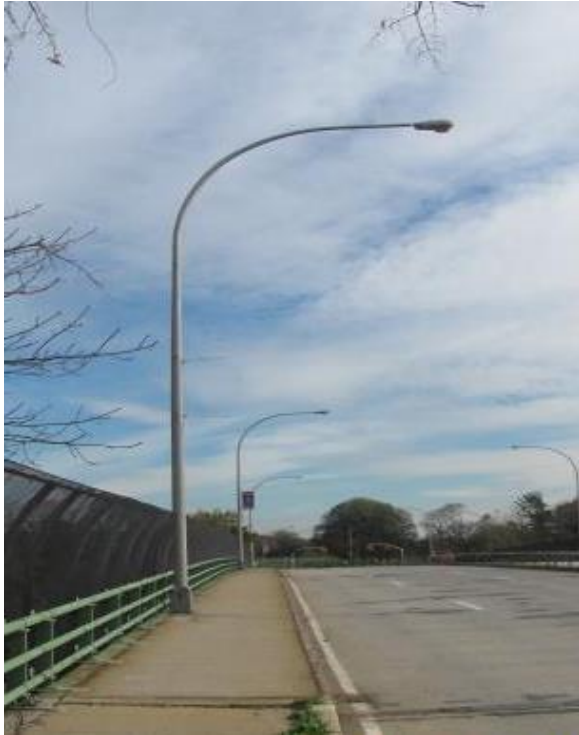
Figure 19.7 Example of Street Lighting Attached to Bridge Structure
