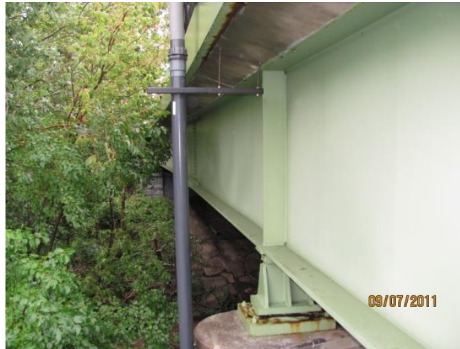
Figure 19.26 Example of Adhesive Anchors Subjected to Continuous Tension Loading
