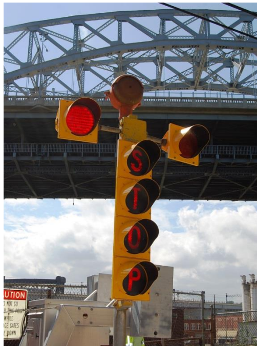
Figure 17.61 Warning Lights and Gong
