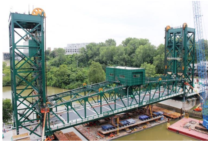
Figure 17.8 Span Driven Vertical Lift Bridge
