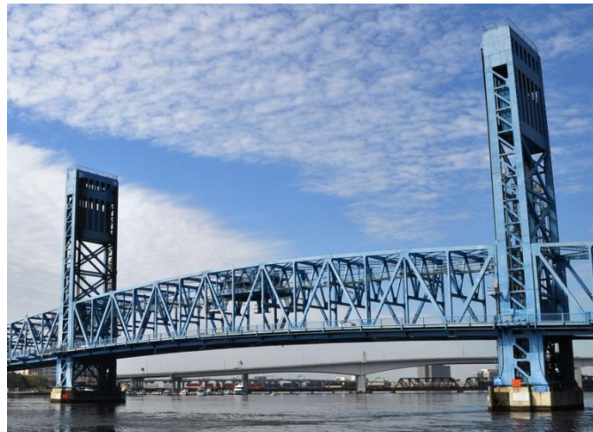
Figure 17.9 Tower Driven Vertical Lift Bridge
