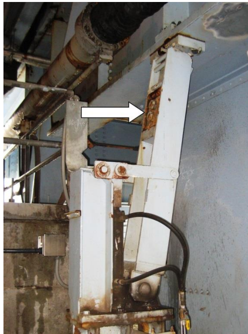
Figure 17.29 Engaged Tail Lock
