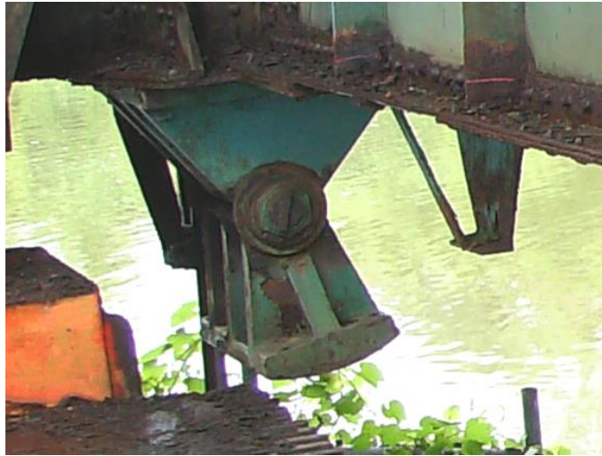
Figure 17.84 Frozen Expansion Live Load Support
