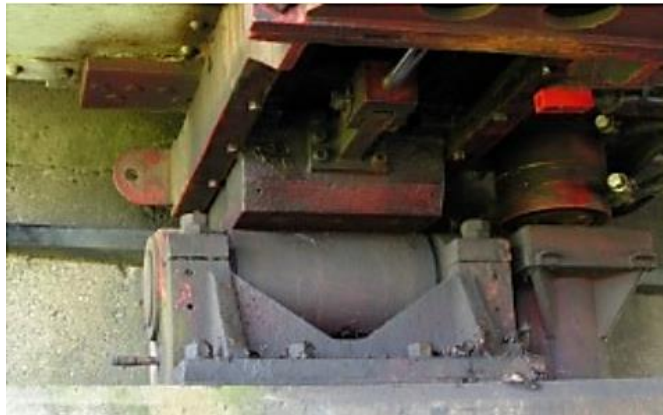
Figure 17.76 Heavy-Duty Roller Bearing on Bascule Bridge
