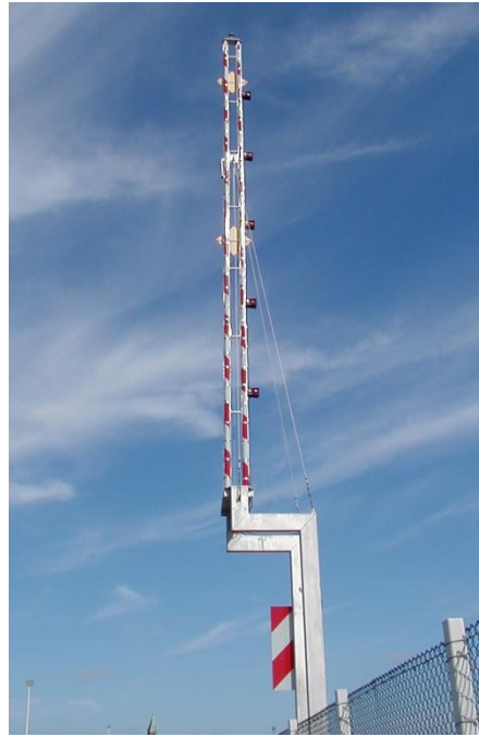
Figure 17.62 Resistance Gate (Courtesy of MaineDOT)
