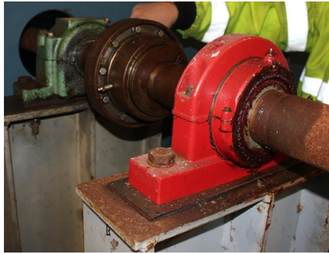
Figure 17.22 Bearings Supporting Span Drive Shaft
