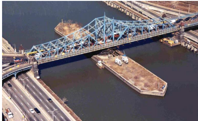
Figure 17.11 Center Bearing Swing Span Bridge
