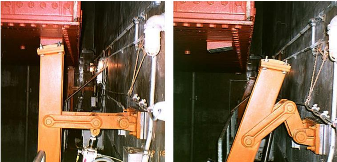
Figure 17.30 Tail Lock in Fully Engaged Position (left) and Disengaged Position (right) (Courtesy of MaineDOT)
