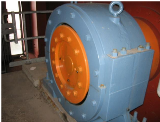
Figure 17.78 Example of a Trunnion Bearing (Courtesy of MaineDOT)
