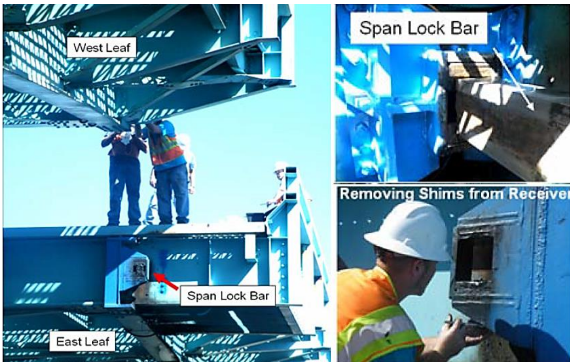
Figure 17.27 Span Lock Bars and Shim Removal (Courtesy of FDOT)
