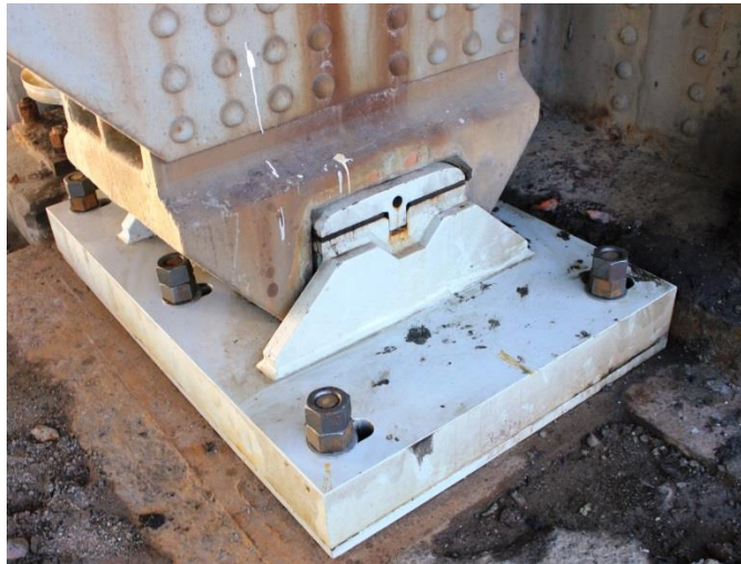
Figure 17.32 Fixed Live Load Bearing
