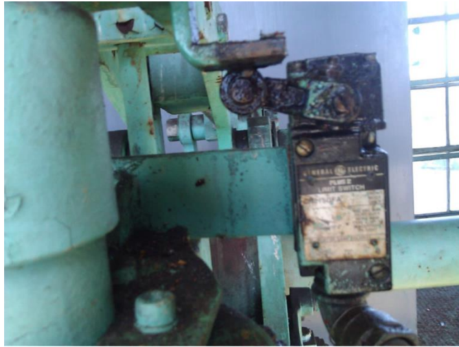
Figure 17.69 Limit Switch Indicates Machine Brake Position (Courtesy of NHDOT)
