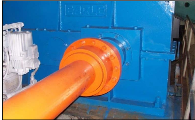
Figure 17.46 Closed Gear (Speed Reducer)
