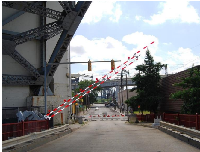
Figure 17.60 Traffic Barrier and Warning Gates
