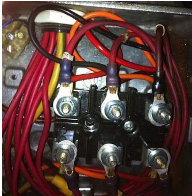
Figure 17.92 Ring-Tongue Terminal Assembly
