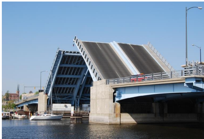
Figure 17.1 Bicentennial Bascule Bridge over the St. Joseph River
