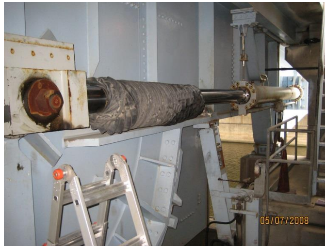
Figure 17.6 Hydraulic Cylinder on Trunnion Bascule Bridge
