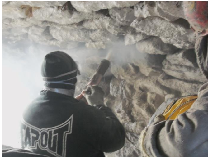
Figure 16.29 Pressure Injection of Mortar (Note presence of paraffin wax on stones)
