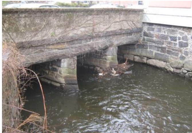
Figure 16.6 Granite Slab Bridge
