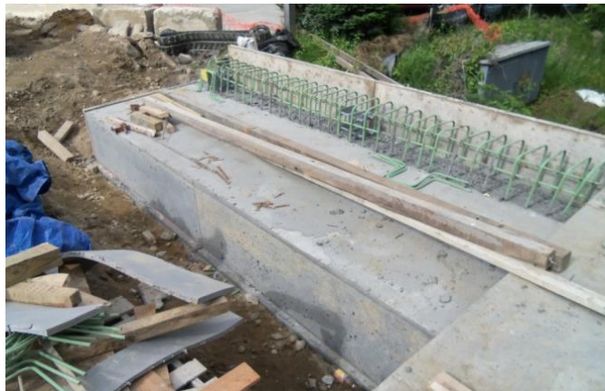
Figure 16.34 Reinforced Concrete Moment Slab (Under Construction)
