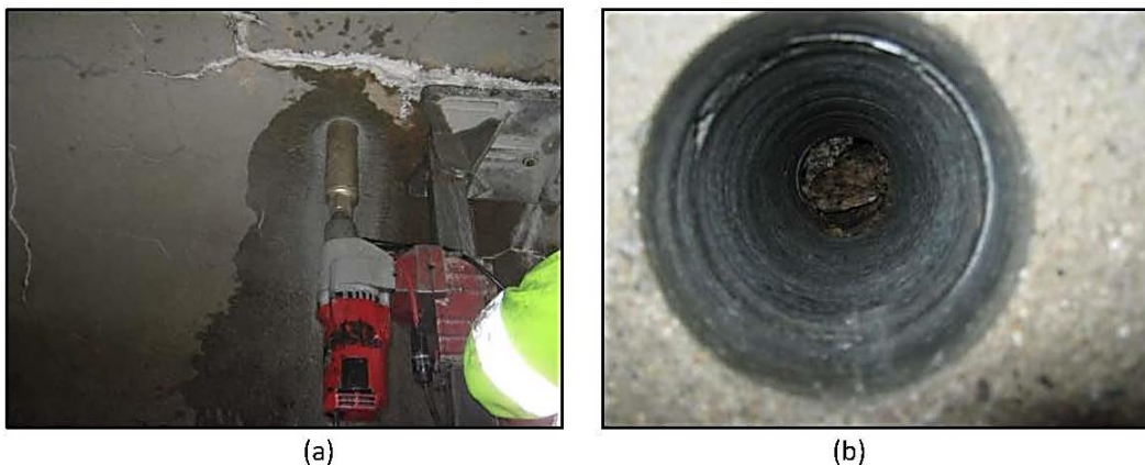
Figure 16.21 Masonry Cores (a) Removing the Core and (b) Finished Masonry Core
