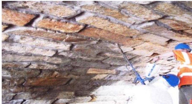
Figure 16.30 Pressure Injection of Mortar (Smaller nozzle size for neater application)
