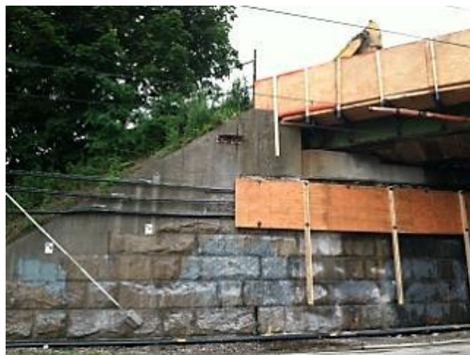
Figure 16.7 Masonry Substructure
