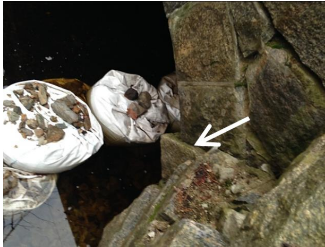
Figure 16.13 Mortar Deterioration (indicated by arrow)
