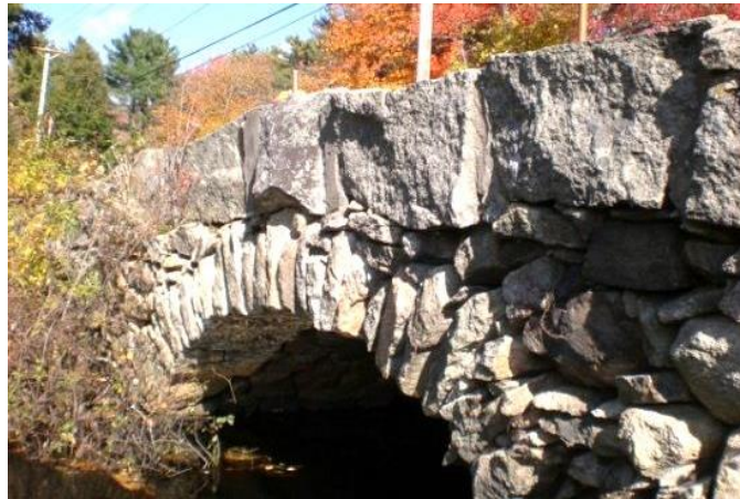
Figure 16.24 Vegetation Growing Through Masonry Joints
