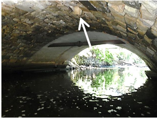
Figure 16.16 Single Slipped Stone
