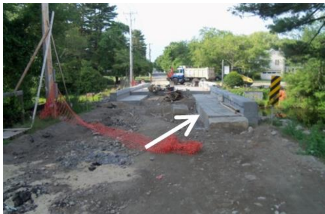
Figure 16.35 Moment Slab (indicated by arrow)
