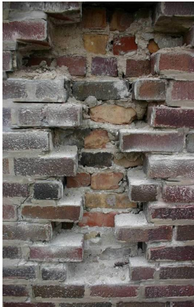
Figure 16.20 Inspection Opening
