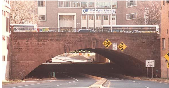
Figure 16.8 Brick Arch and Spandrel Walls
