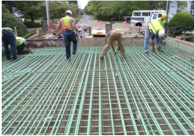
Figure 16.33 Reinforced Concrete Relieving Slab (Under Construction)
