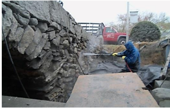
Figure 16.25 Cleaning with Low Pressure Water
