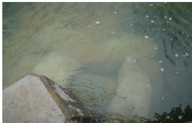
Figure 15.25 Grout Bags Installed around a Pier Nose (Courtesy Virginia DOT)
