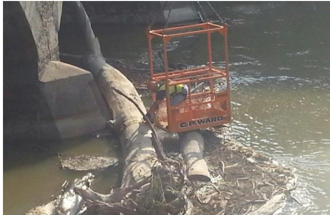
Figure 15.7 Debris Removal Operation (Courtesy of the City of Rochester, New York - Department of Environmental Services)
