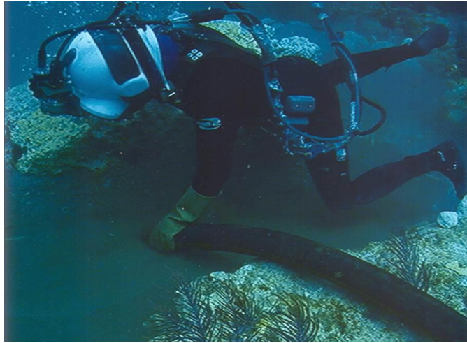
Figure 15.22 Tremie Placement (Courtesy of Underwater Engineering Services, Inc.)
