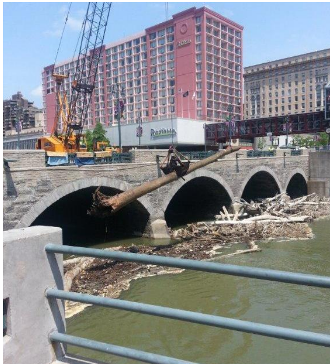
Figure 15.8 Debris Removal Operation (Courtesy of the City of Rochester, New York - Department of Environmental Services)
