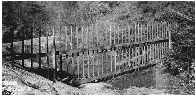
Figure 15.9 Post and Rail Debris Rack Installed 100 Feet Upstream of Culvert
