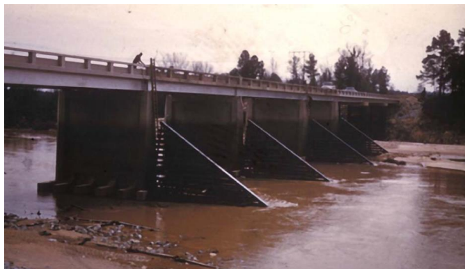
Figure 15.10 Timber Debris Fins with Sloping Leading Edge
