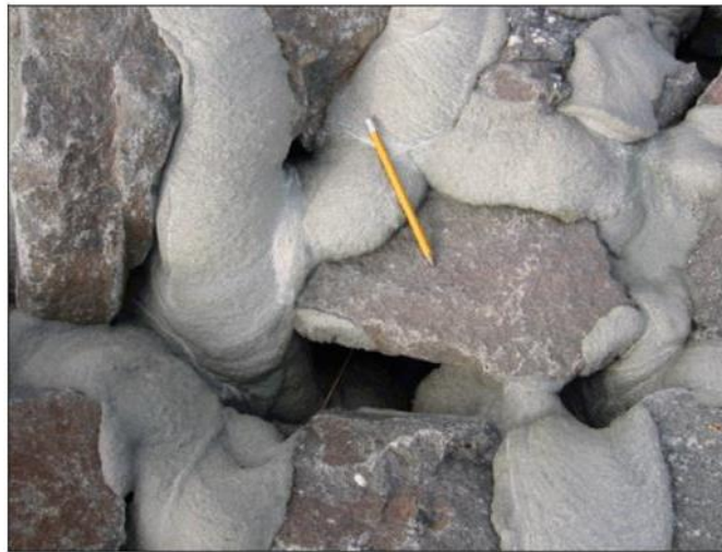
Figure 15.21 Close-Up View of Partially Grouted Riprap
