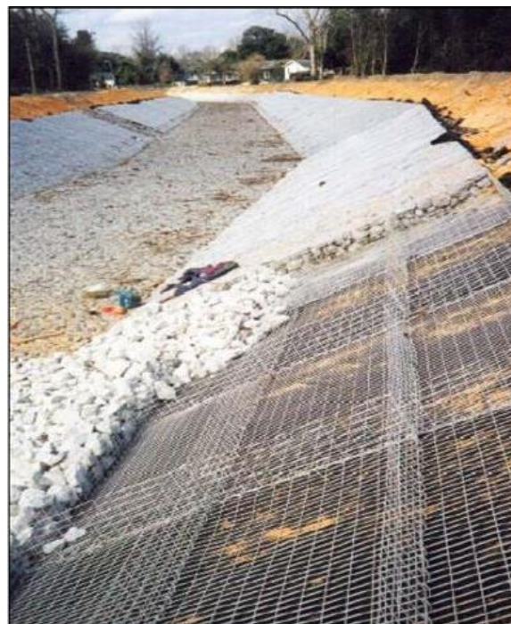
Figure 15.19 Field Installation of Gabion Mattresses on Channel Bed and Banks
