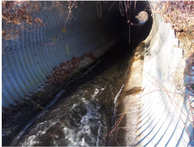
Figure 14.15 Concrete Paved Invert
