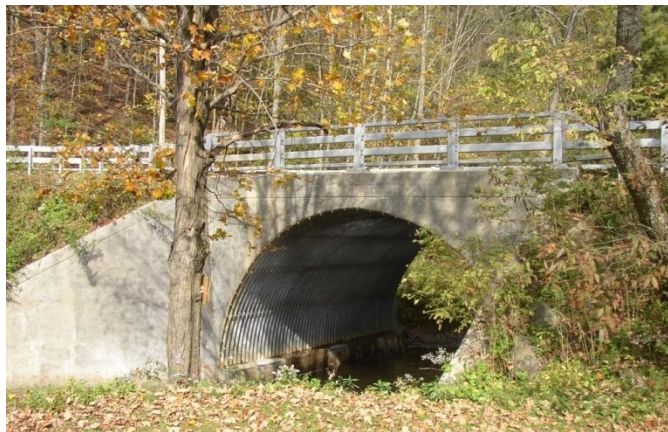
Figure 14.5 Bottomless Corrugated Metal Arch Culvert
