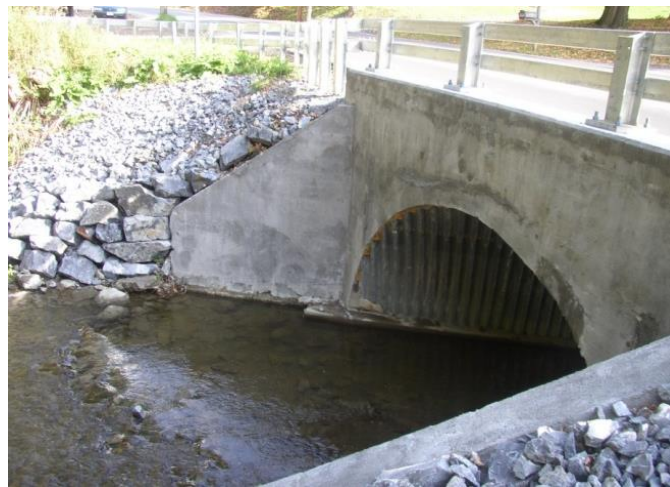
Figure 14.18 Completed Lined Arch (Courtesy of Washington County NY DPW)
