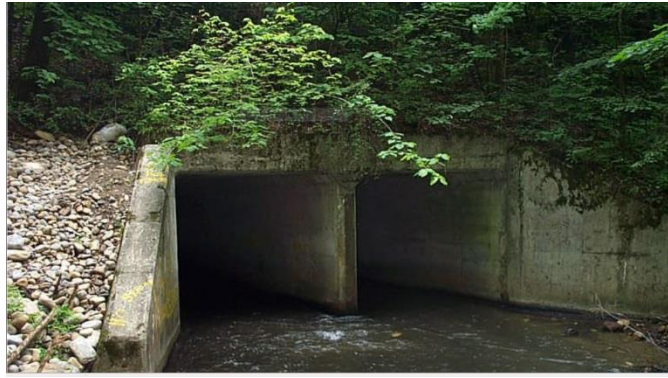
Figure 14.2 Twin Barrel Cast-in-Place Concrete Box Culvert
