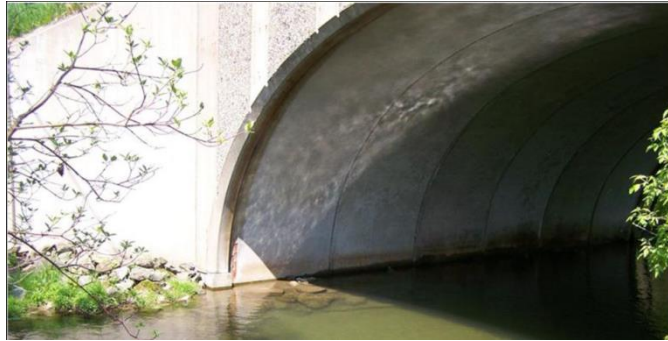
Figure 14.4 Bottomless Precast Concrete Arch
