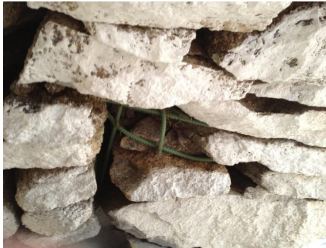
Figure 14.26 Reinforcing Steel Installed Prior to Grouting Stone Masonry
