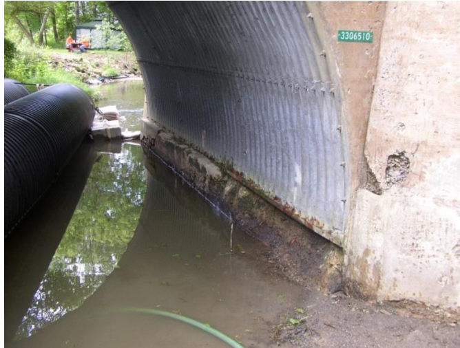
Figure 14.27 Preparation for Footing Repair on Corrugated Plate Arch
