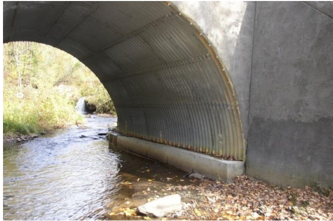
Figure 14.28 Repaired Footing for Corrugated Plate Arch
