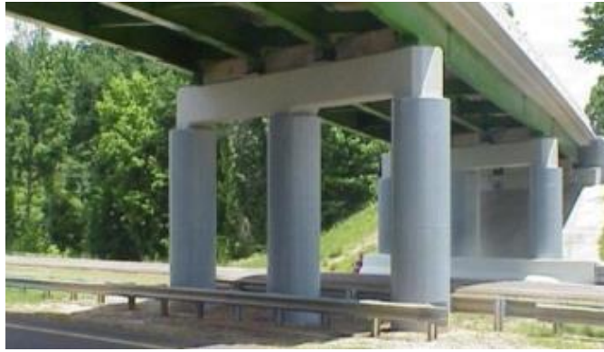
Figure 13.88 Fiber Reinforced Polymer Column Confinement Shells
