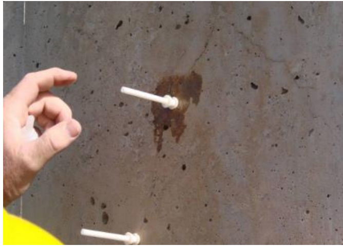
Figure 13.33 Installation of Epoxy Injection Ports (Courtesy of MDOT)
