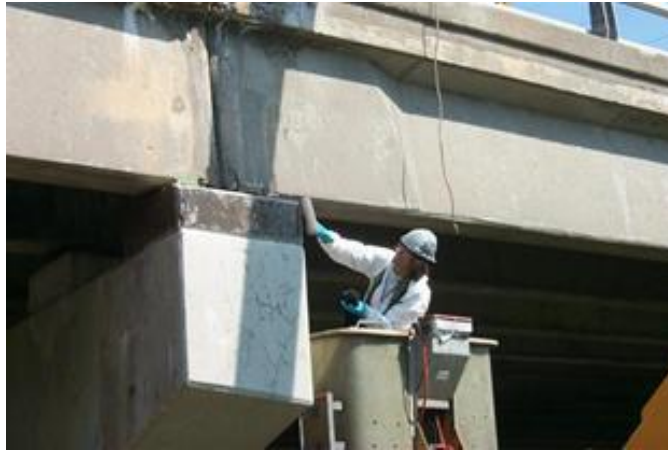
Figure 13.50 Pedestal Repair with FRP
