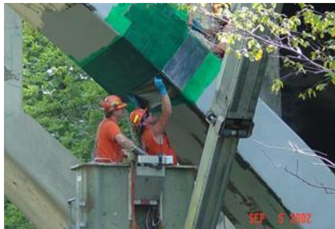
Figure 13.49 Strengthening a Spandrel Arch with FRP
