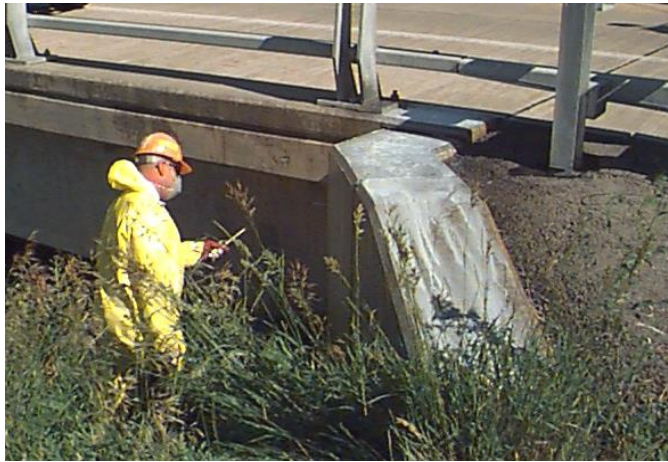
Figure 13.7 Hand Sealing the Substructure
