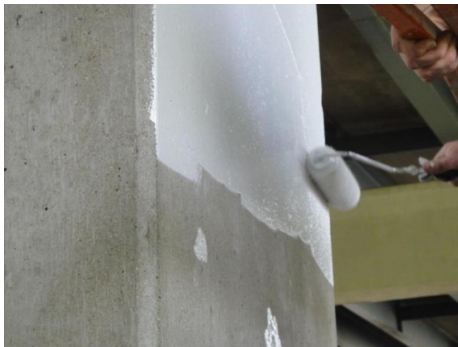
Figure 13.8 Protective Coating Applied on the Substructure
