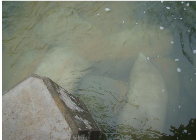
Figure 13.40 Grout Bags Used to Prevent Undermining
