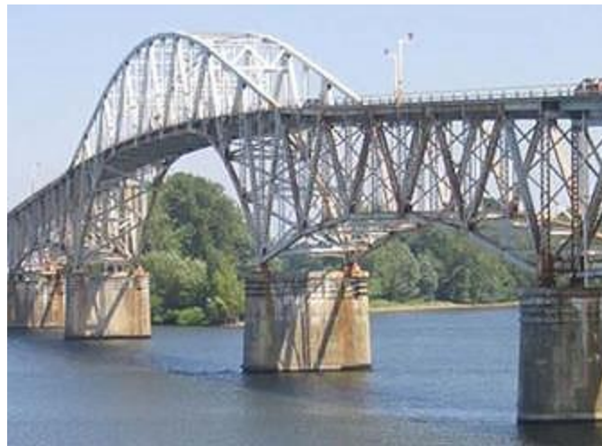
Figure 13.52 External Post-Tensioning Rods used in Pier Containment
