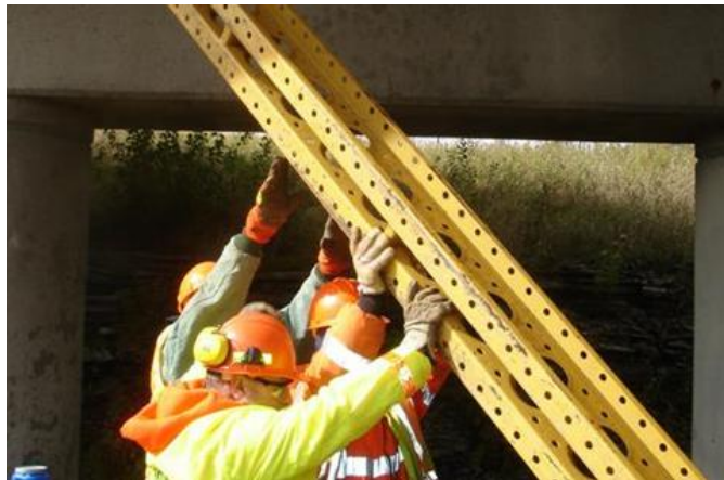
Figure 13.81 Lifting a Support Column
