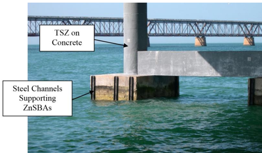
Figure 13.13 Thermally Sprayed Zinc Applied to a Pier Column
