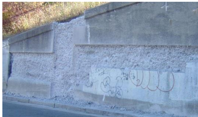
Figure 13.24 Preparation for Repair of Retaining Wall
