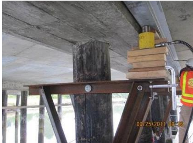
Figure 13.67 Timber Cap Replacement (Courtesy of Virginia DOT)
