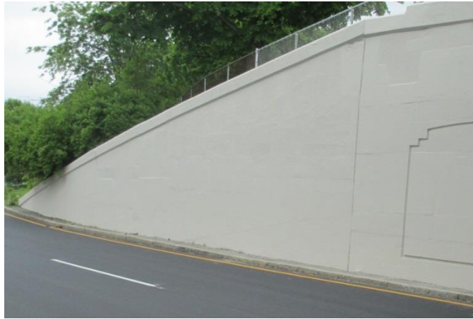
Figure 13.25 Retaining Wall After Repairs
