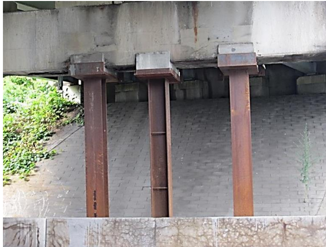
Figure 13.84 Temporary Steel Shoring used to Support Deteriorated Concrete Pier Cap
