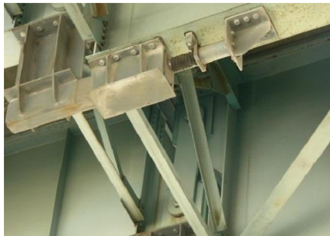
Figure 13.90 Viscous Dampers (Courtesy of California Department of Transportation)
