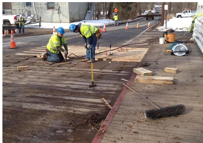
Figure 13.20 Timber Bridge Deck Being Replaced
