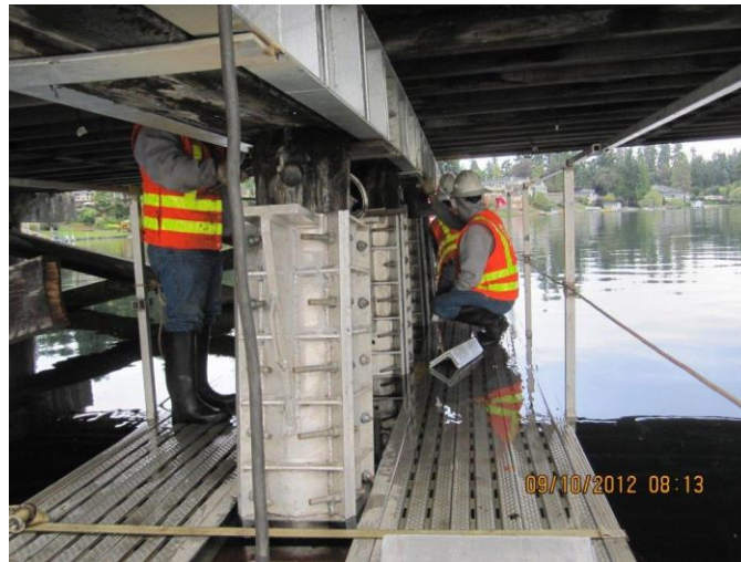
Figure 13.70 Use of Jack Stands to Ensure Adequate Load Transfer for Pile Splices (Courtesy of Washington DOT)
