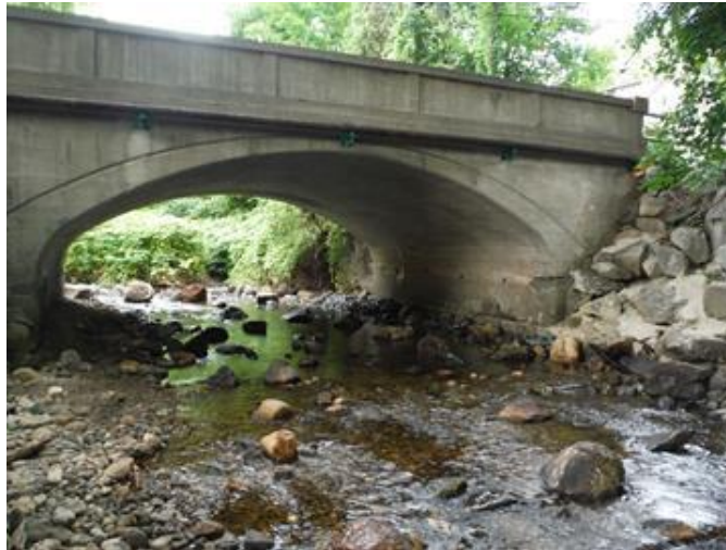
Figure 13.39 Final Condition with Streambed Restored
