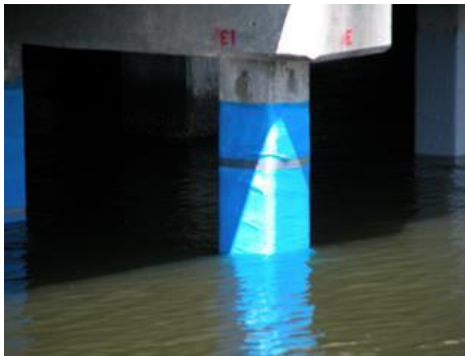
Figure 13.51 Completed Column Repair with FRP
