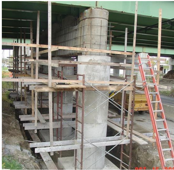
Figure 13.23 Non-Structural Repair of a Column
