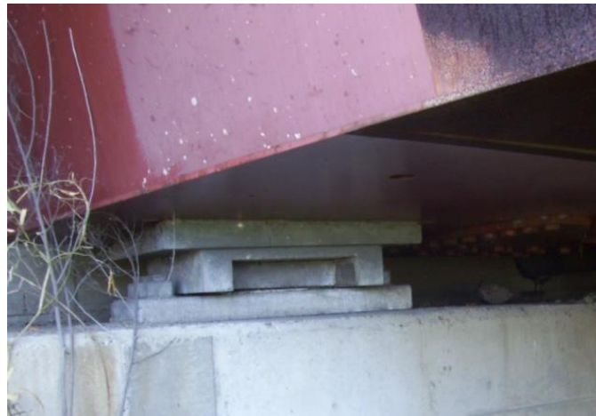
Figure 12.9 Example of a Pot Bearing
