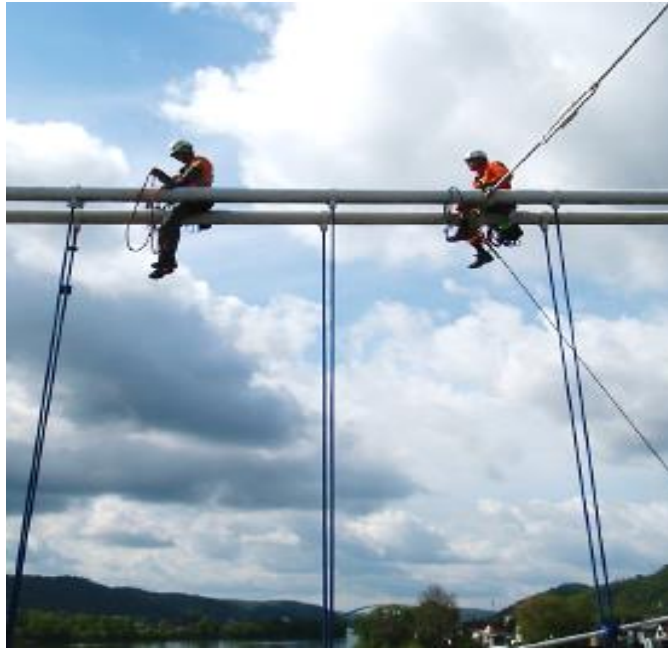
Figure 12.30 Main Cable Inspection
