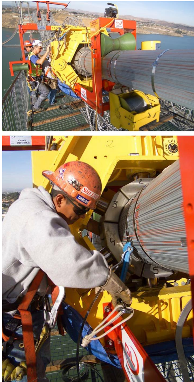
Figure 12.34 Cable Compaction Photos (Courtesy of Caltrans)
