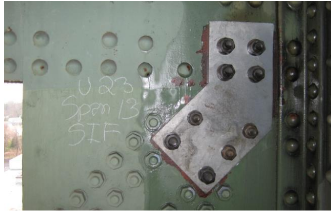
Figure 12.20 Gusset Plate Repair by Installation of Reinforcement Plate
