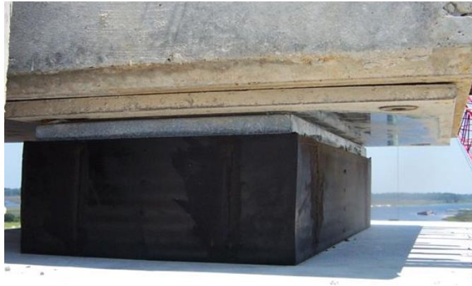
Figure 12.6 Photo of a Reinforced Elastomeric Bearing
