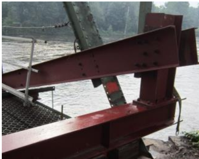
Figure 12.21 End Diagonal Support
