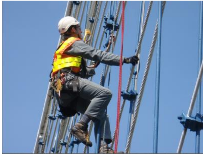
Figure 12.32 Inspection of Stay Cables
