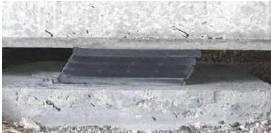
Figure 12.14 Resetting Bearings
