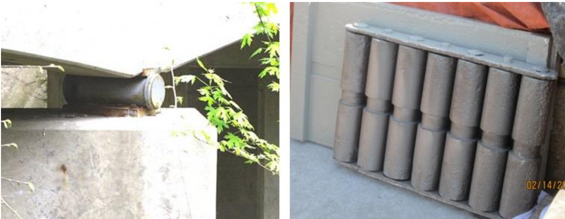
Figure 12.4 Roller bearings. Single Roller (left) and Nested Roller (right).
