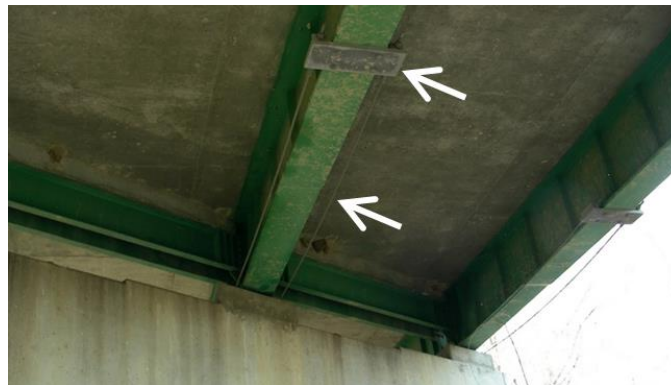
Figure 12.38 Earthquake Restrainer System
