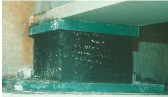
Figure 12.10 Seismic Isolation Bearing
