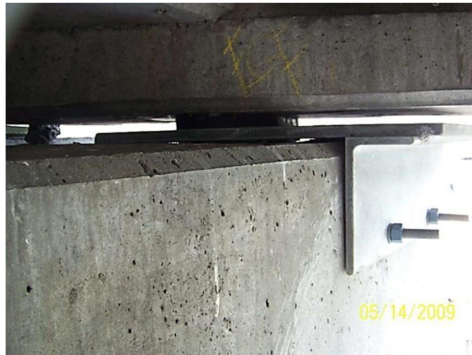
Figure 12.15 Restrainer Plate
