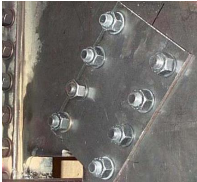
Figure 11.56 Example of Reinforcement Plate Repair
