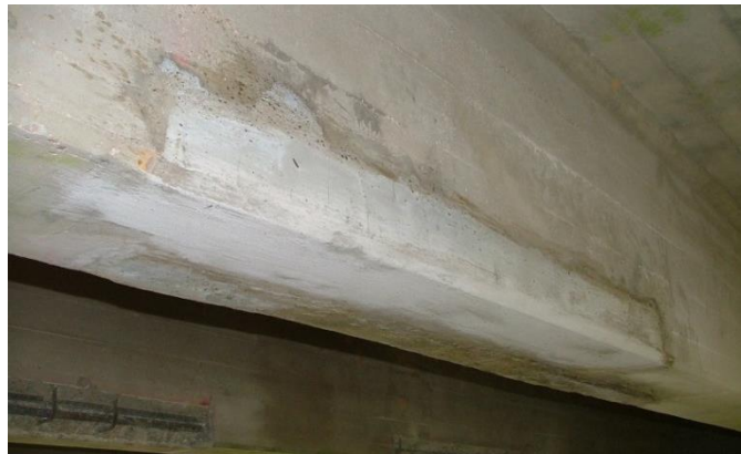
Figure 11.18 Completed Form Repair
