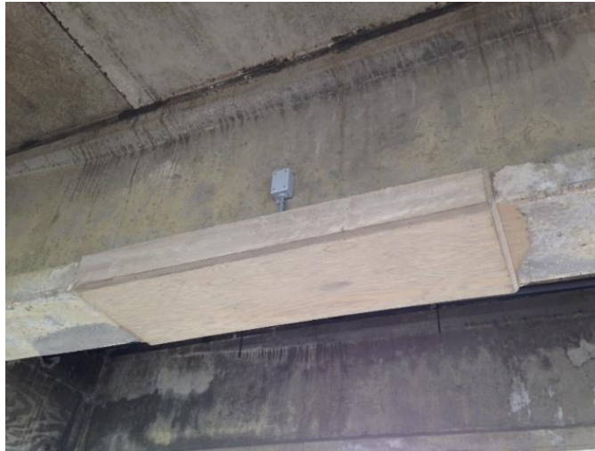
Figure 11.15 Concrete Superstructure with Wood Form (Courtesy of Washington DOT)
