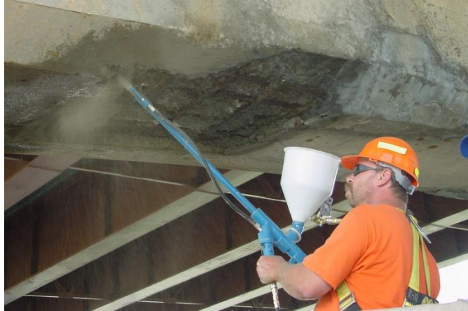
Figure 11.20 Shotcrete Application
