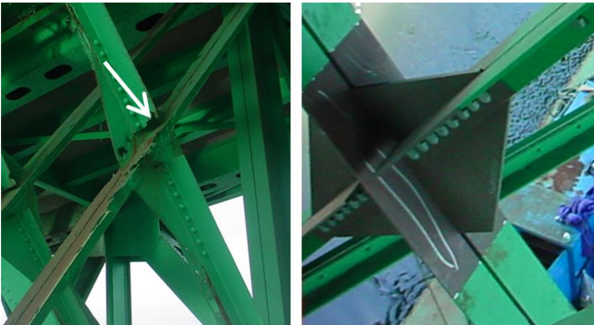
Figure 11.42 Replacement of Bracing and Connection Plate. Before (left) and After (right)
