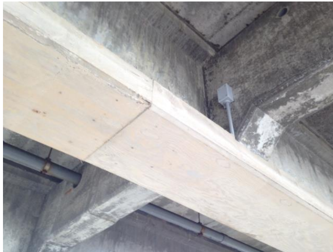
Figure 11.16 Completed Repair of Concrete Superstructure (Courtesy of Washington DOT)
