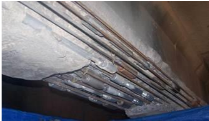
Figure 11.30 Completed Strand Coupling System in Prestressed Girder Repair
