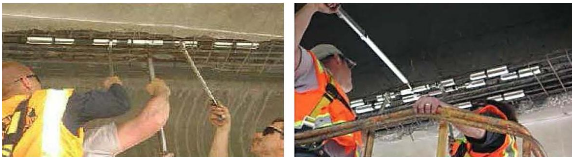
Figure 11.28 Tensioning the Splice (Courtesy of the Nebraska Department of Roads)
