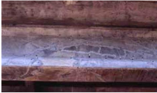
Figure 11.21 Completed Epoxy Crack Repair
