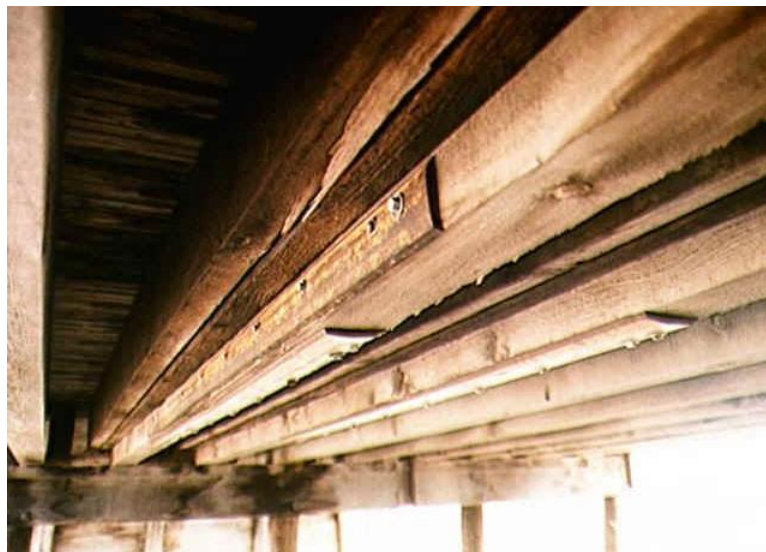
Figure 11.64 Example of Scabbing an Existing Timber Member
