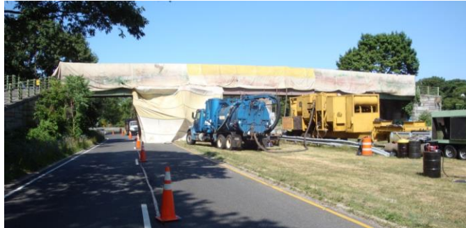
Figure 11.6 Painting Project with Approved Containment System
