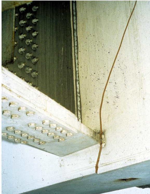
Figure 11.52 Fatigue Crack
