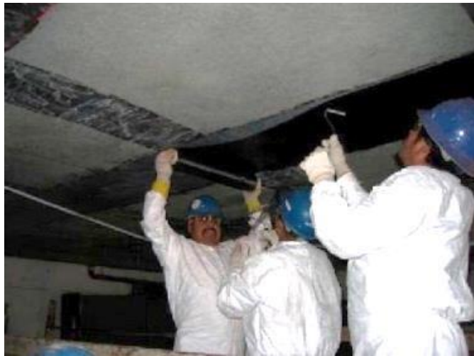
Figure 11.25 Applying FRP to Strengthen a Beam
