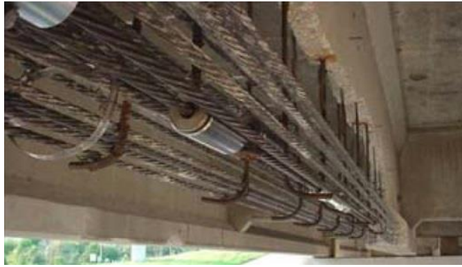
Figure 11.29 Completed Splice Ready for Concrete
