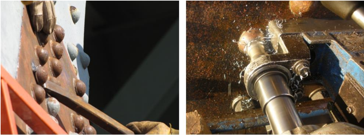
Figure 11.51 Rivet Removal. Pneumatic Rivet Breaker (left) and Drill Removal (right)
