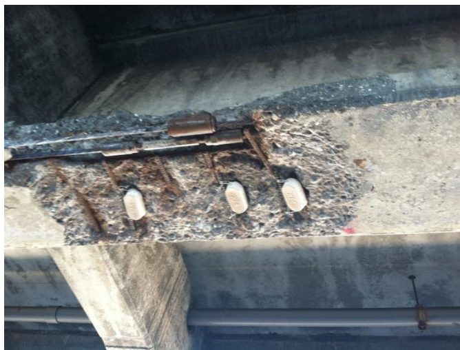
Figure 11.14 Concrete Superstructure Ready for Patch (Courtesy of Washington DOT)
