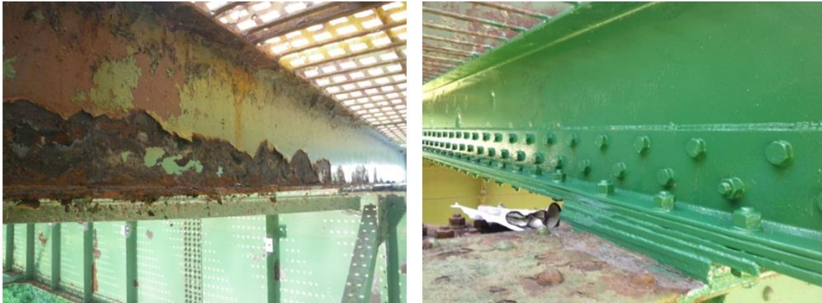
Figure 11.39 Girder Repair. Before (left) and After (right).
