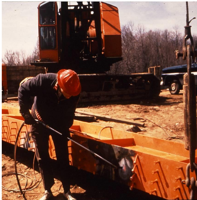
Figure 11.60 Example of Heat Straightening Procedure
