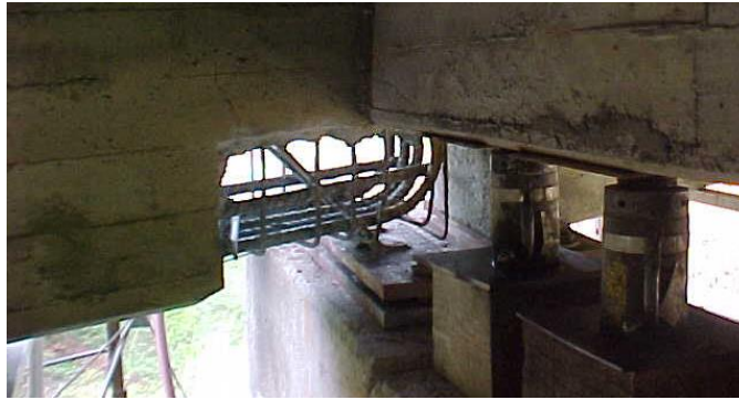
Figure 11.23 Beam End Repair Preparation
