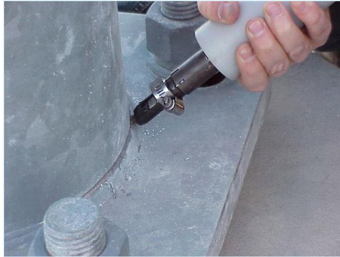
Figure 11.7 Peening of Weld using Ultrasonic Impact Technology
