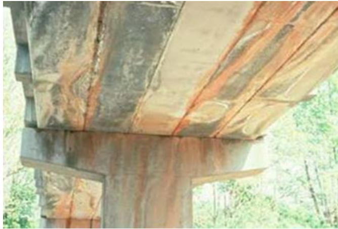
Figure 11.31 Underside of Adjacent Box Beam
