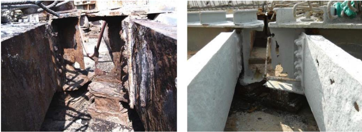
Figure 11.33 Corrosion Damage at Girder Ends (Concrete Deck has been Removed)
