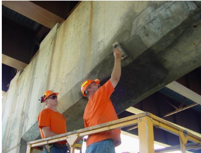
Figure 11.13 Patching of Concrete Superstructure (Courtesy of the New York State DOT)
