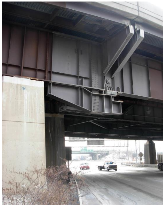
Figure 18.23 Zone Painted Below / Near a Roadway Expansion Joint
