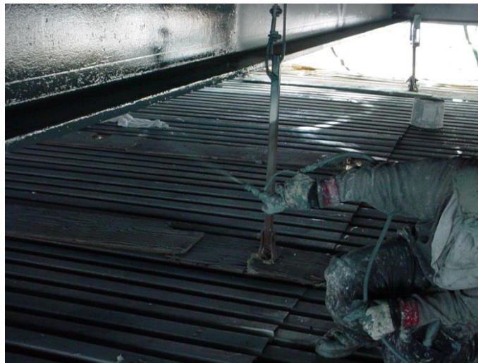
Figure 18.42 Airless Spray Application on a Bridge Project
