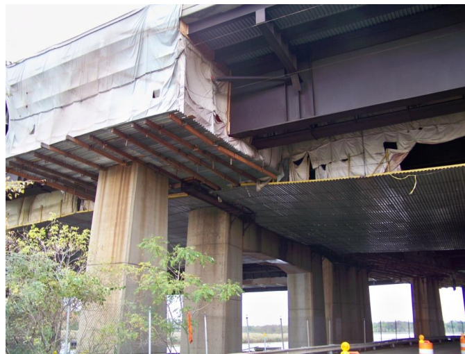
Figure 18.24 Class 1A Containment for Zone Painting
