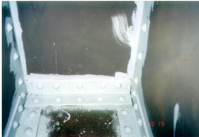
Figure 18.40 Stripe Coat Inside a Chord Member
