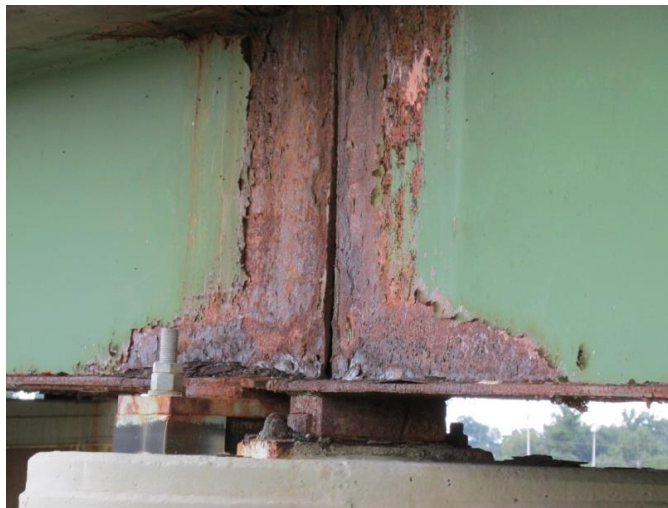
Figure 18.13 Example Beam End and Bearing Zone
