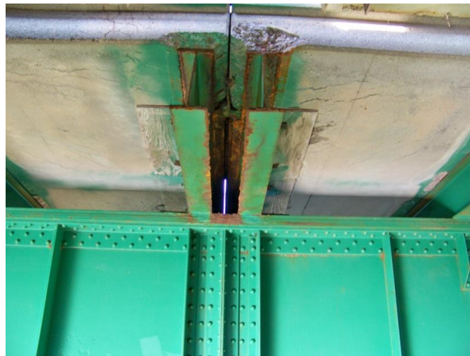
Figure 18.17 Deck Relief Joint is a Potential Painting Zone
