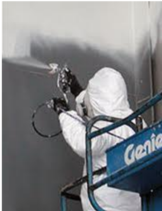
Figure 18.41 Airless Spray Application
