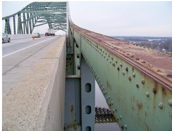
Figure 18.19 Truss Near Roadway Level in the Splash Zone
