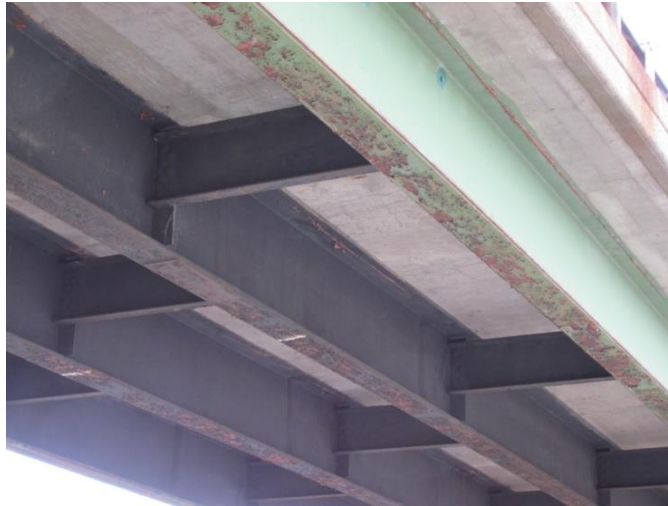
Figure 18.14 Underside of the Bridge
