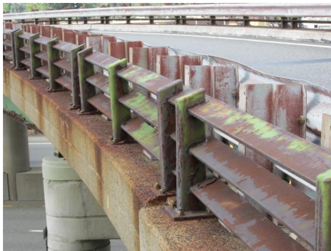
Figure 18.15 Railing on the Top Deck. Roadway Splash Zone.
