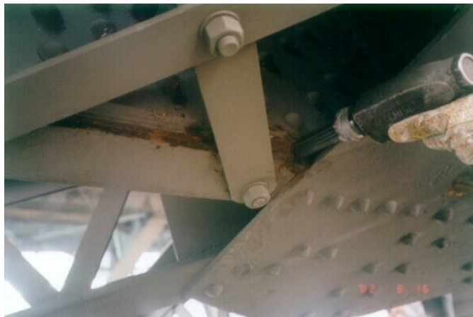
Figure 18.32 Needle Gun Cleaning for Spot Repairs to a Bridge Coating
