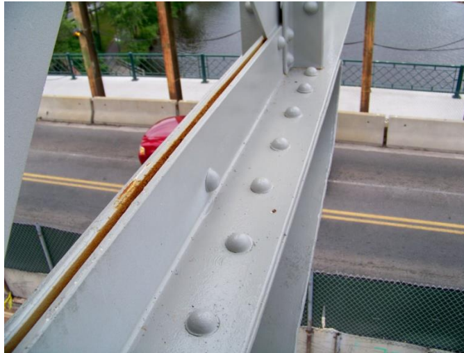
Figure 18.10 Back-to-Back Angles May Require Alternate Methods to Apply Coatings
