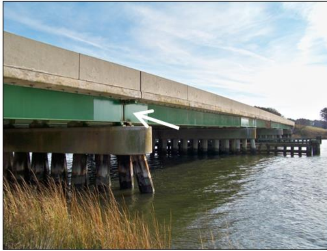
Figure 18.16 Beam End and Bearing Zone Painting
