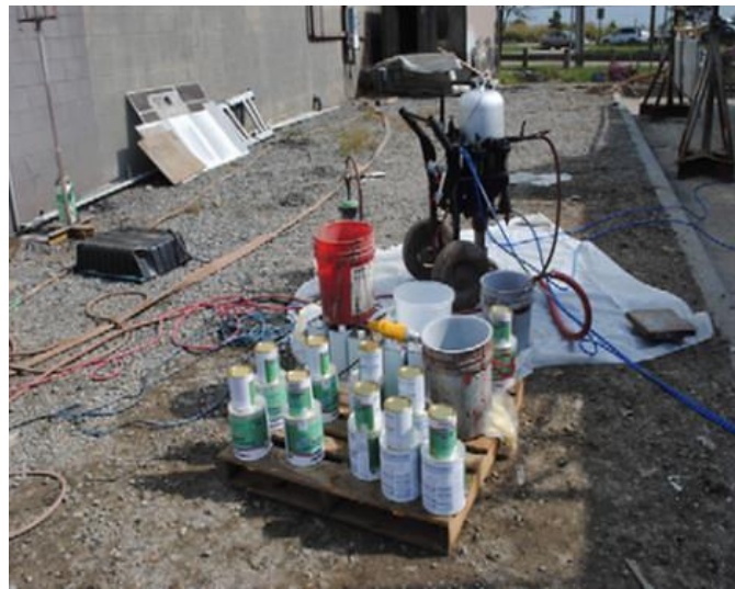
Figure 18.39 Mixing Area for Coatings (Courtesy of SSPC)
