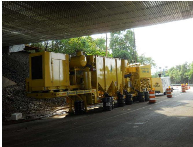
Figure 18.34 Recyclable Steel Grit Machine Used for Abrasive Blasting
