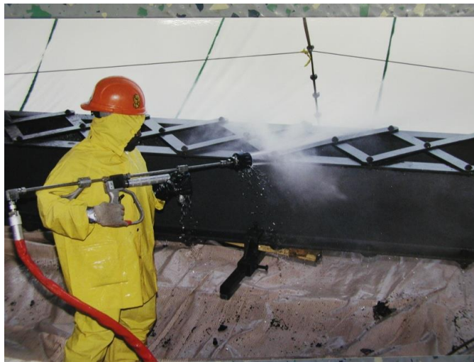
Figure 18.28 HP Water Cleaning on a Bridge (10,000 psi)
