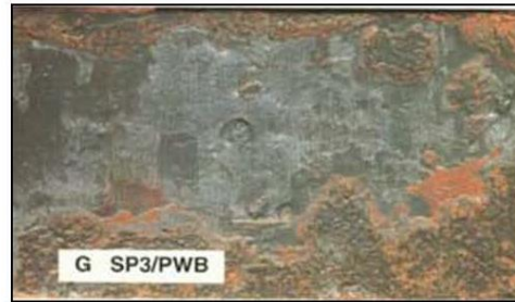
(b) Condition G cleaned to SP3 using power wire brush
