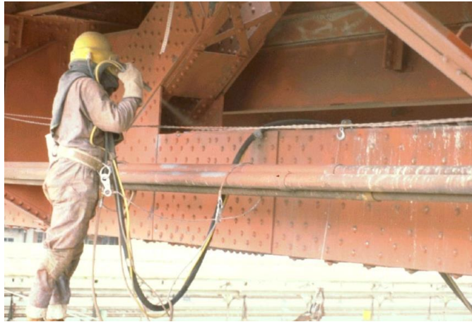
Figure 18.35 Abrasive Blasting on a Bridge (Courtesy of SSPC)
