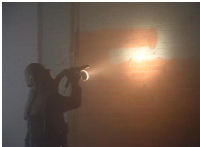
Figure 18.36 Abrasive Blasting with Disposable Abrasive
