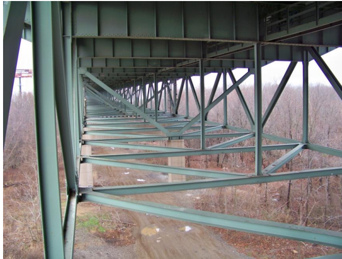
Figure 18.20 Bridge Underside Zone on a Deck Truss
