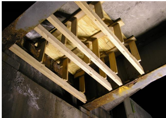
Figure A.36 Example of Form Constructed on Deck Underside
