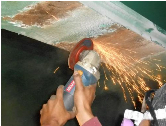
Figure A.9 Mechanical Removal of Paint
