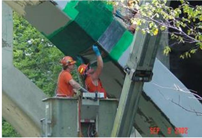
Figure A.37 Hand Lay-Up of Saturated Fabric
