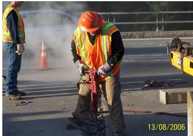
Figure A.20 Chipping out Concrete at Joint
