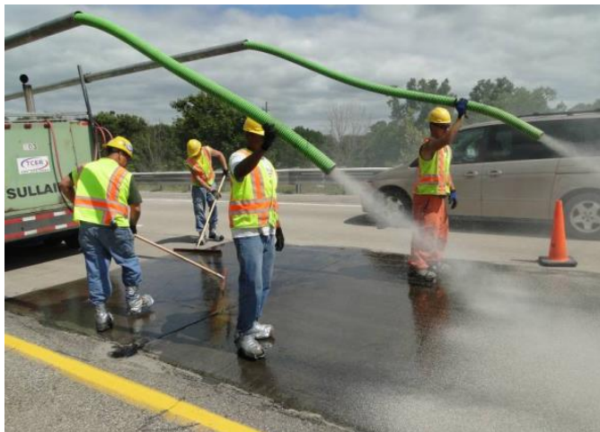
Figure A.32 Broadcasting Sand using a Mechanized Application (Courtesy of MDOT)
