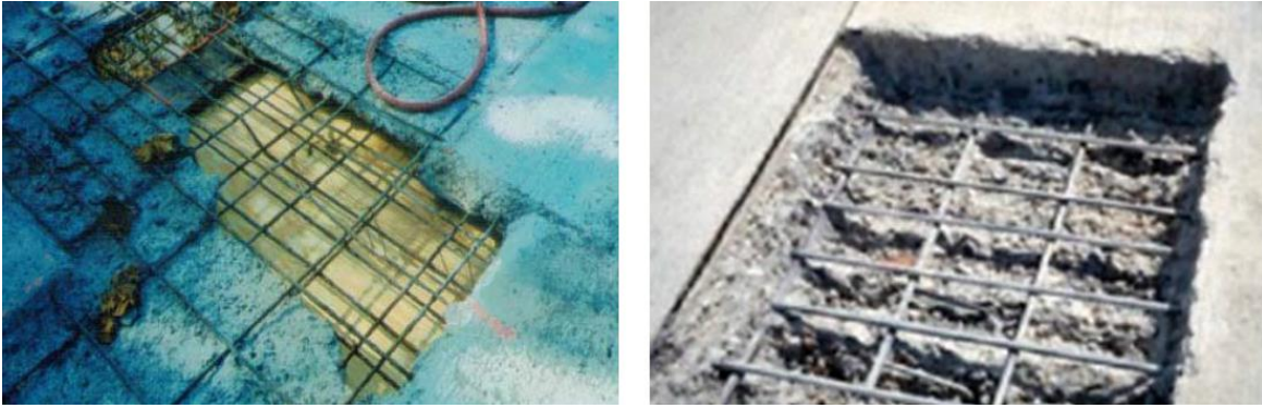
Figure A.35 Deteriorated Concrete Removal and Exposed Steel Cleaned
