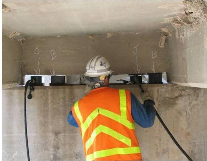
Figure A.25 Example of Jacked Structure
