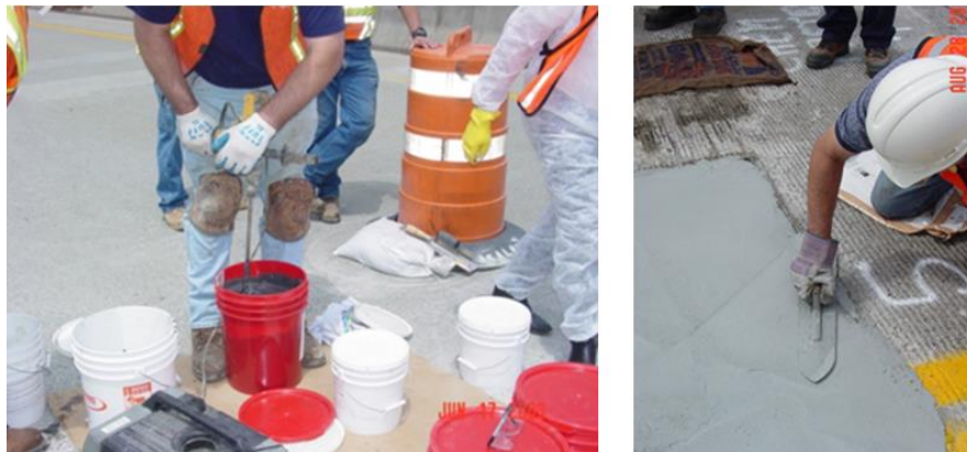
Figure A.18 Mixing Patching Material (left) and Patch Concrete Placement (right)
