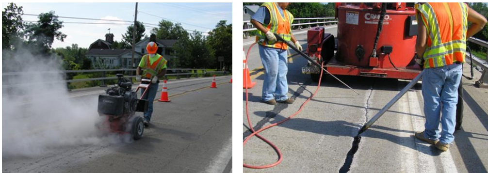
Figure A.3 Crack Sealing in Concrete Decks
