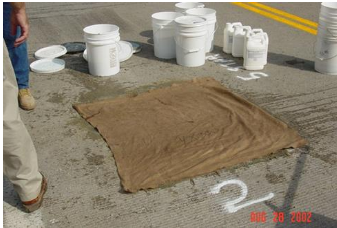
Figure A.19 Example of Wet Cure
