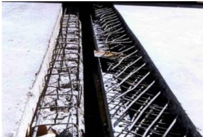
Figure A.21 Removed Joint System
