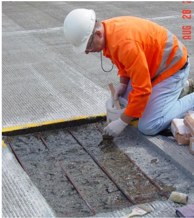
Figure A.17 Bonding Agent Application
