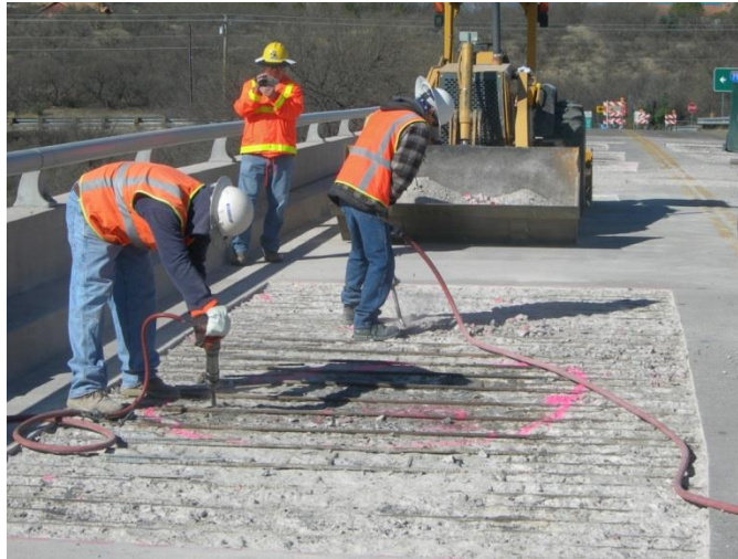
Figure A.16 Deteriorated Concrete Removal (Courtesy of Kwikbond Polymers)
