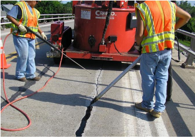
Figure A.2 Applying a Crack Sealer
