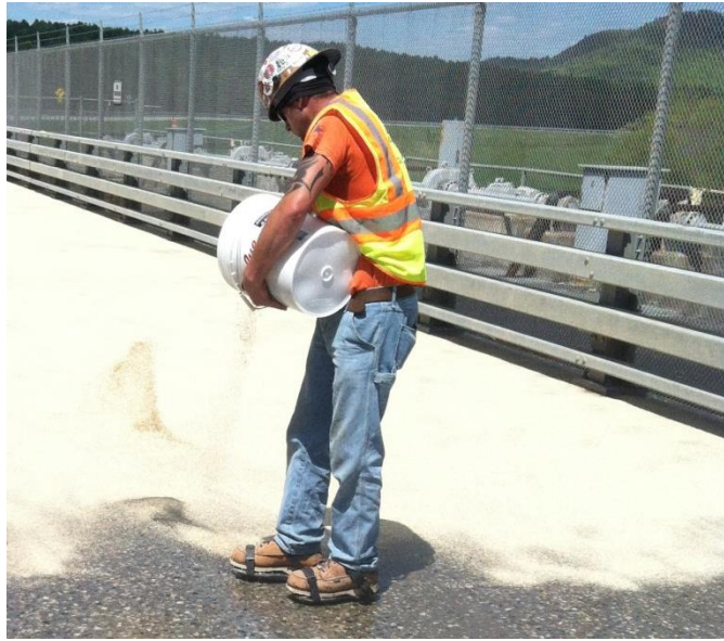
Figure A.30 Broadcasting Aggregate by Hand
