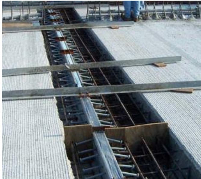
Figure A.22 Box Preparation for New Joint
