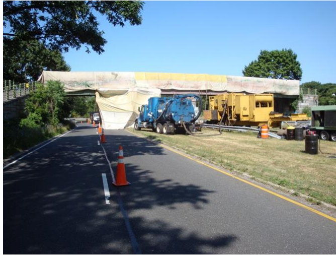
Figure A.12 Painting Project with Approved Containment System
