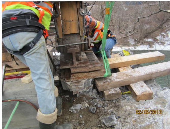
Figure A.27 Example of Bearing Removal
