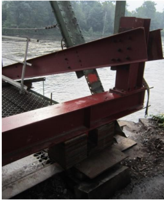
Figure A.23 Temporary Support
