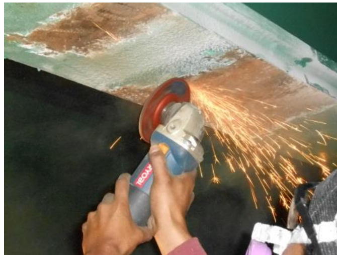
Figure A.14 Mechanical Removal of Paint
