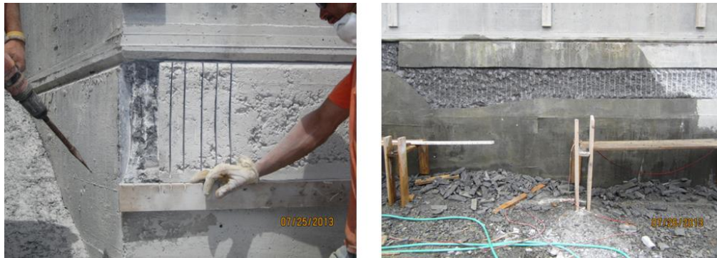
Figure A.28 Deteriorated Concrete Removal
