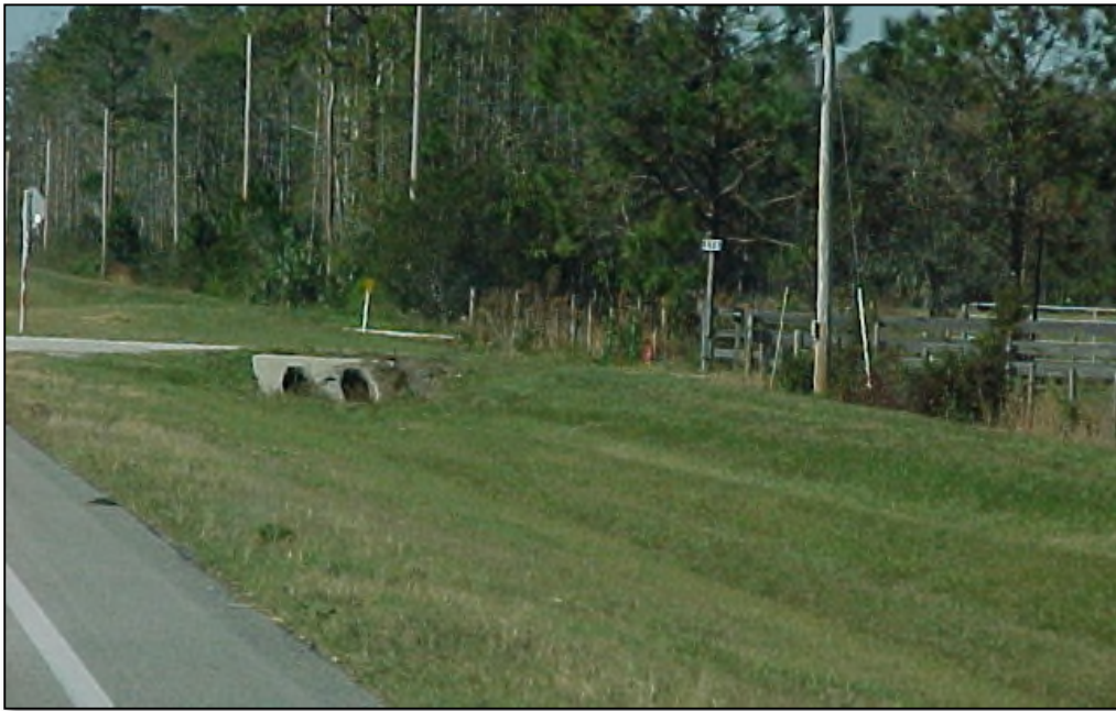
Roadside ditch with side drainpipe.
