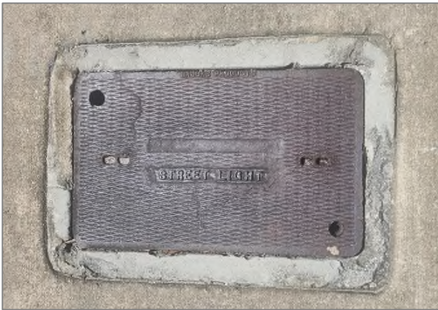
Pull box missing bolts. This would not meet conditions.
