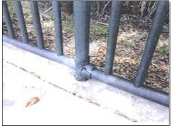
Cracked or broken hardware would not meet desired maintenance conditions.
