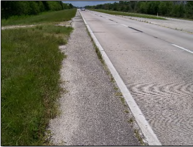
Examples of unwanted vegetation growing out of cracks in pavement.
