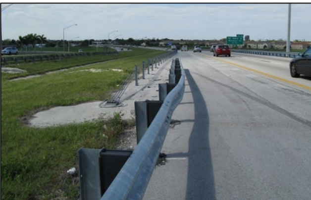
End anchor for SAFENCE behind guardrail.
