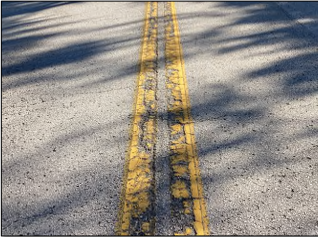
Worn out striping does not meet MRP standards.
