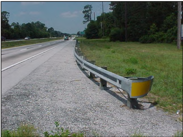
This end section has been hit and does not meet MRP standards.
