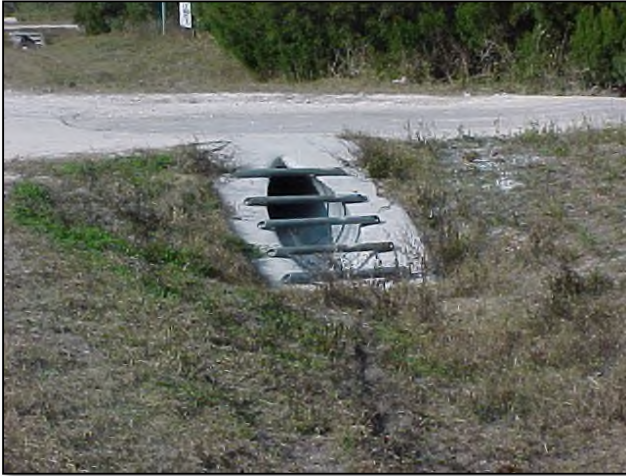
This is a side drainpipe with grates. This meets MRP standards.
