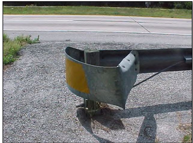
This damaged end section does not meet MRP standards.
