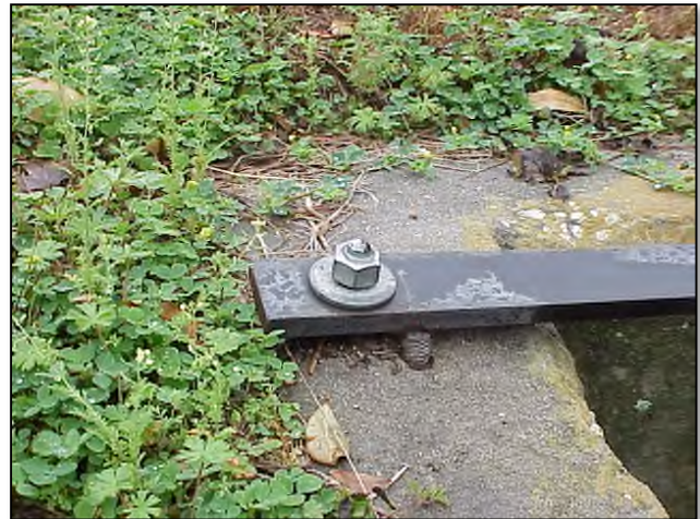
Repaired grate. Epoxy bolt. Meets conditions.
