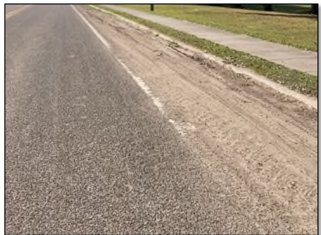
Edge line obscured by soil or other debris does not meet MRP standards.
