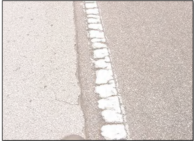
Worn out edge line does not meet MRP standards.
