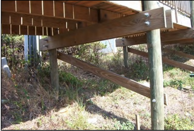
Support piling / post with bracing.
