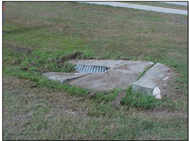
Side/cross drainpipe with 3 or more cracks > ½ in. wide 1 ft. in length. This does not meet MRP standards.
