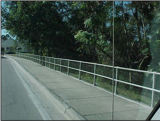
Handrail meets desired maintenance conditions.
