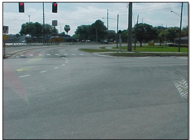
These skip lines are an example of radius markings.
