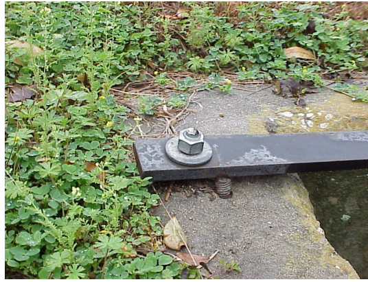
Repaired grate. Epoxy bolt. Meets conditions.
