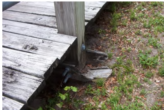
Deterioration of supports.
