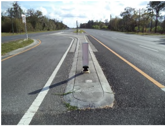
Paddle type, high visibility flexible delineators
