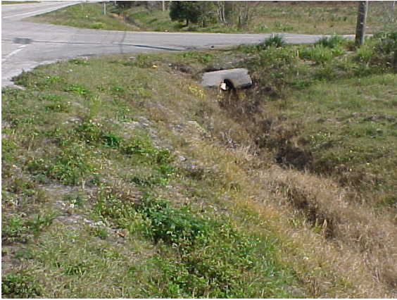
Side drain pipe under turnout.
