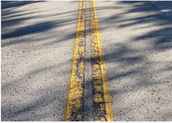
Worn out stripping does not meet MRP standards.
