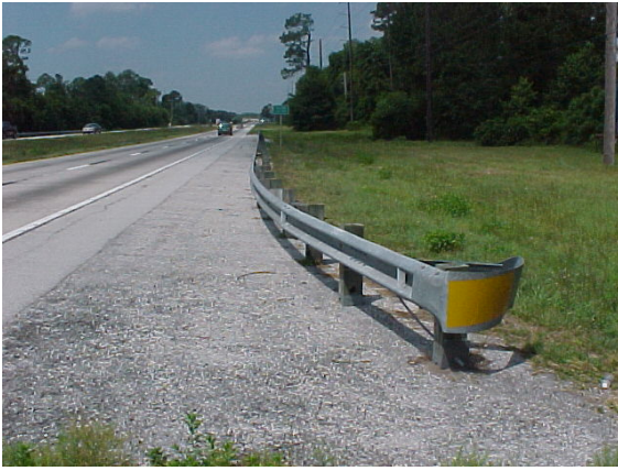
This end section has been hit and does not meet MRP standards.
