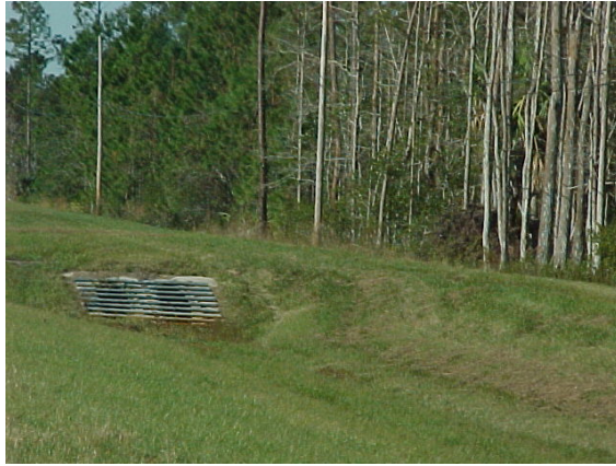
Side drain pipe with grates.
