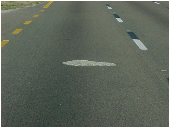
Concrete spill, rate as a bump.
