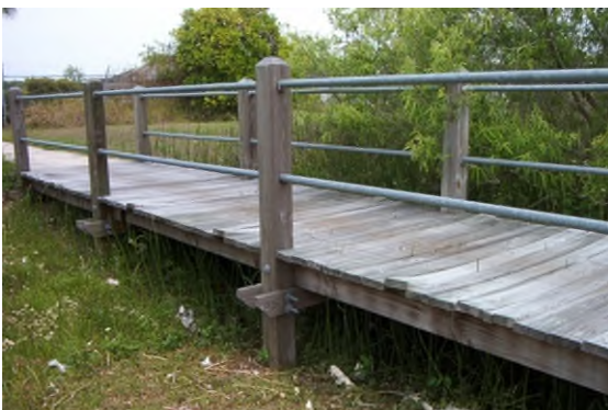
Surface deck boards with misalignments.
