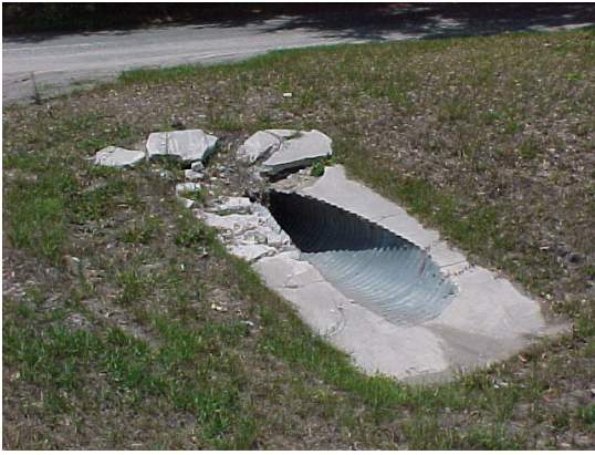
Side drain pipe with damaged concrete.
