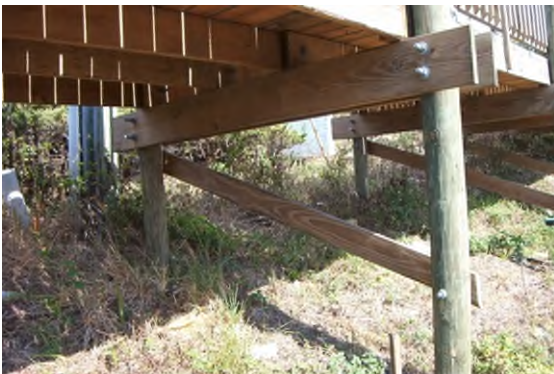
Support piling / post with bracing.
