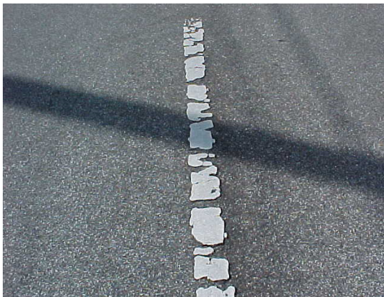
Edge line does not meet MRP standards.
