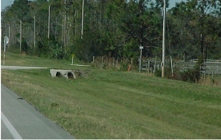
Roadside ditch with side drain pipe
