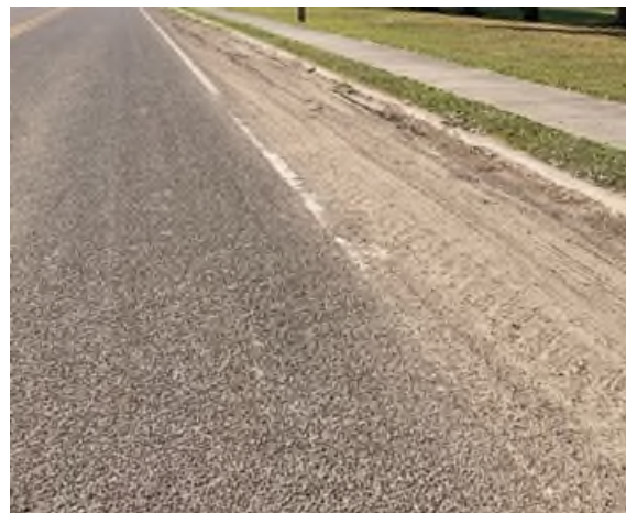
Edge line obscured by soil or other debris does not meet MRP standards
