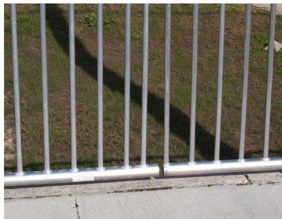
Picket railing missing steel sleeve at expansion joint. This does not meet MRP standards.
