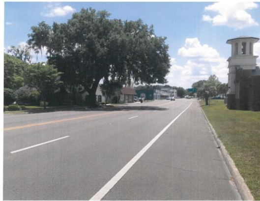
Examples of trees over roadway if measured lower than 14½ feet it would not meet MRP standards.
