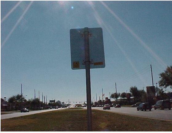
Evaluate only FDOT signs. This sign has the proper label indicating when it was installed and that it is the property of FDOT.
