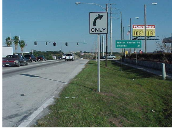
Rate ground mounted signs according to Design Index used for installation.
