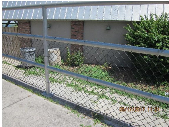
Handrail with wired mesh meets desired maintenance conditions.
