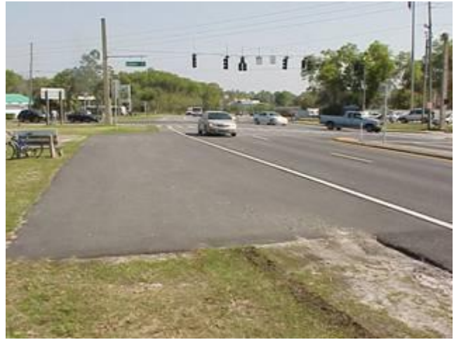
Asphalt bus turnout on rural roadway. This should be rated as roadway pavement, also rate for edge raveling. (Note: Rate only the edge of pavement parallel to the travel lanes for raveling)
