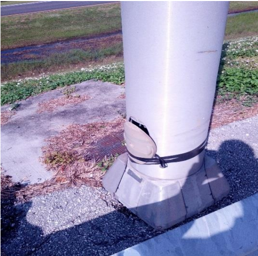
This would not meet conditions as properly secured.
