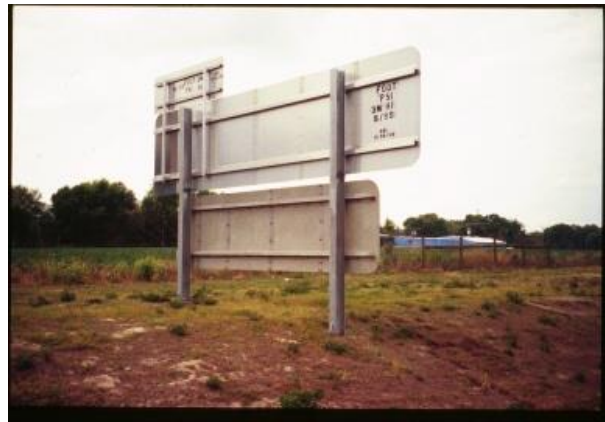
This breakaway device is covered and does not meet MRP standards unless behind a barrier.
