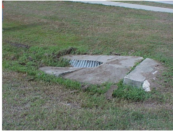
Side/cross drain pipe with 3 or more cracks > ½ in. wide 1 ft. in length. This does not meet MRP standards.
