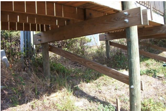
Support piling / post with bracing.
