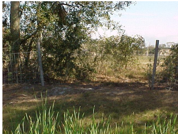
This fence has been cut and is open. This does not meet MRP standards.
