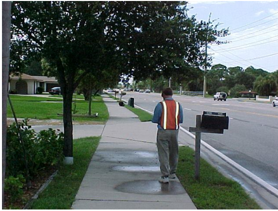
This tree limb appears lower than 8½ feet over the sidewalk. This does not meet MRP standards.
