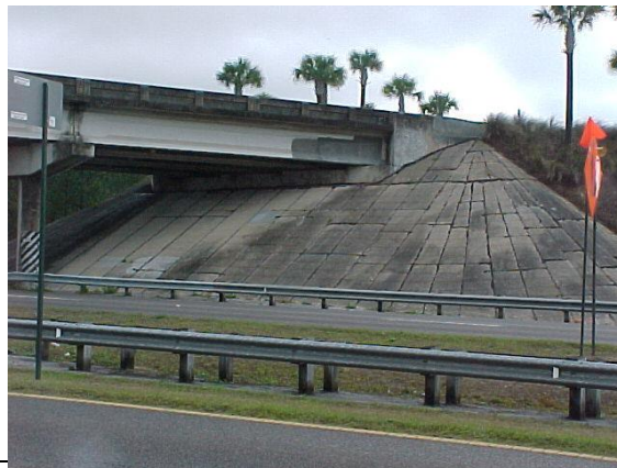
This is an example of concrete slope pavement.
