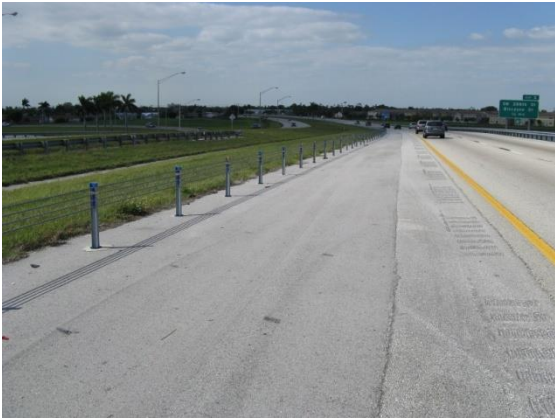
SAFENCE Post installation is similar to CASS but with 4 cables.
