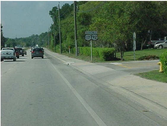
This is an urban flared turnout. The sidewalk should be projected across the turnout and evaluated as sidewalk. In this case turnout would not be evaluated.
