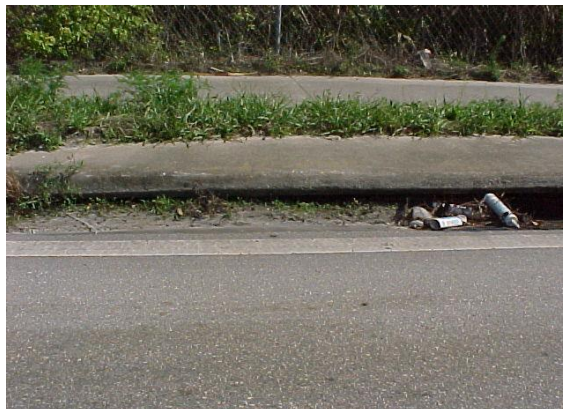
Soil buildup at curb inlet. Determine the percentage of opening area obstructed and compare to the standard.
