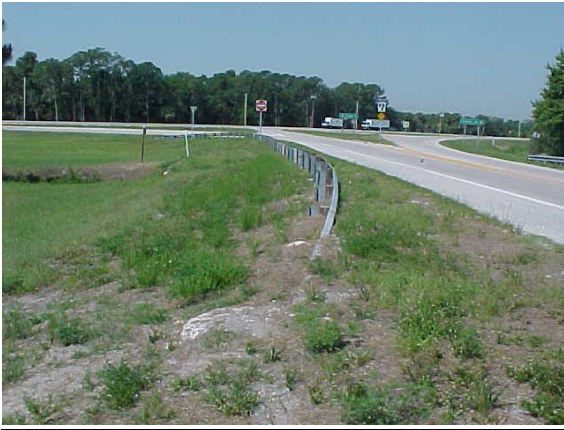
Buried end guardrail section. Guardrail shall be evaluated according to the index it was installed under. This may meet MRP standards.
