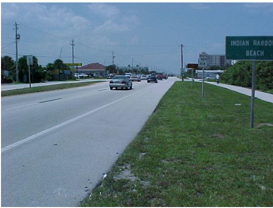
This is an example of a soil shoulder that meets MRP standards.
