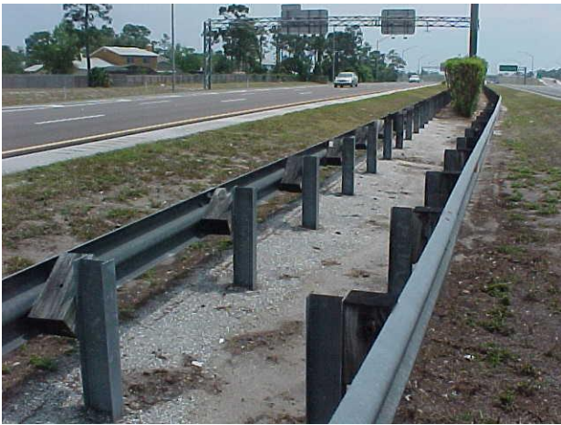
The offset blocks in these pictures are not aligned properly. If more than 10% of the blocks in a guardrail run are twisted it would not meet MRP standards.
