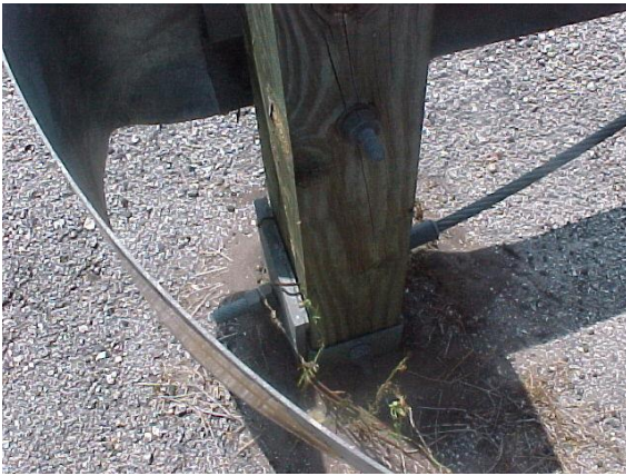
The bearing plate must be secured to prevent rotation
