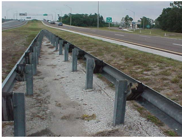
The offset blocks in these pictures are not aligned properly. If more than 10% of the blocks in a guardrail run are twisted it would not meet MRP standards.
