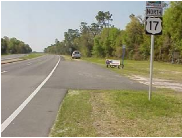
Asphalt bus turnout on rural roadway. This should be rated as roadway pavement, also rate for edge raveling. (Note: Rate only the edge of pavement parallel to the travel lanes for raveling)
