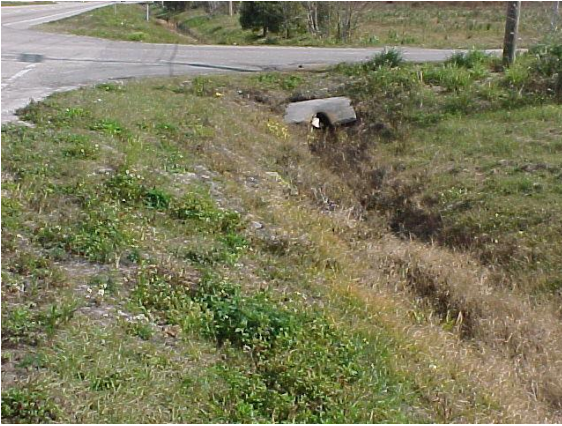
Side drain pipe under turnout.
