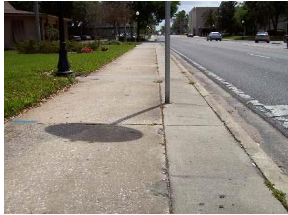
These pictures are examples of utility strips that have been paved with brick and concrete. For MRP purposes these areas should be rated as sidewalk.
