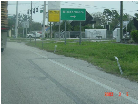
These post-mounted delineators would not be rated because they are being used to prohibit unauthorized traffic movements.
