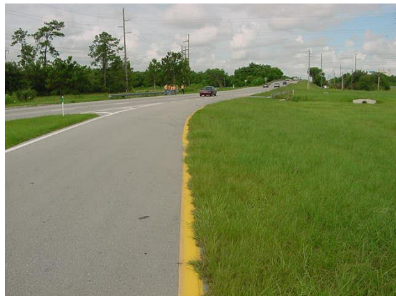
Edge line obscured by grass does not meet MRP standards.
