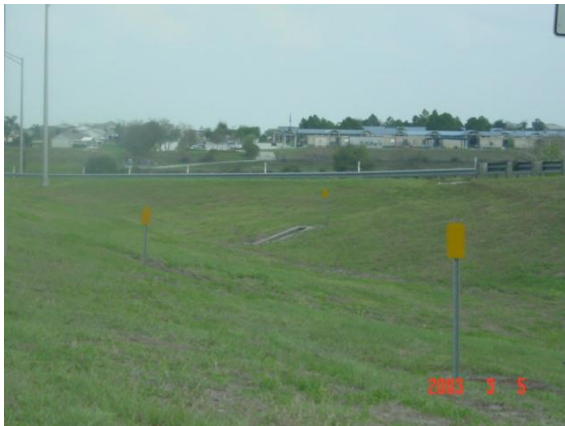
Object markers are used to mark obstructions within or adjacent to the roadway. These object markers are marking a manhole, head- wall and U-end wall.
