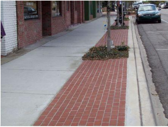
These pictures are examples of utility strips that have been paved with brick and concrete. For MRP purposes these areas should be rated as sidewalk.
