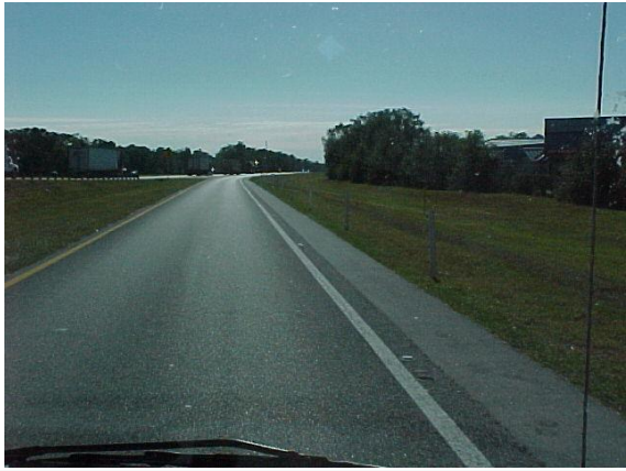
These post mounted delineators are installed on a ramp according to Standard Plans.
