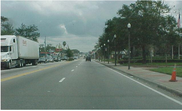
Existing white edge line on an urban curb & gutter section. This meets MRP standards.
