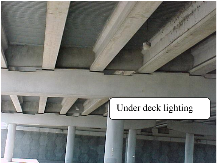
Under highway deck lighting should be included in the evaluation of lighting.
