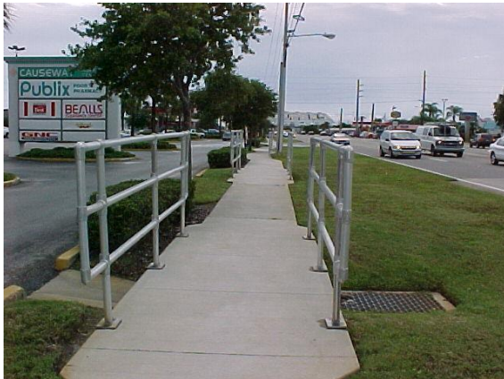
Handrail meets desired maintenance conditions.
