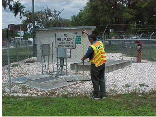
Measure the height of the fence from natural ground to the top of the fence fabric.
