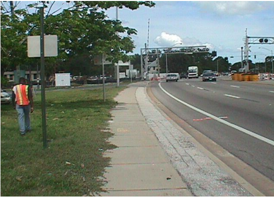
This vegetation is encroaching onto the sidewalk more than 6 inches for a continuous 10 feet. This does not meet MRP standards for curb/ sidewalk edging.
