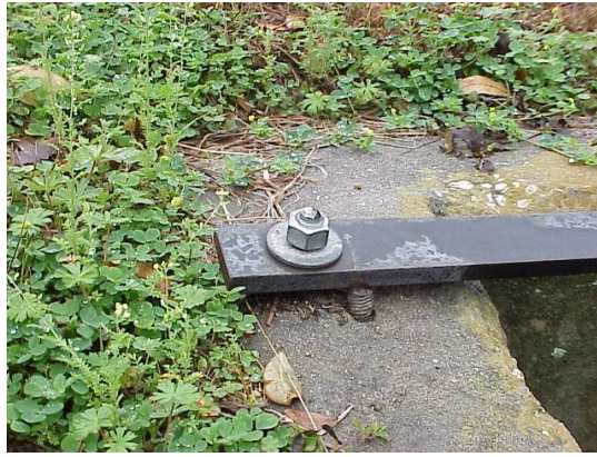
Repaired grate. Epoxy bolt. Meets conditions.
