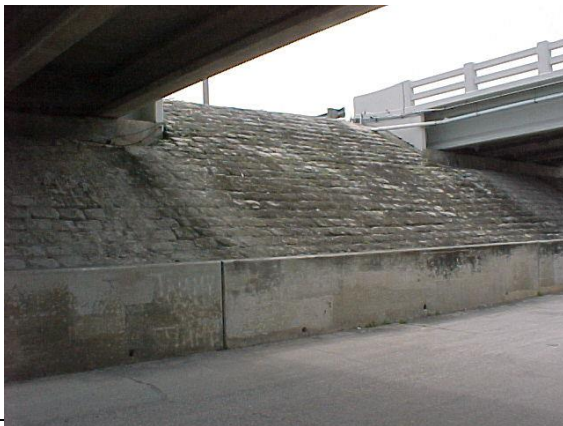
This is an example of rip-rap slope pavement.
