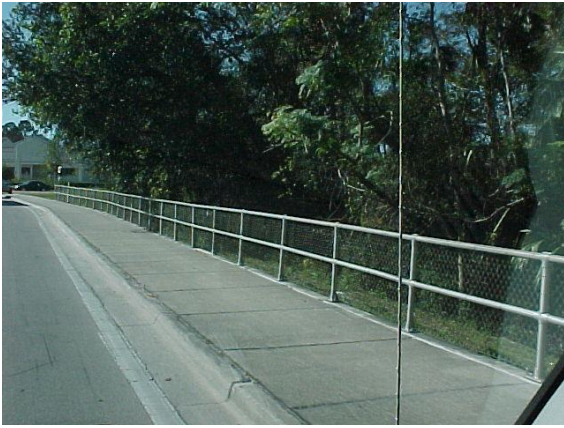
Handrail meets desired maintenance conditions.
