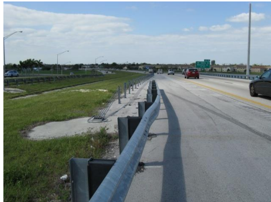
End anchor for SAFENCE behind guardrail.
