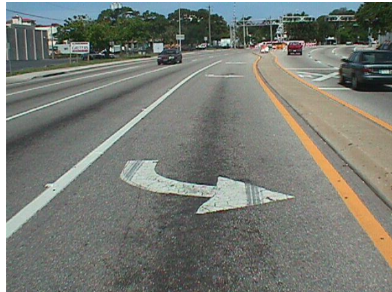
Pavement symbols in good condition, meets MRP standards.
