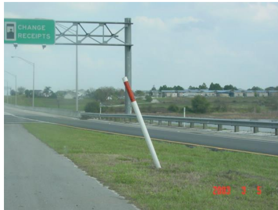
This object marker is for fiber optic cable. It would not be rated since this is not a roadway department maintained object.
