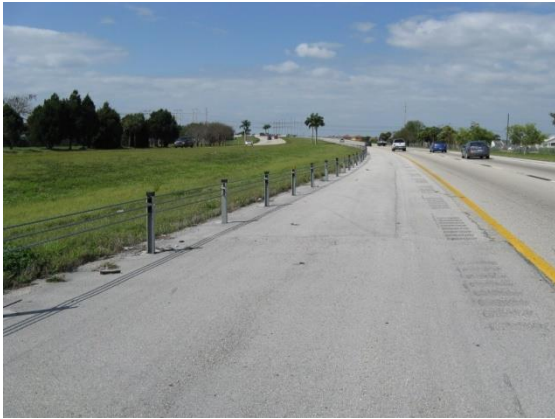
CASS Cable Safety System: C-shaped posts Installed in a sleeve driven into asphalt or set in concrete foundation. 3 cables in a slot at the Top of the post separated by plastic spacers.
