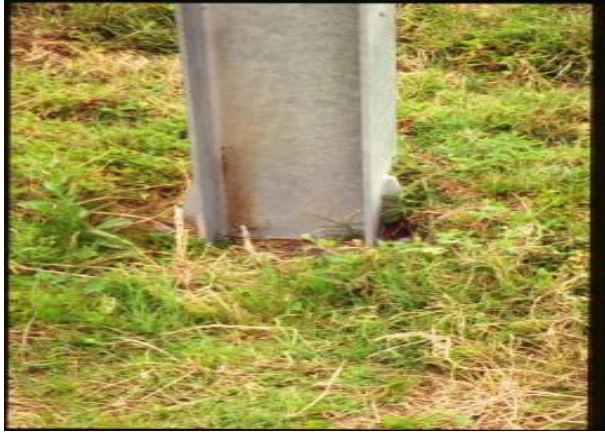
This breakaway device is covered and does not meet MRP standards unless behind a barrier.
