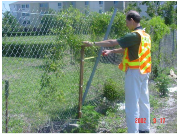
Fence fabric should be attached securely to two consecutive fence post. Fence posts should be in place and functioning as intended.
