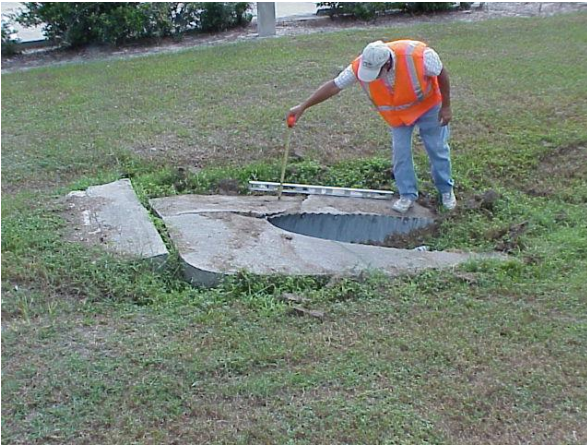
Side/cross drain pipe with 3 or more cracks > ½ in. wide 1 ft. in length. This does not meet MRP standards.
