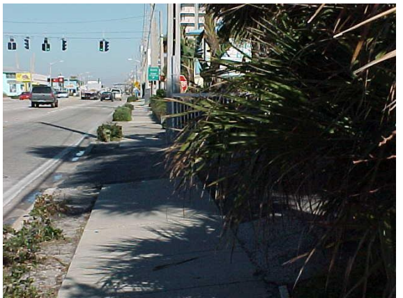
These pictures are examples of vegetation growing over the sidewalk. This obstructs the use of the sidewalk by pedestrians. If there is encroachment of vegetation onto the sidewalk more than 6 inch it does not meet MRP standards.
