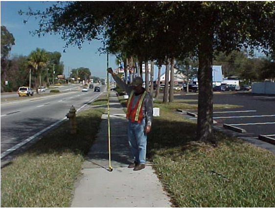
Trees, tree limbs or vegetation should be no lower than 8½ feet over sidewalk. This does not meet MRP standards.
