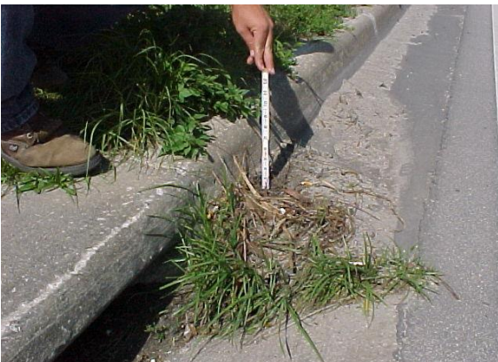
Soil buildup at curb inlet. Determine the percentage of opening area obstructed and compare to the standard.
