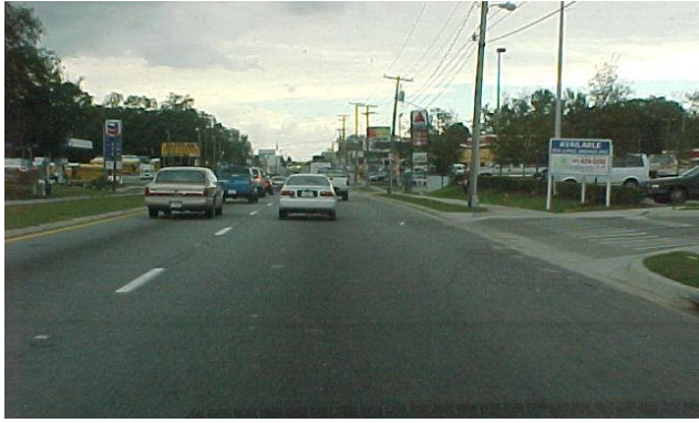
No white edge line on this urban curb & gutter section. This also meets MRP standards.
