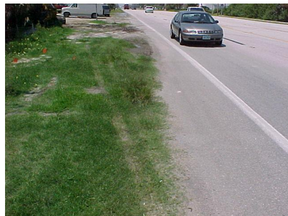
Build-up of sand, soil, and vegetation of unpaved shoulder onto outside paved shoulder.
