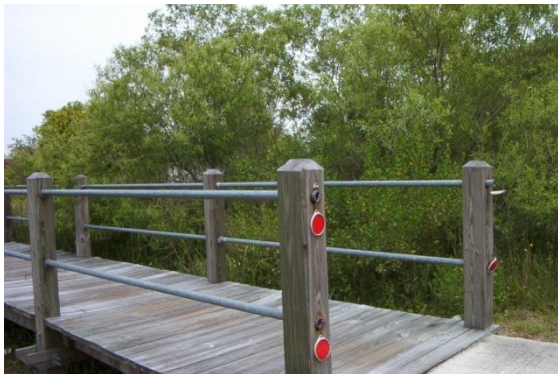
Pipe handrail
