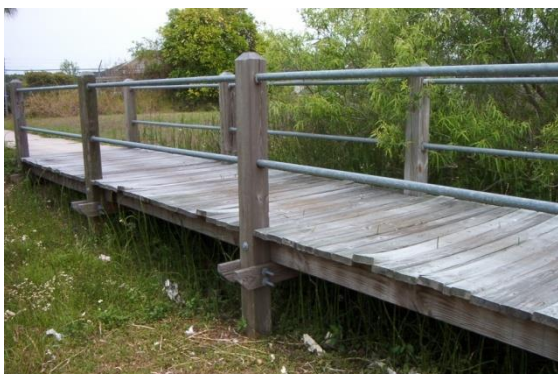
Surface deck boards with misalignments.
