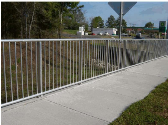
Picket railing protecting drop-off next to sidewalk.
