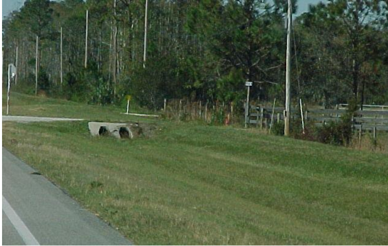
Roadside ditch with side drain pipe
