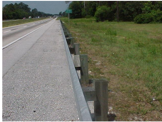
Guardrail offset blocks are not aligned properly. This condition does not meet MRP standards if more than 10% are twisted.
