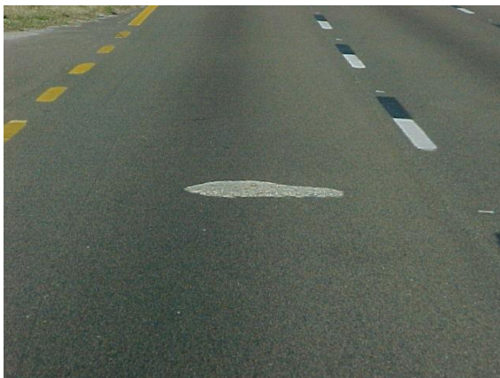
Concrete spill, rate as a bump.
