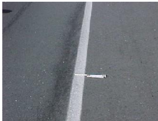
These pictures show painted yellow and white edge lines installed on a newly constructed or resurfaced roadway. Evaluate according to the striping characteristic.
