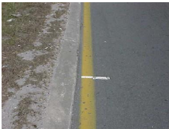
These pictures show painted yellow and white edge lines installed on a newly constructed or resurfaced roadway. Evaluate according to the striping characteristic.
