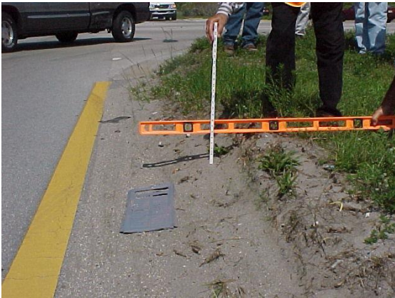
High shoulder 2 inches or more for 25 continuous feet does not meet MRP Standards.
