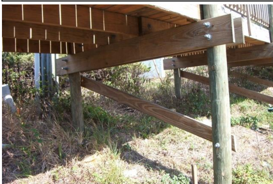
Support piling / post with bracing.
