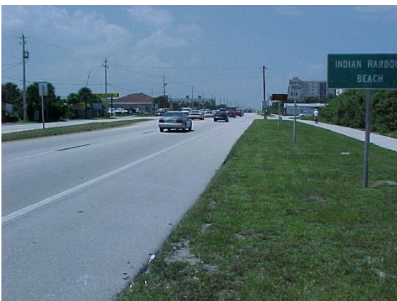
This is an example of a soil shoulder that meets MRP standards.
