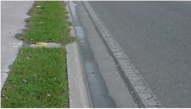
Worn out edge line does not meet MRP standards.
