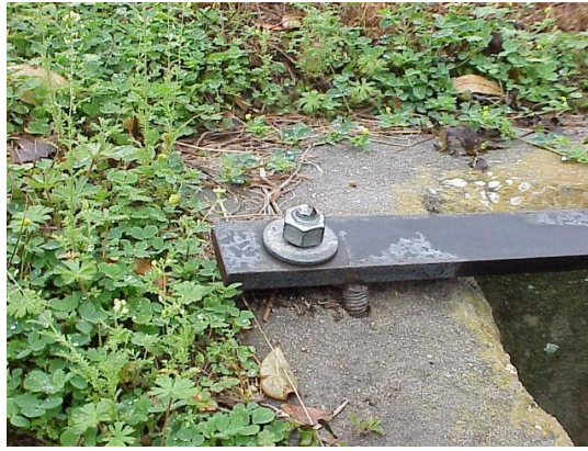
Repaired grate. Epoxy bolt. Meets conditions.
