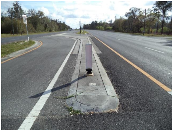
Paddle type, high visibility flexible delineators
