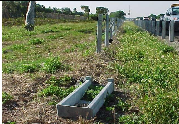
Damaged GIBRALTAR end anchor. This does not meet MRP standards.
