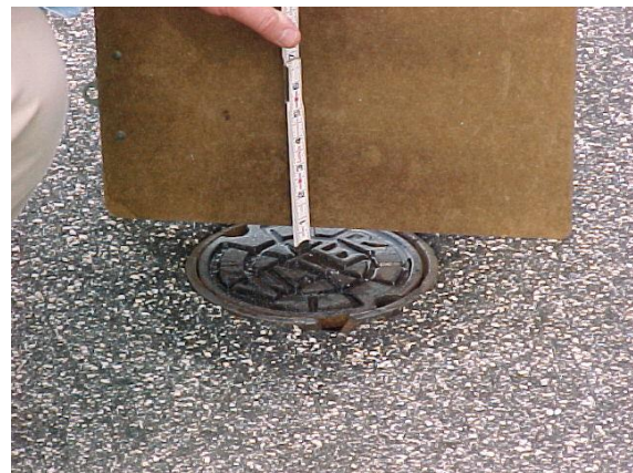
Depression at a water valve in pavement.
