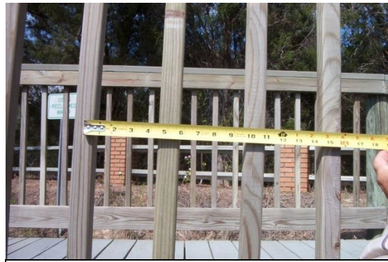
Spindles or pickets on handrail
