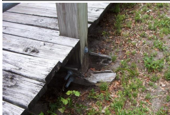
Deterioration of supports.
