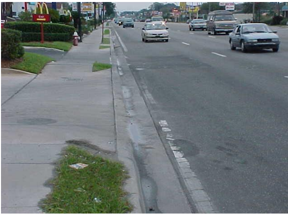
Worn out striping in an urban area does not meet MRP standards.
