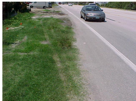
Build-up of sand, soil, and vegetation of unpaved shoulder onto paved shoulder.
