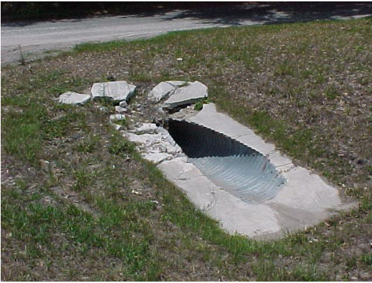
Side drain pipe with damaged concrete.
