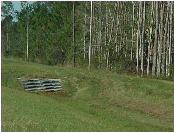
Side drain pipe with grates.
