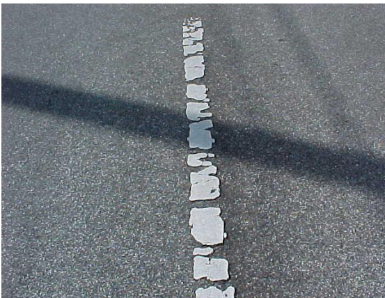
Edge line does not meet MRP standards
