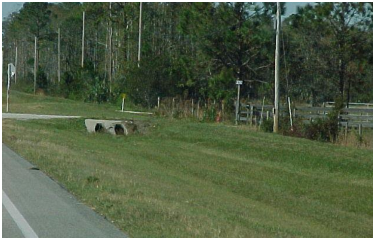
Roadside ditch with side drain pipe
