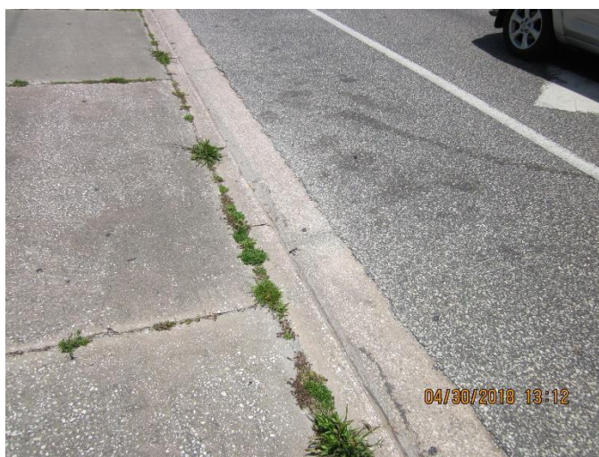
Area may not meet maintenance conditions if more than 7-1/2 square feet of unwanted vegetation for any 50 square foot area of curb/asphalt joint and curb/sidewalk joint.
