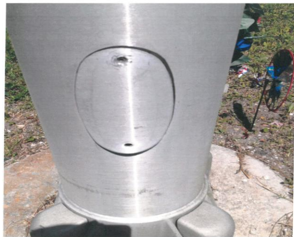
Inspection cover missing screws this would not meet conditions as properly secured.
