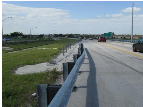
End anchor for SAFENCE behind guardrail.
