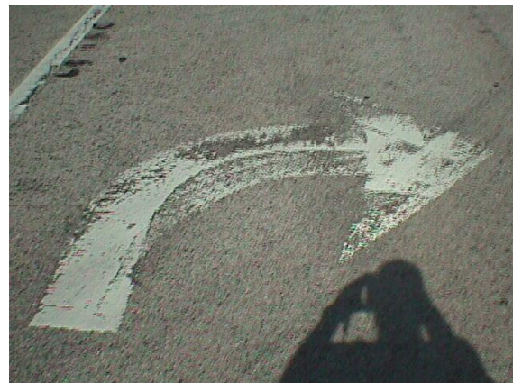
These pictures are examples of worn out symbols. If more than 10% of the cumulative symbol area or 50% or less of any one symbol is not functioning as intended then this would not meet MRP standards.
