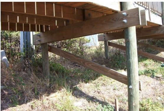
Support piling / post with bracing.
