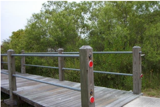
Pipe handrail
