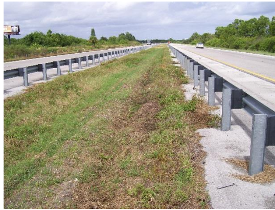
Example of vegetation growing on paved shoulder and under guardrail.
