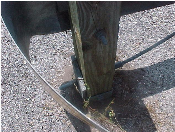
The bearing plate must be secured to prevent rotation
