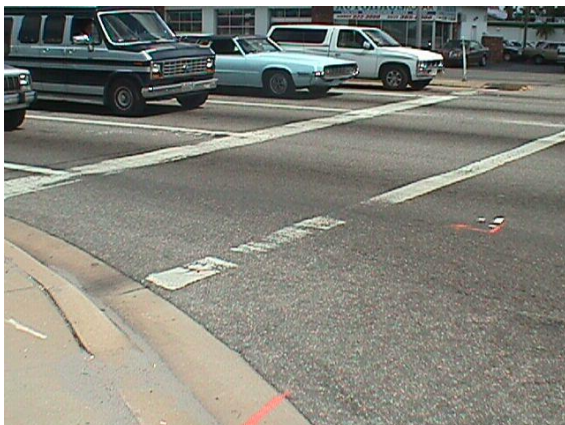
These pictures are examples of worn out symbols. If more than 10% of the cumulative symbol area or 50% or less of any one symbol is not functioning as intended then this would not meet MRP standards.
