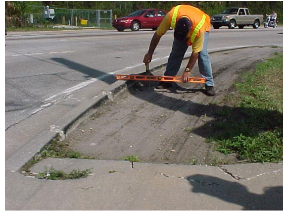
Drop-off behind curb. Since this road has curb & gutter this would be evaluated under curb & sidewalk edging.
