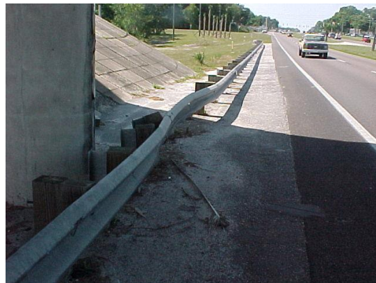
This guardrail has been damaged by a crash. Several posts are damaged. This does not meet MRP standards.
