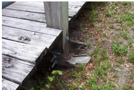
Deterioration of supports.
