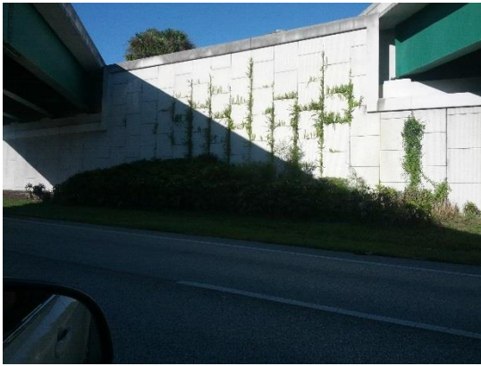
Example of vegetation growing on an MSE wall.
