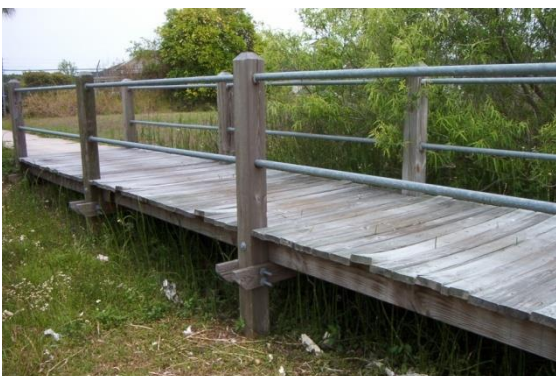
Surface deck boards with misalignments.
