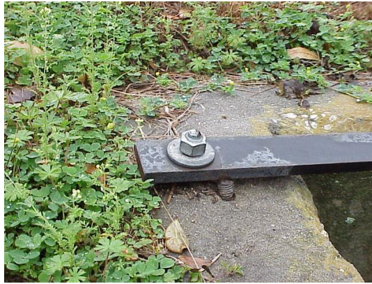
Repaired grate. Epoxy bolt. Meets conditions.
