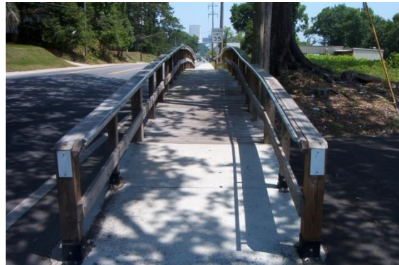
Wood with pipe handrail
