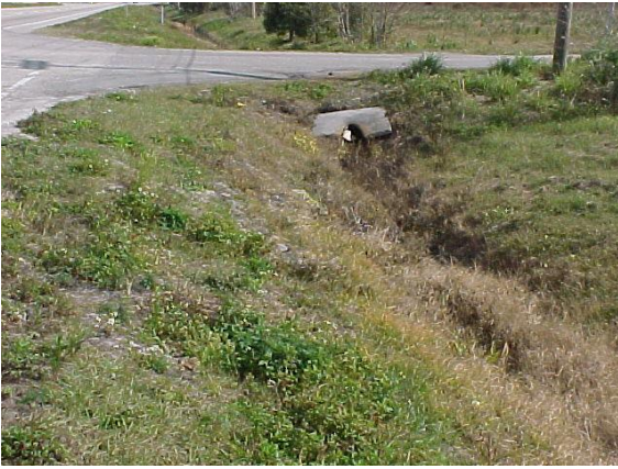
Side drain pipe under turnout.
