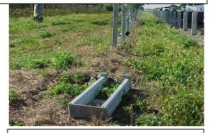
Damaged GIBRALTAR end anchor. This does not meet MRP standards.
