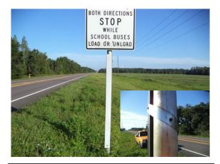
This Retroreflective panel is the correct color but has been riveted into the post. This would not meet maintenance conditions.
