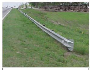
This guardrail section is low and should be measured to determine if it meets MRP standards.
