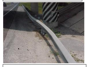
This guardrail has been hit and several posts are missing. This guardrail does not meet MRP standards.
