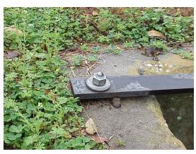
Repaired grate. Epoxy bolt. Meets conditions.
