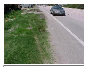
Build-up of sand, soil, and vegetation of unpaved shoulder onto paved shoulder.
