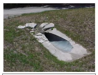
Side drain pipe with damaged concrete. This does not meet MRP standards.
