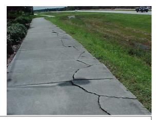
Sidewalk cracking. Measure each horizontal crack greater than ½ inch wide. For MRP purposes, each linear foot of horizontal crack greater than ½ inch equals 1 sq. ft. of crack area. Vertical misalignments greater than 1/4 inch equals 1 sq. ft. of crack area.
