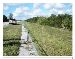
Misaligned cable would not meet desired maintenance conditions.
