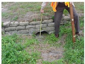
These two pictures show a typical side drain pipe in a roadside ditch. Determine the cross section of the pipe that is not obstructed and functions as intended. If more than 40% of the pipe cross section is obstructed or does not function as intended, then CROSS/SIDE DRAIN does not meet desired maintenance conditions.
