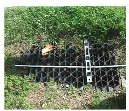
This is an obstructed inlet grate. If the Opening is obstructed more than <u>85%</u>, then it would not meet MRP standard for inlets.
