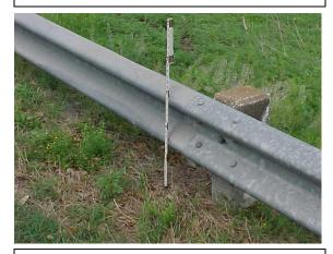
This guardrail section may not meet MRP standards, because the height above the ground is incorrect.
