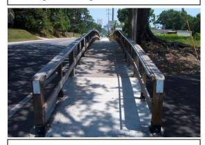
Wood with pipe handrail
