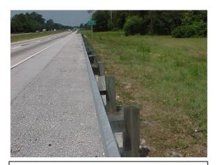
Guardrail offset blocks are not aligned properly. This condition does not meet MRP standards if more than 10% are twisted.
