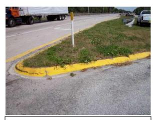
Painted curb markings are rated as symbols. Do not rate curb markings for nighttime reflectivity.
