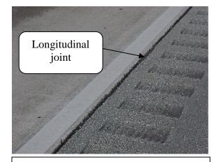
Do not rate the longitudinal joint between the rigid pavement and the asphalt shoulder if it was never sealed.
