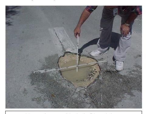
Measure the area and the depth of the pothole.
