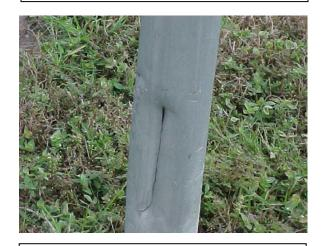
This sign column has been damaged and does not meet desired MRP standards.
