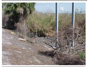
This fence has been damaged and is not the correct height. This does not meet MRP standards.
