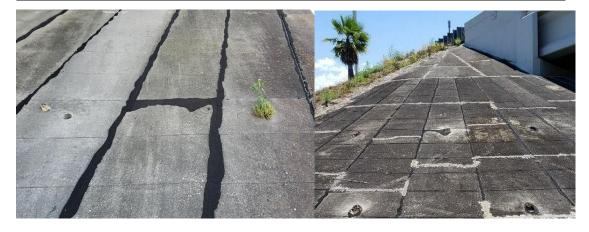
Some of these weep holes have vegetation growing out of them. If more than 10% are filled on one side of sample point, this would not meet maintenance conditions.
