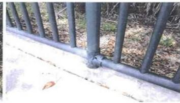
Cracked or broken hardware would not meet desired maintenance conditions.
