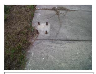
Rigid objects protruding from concrete greater than ¼ inch in height.
