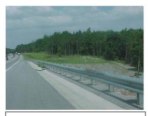
Penetrated guardrail does not meet MRP standards.
