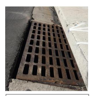
The inlet grate is not fitted into the slot correctly. This would not meet MRP standards.
