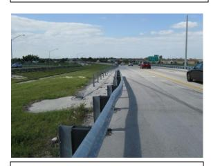
End anchor for SAFENCE behind guardrail.
