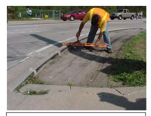
Drop-off behind curb. Since this road has curb & gutter this would be evaluated under curb & sidewalk edging.
