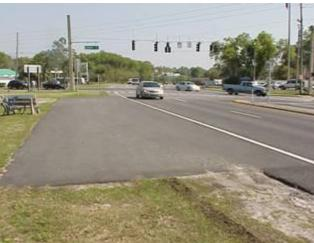
Asphalt bus turnout on rural roadway. This should be rated as roadway pavement, also rate for edge raveling. (Note: Rate only the edge of pavement parallel to the travel lanes for raveling)
