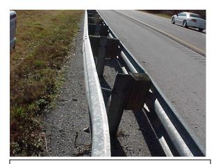
This guardrail has minor damage to the rail and a missing offset block. This would not meet MRP standards.
