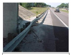
This guardrail has been damaged by a crash. Several posts are damaged. This does not meet MRP standards.
