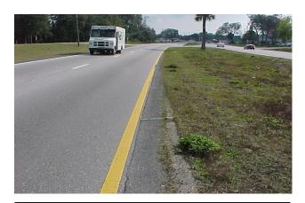
This edge widening is less than 2 feet wide therefore, does not meet MRP standards for paved shoulders (unless specified in the Straight-line Diagrams).
