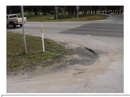
This is a rural crossover with a post mounted delineator installed. According to Standard Plans the delineator should be installed <u>6 ft.</u> from the edge of pavement to the delineator. MRP has a tolerance of <u>1 ft. 6 inches</u>. This delineator is installed <u>8 ft. 6 inches</u> from the edge of pavement. This installation does not meet MRP standards.
