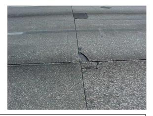
These are pictures of defects in rigid pavement. Calculate the area to determine if it is greater than <u>1/2 square foot</u> and measure the depth of the defect. If BOTH depth and area are greater than the standard limits the areas do not meet MRP standards.
