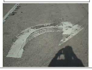
These pictures are examples of worn out symbols. If more than 10% of the cumulative symbol area or 50% or less of any one symbol is not functioning as intended then this would not meet MRP standards.
