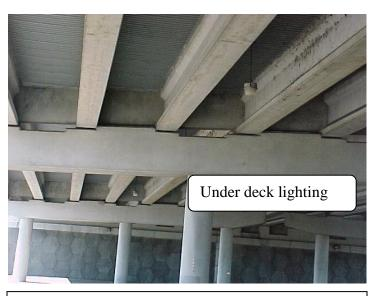
Under highway deck lighting should be included in the evaluation of lighting.
