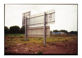
Signs installed below the fuse cut do not meet MRP standards.
