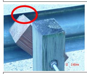
A guardrail block is considered twisted if there is a gap between the top edge of the block and the guardrail.
