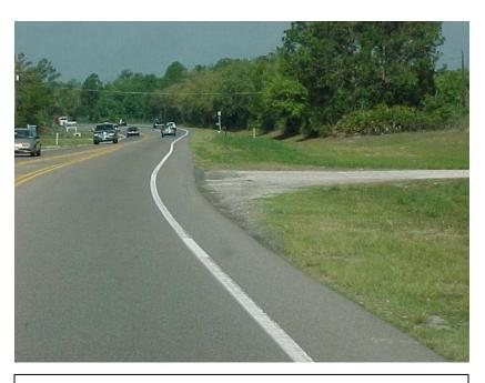
This is an example of a turnout in a paved shoulder section. This should be rated as paved shoulder only.
