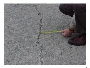
These pictures show an unsealed crack wider than 1/8 inch in rigid pavement.
