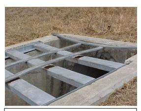
Broken welds on grate. Does not meet conditions.
