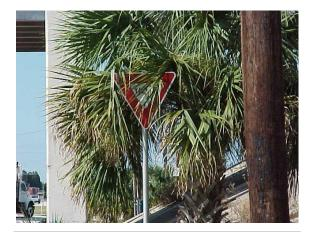
This sign is in good condition but cannot be seen because of a palm tree. The sign meets MRP standards, however tree trimming would not meet MRP standards.
