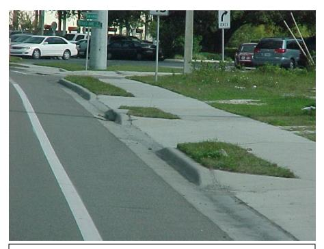
These are urban flared turnouts. The area from the back of curb to the front of the sidewalk is to be rated as turnout.
