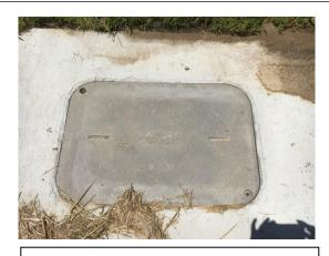
Pull box missing bolts. This would not meet conditions.
