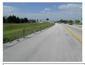
CASS Cable Safety System: C-shaped posts Installed in a sleeve driven into asphalt or set in concrete foundation. 3 cables in a slot at the Top of the post separated by plastic spacers.
