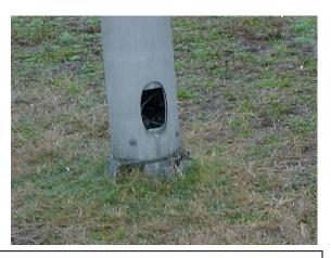
Any electrical inspection plate, access panel cover or pull box cover that is not properly secured in place will cause this characteristic not to meet the desired maintenance conditions. The light poles shown above are missing the access panel cover and, therefore, do not meet MRP standards.
