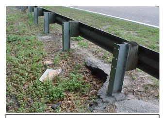
The asphalt under the guardrail has washed out. The guardrail meets desired maintenance conditions, however, unpaved shoulder or front slope would not meet MRP standards.
