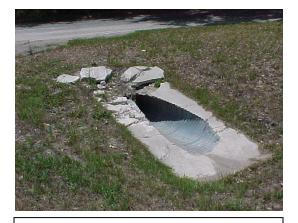
Side drain pipe with damaged concrete.
