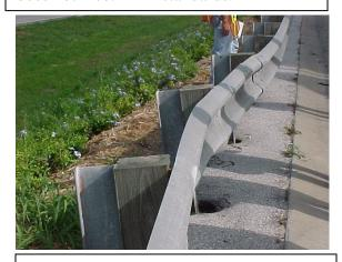
This guardrail has been hit by a vehicle. The posts have been knocked out of alignment and may not function as designed. This guardrail does not meet MRP standards.
