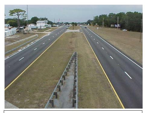
Striping on a typical four lane divided highway.
