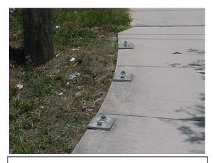
Missing handrail, this does not meet MRP standards.
