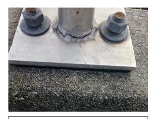
Broken welds will not meet desired maintenance conditions.
