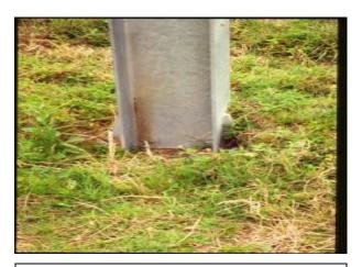
This breakaway device is covered and does not meet MRP standards.
