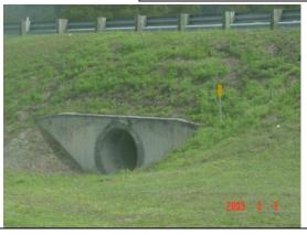
This object marker was installed but is not needed because the headwall is behind guardrail. Since the object marker is installed, it will be rated. The object marker is installed 2 feet 6 inches from the ground to the bottom of the marker. It should be installed no less than 4 feet plus or minus 1 foot from the ground to the bottom of the marker. This marker does not meet MRP standards.
