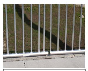
Picket railing missing steel sleeve at expansion joint. This does not meet MRP standards.
