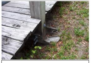
Deterioration of supports.
