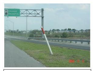
This object marker is for fiber optic cable. It would not be rated since this is not a Department maintained object.
