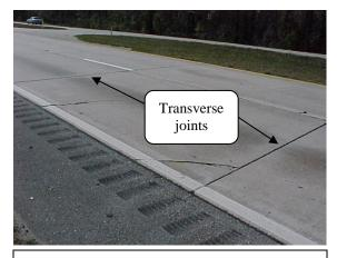
This picture shows two traverse joints and a slab that has two unsealed cracks.
