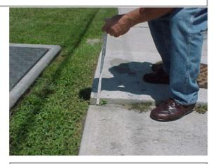
Any single vertical misalignment measured greater than  $\frac{1}{2}$  inch would not meet desired maintenance conditions.
