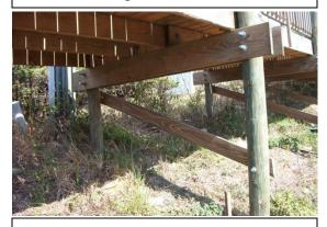
Support piling / post with bracing.
