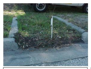
Soil buildup in a miscellaneous drainage structure. This does not meet MRP standards for miscellaneous drainage.
