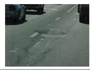
These are pictures of shoving. Measure the length and width to determine the shoving area. If the shoving area is more than 25 cumulative square feet, then this would not meet conditions for shoving.
