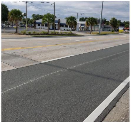
These areas should be rated for rigid and flexible pavement.
