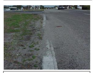
Edge line obscured by soil or other debris does not meet MRP standards
