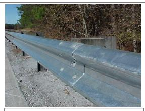
This guardrail section is lapped incorrectly. If hit by a vehicle, the rail would not function as designed. This does not meet MRP standards.
