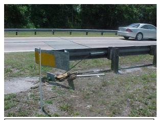
Damaged guardrail end section. This site does not meet MRP standards.
