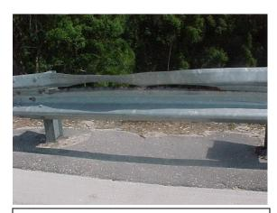
This guardrail section has been penetrated due to a crash. This does not meet MRP standards.
