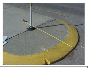
Post mounted delineators are installed according to the Standard Plans. The index shows the edge of pavement as the standard reference point. If curb and gutter is present measure from the top face of curb. At a curb without a gutter or traffic separator, the face is the edge of pavement (picture on right).
