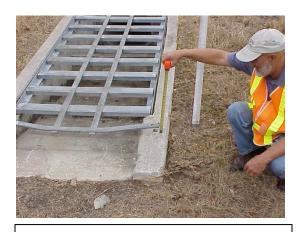
Broken bolt, grate bent. Does not meet conditions.
