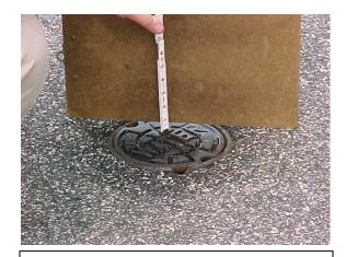
Depression at a water valve in pavement.
