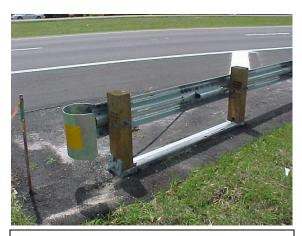
This is an approach end guardrail end section. Check to make sure all connecting hardware is in place.
