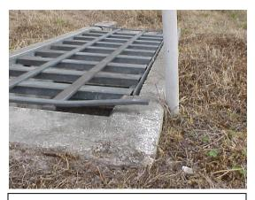
Broken/missing bolts, grate bent. Does not meet conditions.
