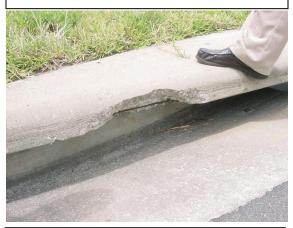
Exposed steel in this curb inlet. This does not meet MRP standards for inlets.
