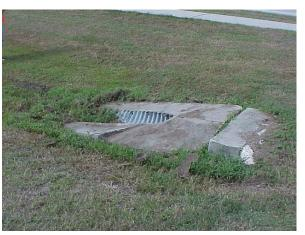
Side drain pipe with 3 or more cracks  $> \frac{1}{2}$  in. wide 1 ft. in length. This does not meet MRP standards.
