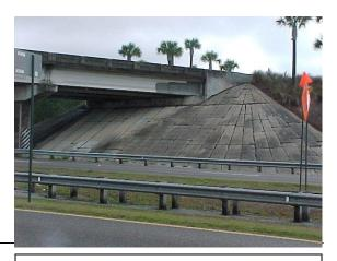
This is an example of concrete slope pavement.
