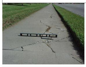
Sidewalk cracking. Measure each horizontal crack greater than ½ inch wide. For MRP purposes, each linear foot of horizontal crack greater than ½ inch equals 1 sq. ft. of crack area.
