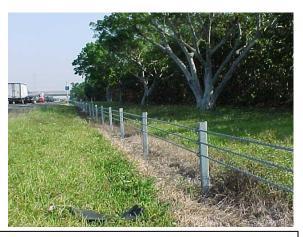
GIBRALTAR Post installation similar to the CASS and SAFENCE. 3 cables are placed in molded "hairpin" slots or J bolts installed along the sides of the posts.
