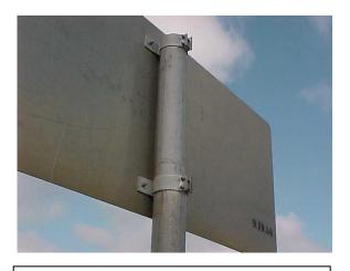
This sign was installed using "C clamps and does not meet MRP standards.
