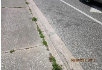
Area may not meet maintenance conditions if more than 7-1/2 square feet of unwanted vegetation for any 50 square foot area of curb/asphalt joint and curb/sidewalk joint.
