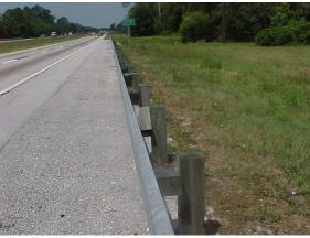
For MRP purpose, evaluate asphalt from edge of travel lane to face of guardrail as paved shoulder.
