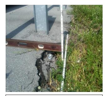
The asphalt is broken with a deviation greater than <u>5 inches</u> and would not meet desired maintenance conditions for unpaved shoulder
