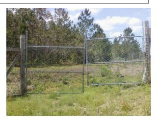
Misaligned gates, measure opening to ensure it is not greater than 6 inches.
