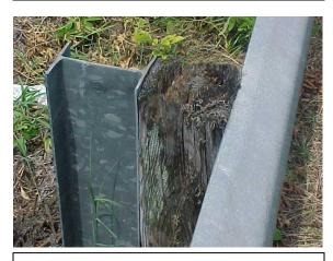
This is a rotten and deteriorated guardrail offset block. It does not meet MRP standards if more than 10% of the blocks are rotten and deteriorated.
