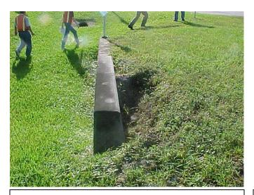
This is a washout in front of a headwall greater than 6 inches in depth. This would not meet MRP standards.
