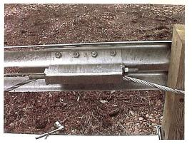
Insert the 6' 6" cable "AP22" into the anchor box (plate) as shown.
