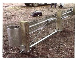
Attach the buffer end with (4) splice bolts and nuts.
