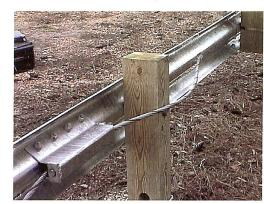
Attach the double cable anchor box (plate) to the rail, and connect the cable using the 1" Nut & Washer.
