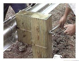
At each post requiring a blockout, use a 5/8" x 18" Bolt "HW231B", with 5/8" Nut and Washer
