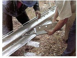
Insert the cable into and through the standard anchor box (plate) "AP32".
