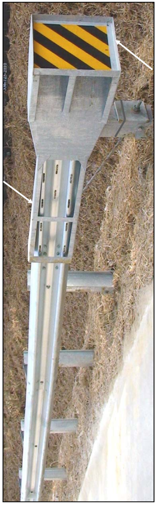
Impact Head Feeder Guide Chute
