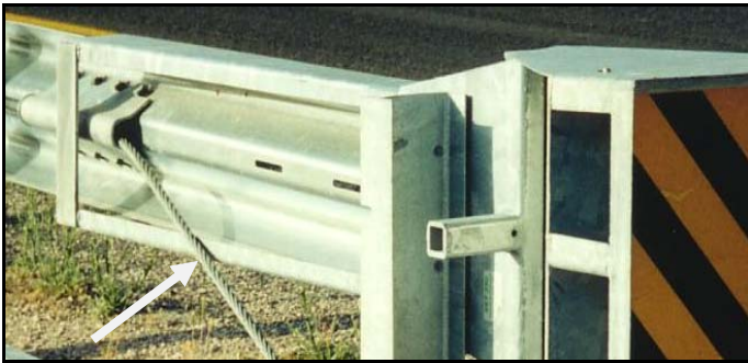
SKT-SP-MGS cable is fed inside through the feeder chute. The SKT feeder chute is longer than the FLEAT
