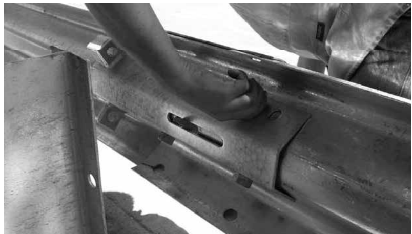
Figure 7. Splice rail 3 to rail 4 with 8 standard splice bolts.
