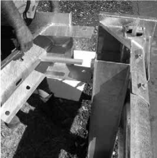
Figure 35. Fit secondary head to main head.
