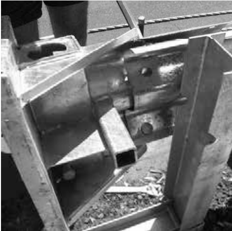
Figure 17. Attach Impact Head to rail 1.
