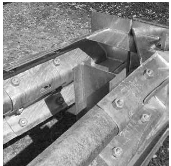
Figure 46. Use 8 standard splice bolts.
