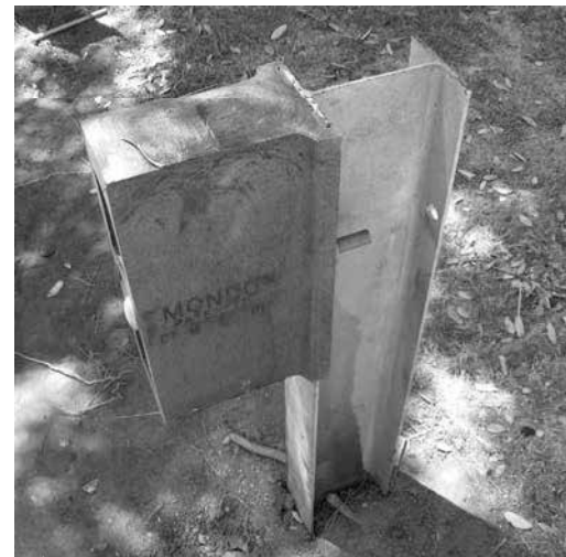
Figure 3. Bolt the blockout prior to attaching the rail.
