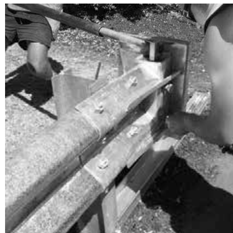
Figure 24. Use socket to lock bar in the turned position.
