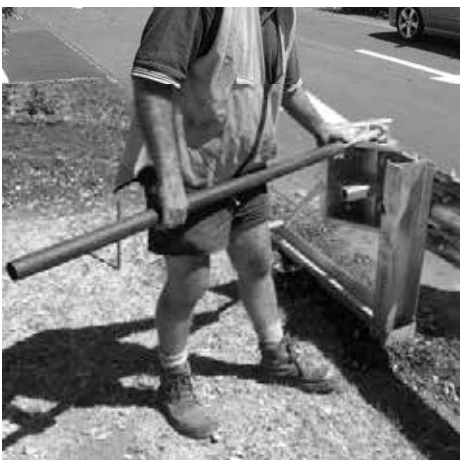
Figure 23. Use crow bar to turn Friction Plate.
