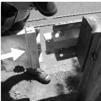
Figure 14. Push Slider Panel over rail 2.
