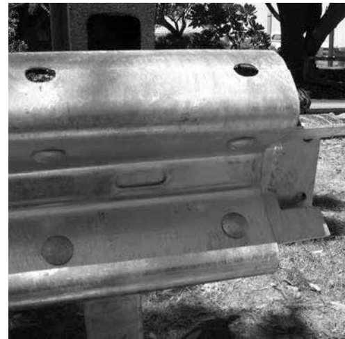
Figure 11. Remove angle bar bolts.
