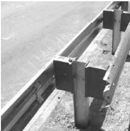
Figure 33. Essentially a tangent system installed parallel to median barrier.
