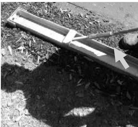
Figure 19. Push cables under steel strap on Ground Strut.
