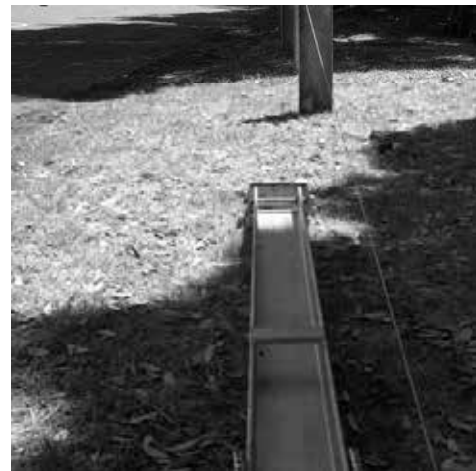
Figure 31. Place Ground Strut parallel to string line.
