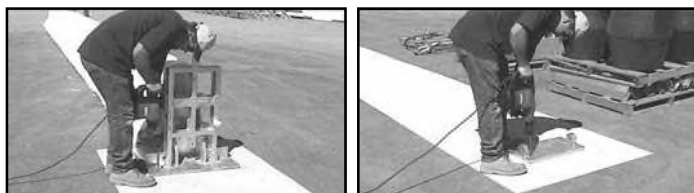
Drill the anchor bolt holes to the proper size and depth
