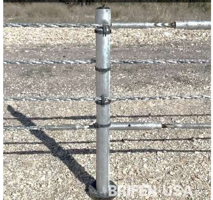
Rigging screws can be located at post
