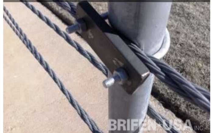
U-bolt used as a temporary clamp
