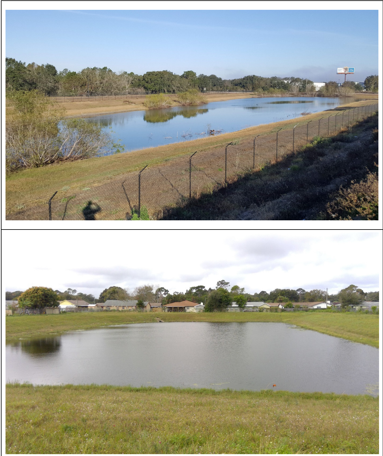
Figure 4-7. Typical Wet Detention Ponds in Good Condition Return to List of Figures
