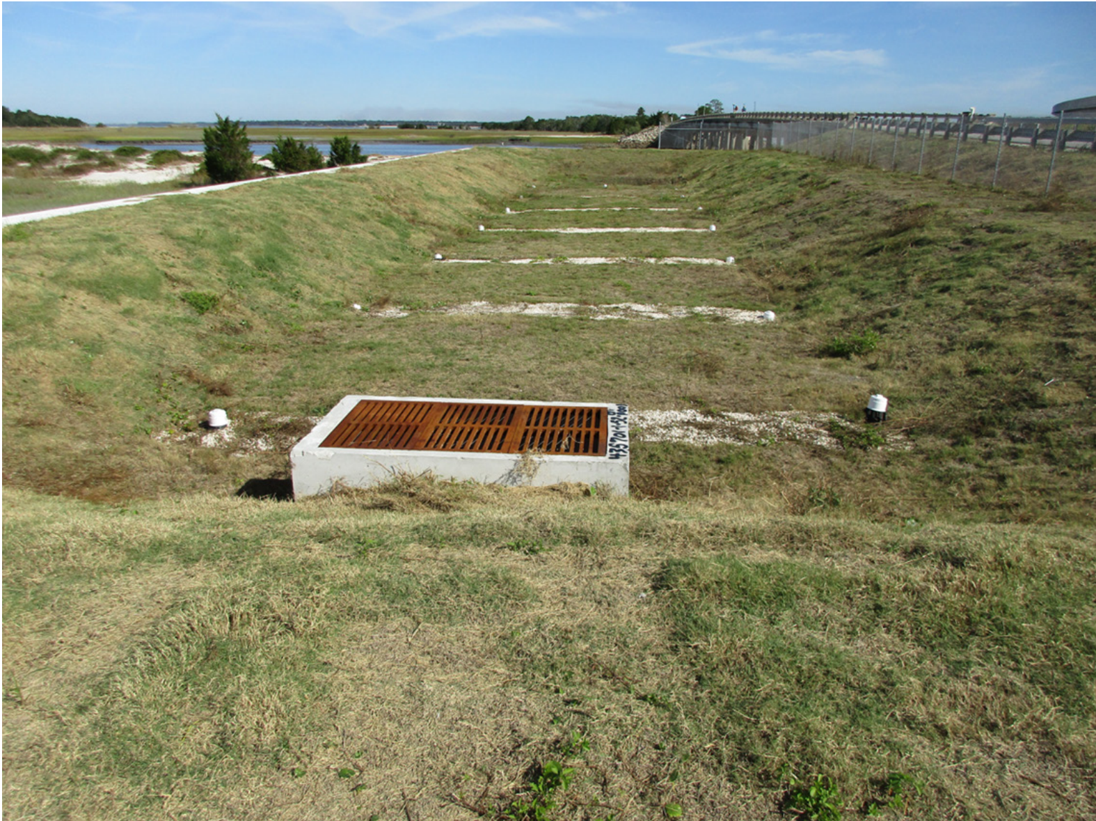
Figure 4-18. Typical Dry Detention Pond with Filtration in Good Condition Return to List of Figures
