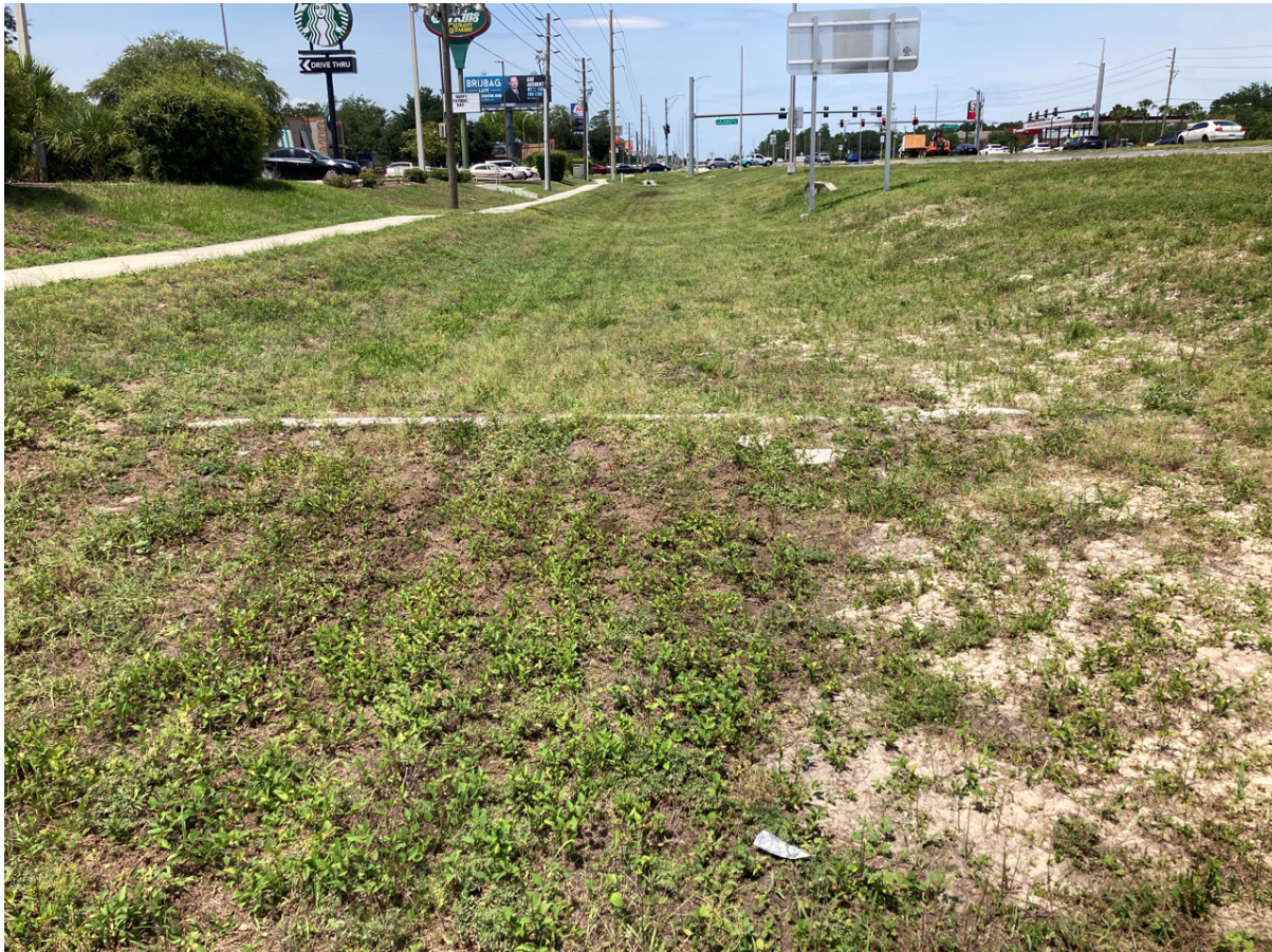
PHOTO 27 LOOKING AT DB-8 STA 431+60 LT (LINTEL DAMAGED).JPG
