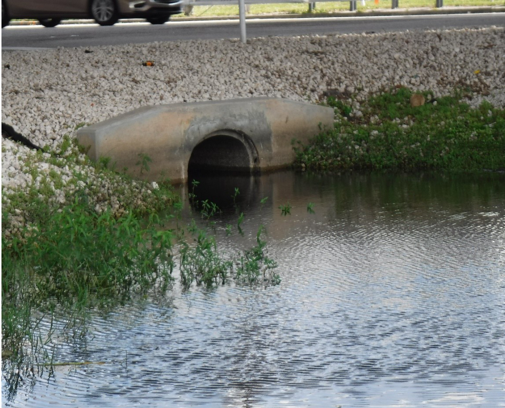
Figure 4-40. Typical Closed Conveyance Outfall in Good Condition Return to List of Figures
