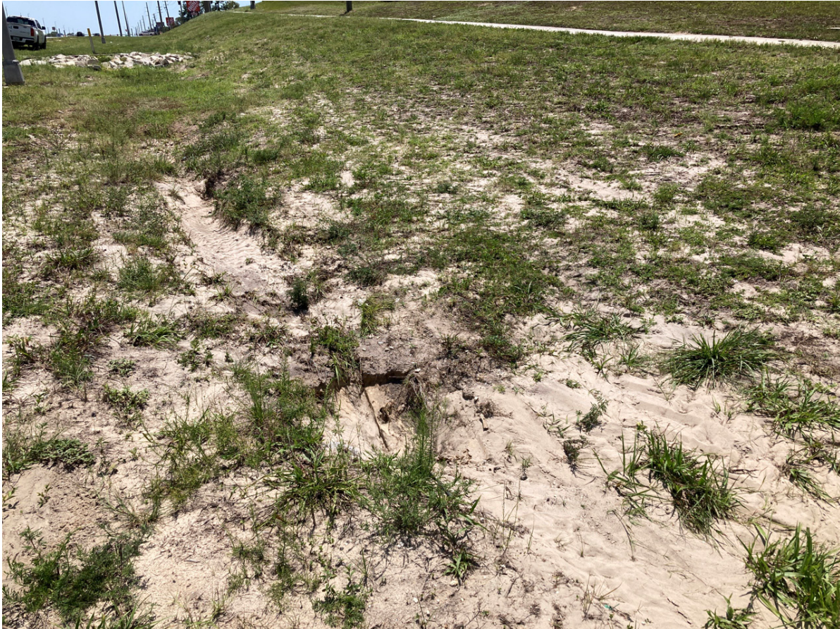
PHOTO 19 LOOKING AT EROSIONAL AREA NORTH OF DB-13.JPG
