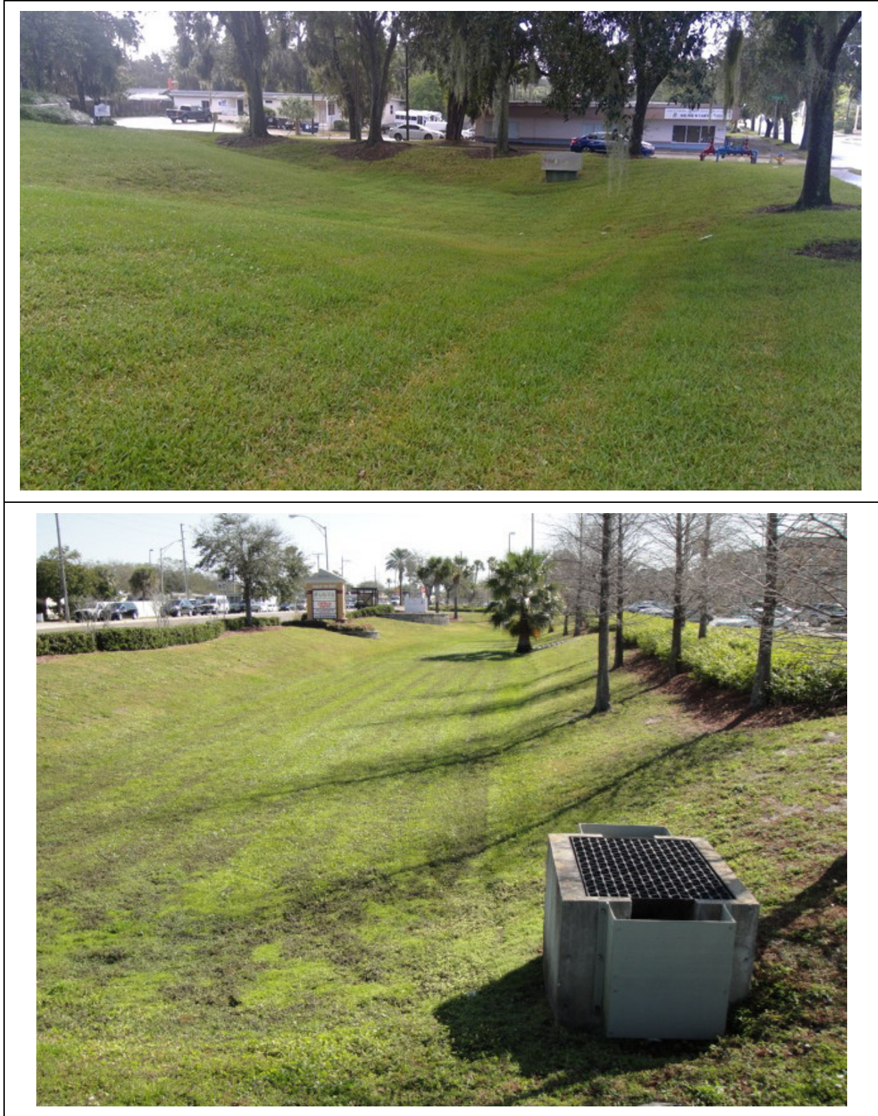
Figure 4-12. Typical Dry Detention Ponds without Filtration in Good Condition
