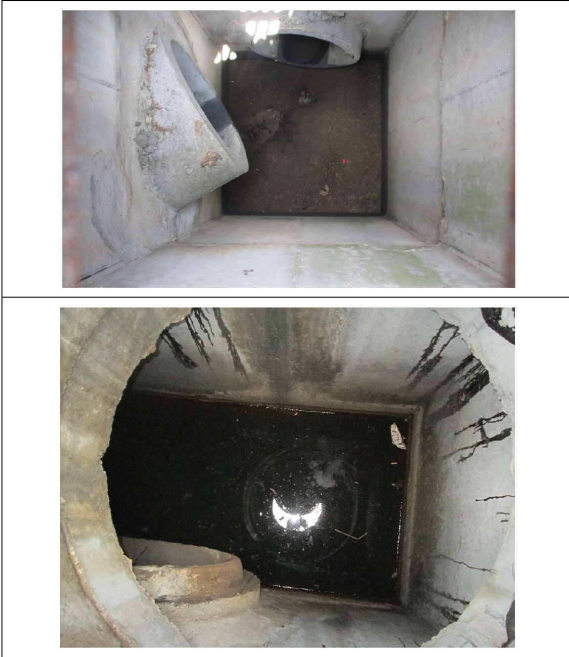
Figure 4-34. Typical Horizontal Exfiltration System Control Structures in Good Condition
