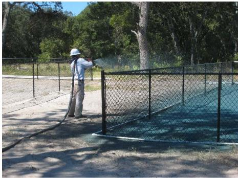
Figure 8. Hydroseeding common bermudagrass.
