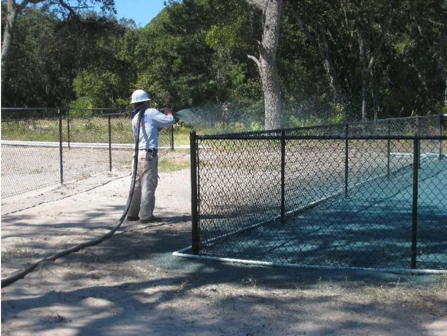
Figure 8. Hydroseeding common bermudagrass.
