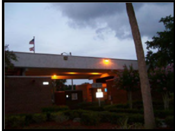
Example of building light not working. The lights under the roof will be included as foyer lighting.
