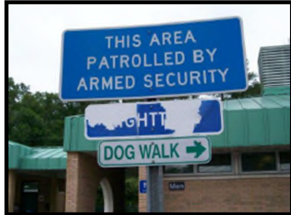
This sign is peeling and would not meet the desired maintenance conditions.
