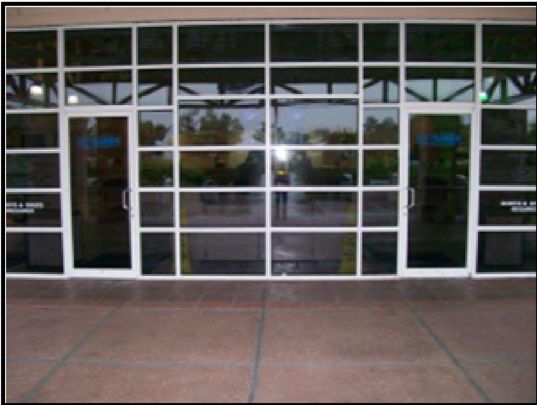
Clean windows meet desired maintenance conditions.
