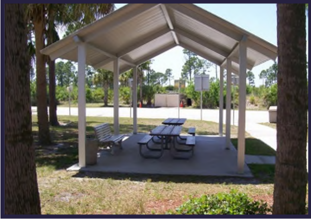
Inspect slab, shelter, table, and the area adjacent to the shelter.
