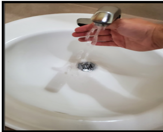
This sink is properly functioning and appears to meet maintenance conditions.
