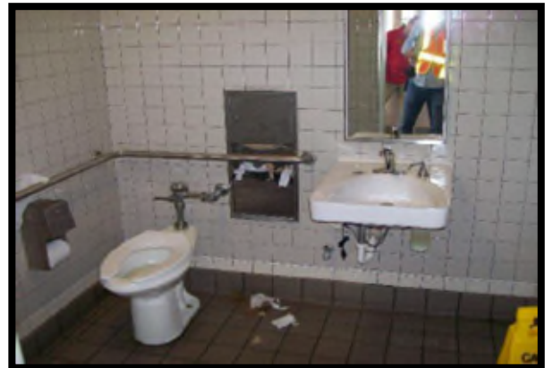
Example of a trash receptacle that is full and would not meet maintenance conditions.
