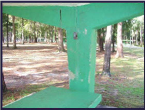
Exposed wires in conduit box would not meet desired maintenance conditions.
