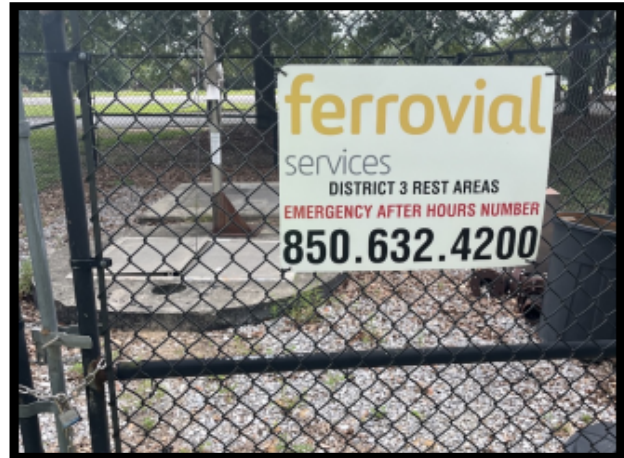
Wastewater treatment facility with signs in place. If information on sign is current, this would meet desired maintenance conditions.
