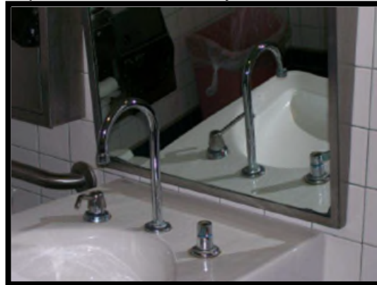
This sink appears to meet desired maintenance conditions.
