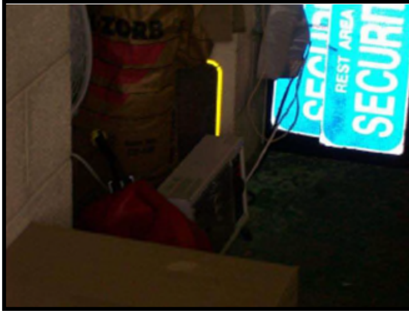
Gas can and electrical heater are stored together in the utility area; this would not meet desired maintenance conditions.
