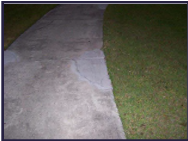
Sidewalk repaired. This meets desired maintenance conditions.
