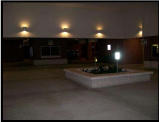
Example of lighting in foyer area.
