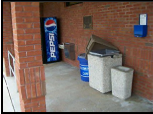
The receptacle lid is not secured; this would not meet desired maintenance
