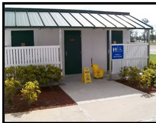
Example of a family restroom with equipment not stored in its proper place. This would not meet the desired maintenance conditions.
