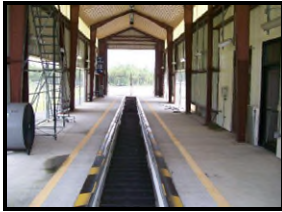
Clean orderly inspection bay and pit.
