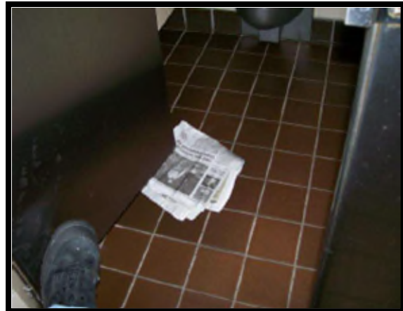
Trash and debris on floor may create a trip hazard and would not meet desired maintenance conditions.
