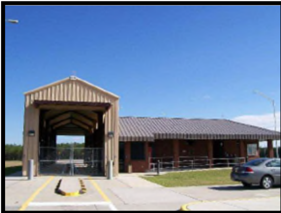
Inspection barn at a truck comfort station.
