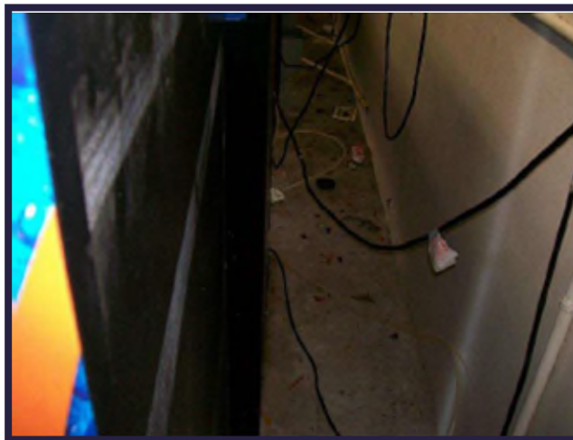
Behind the vending machines should be clean. This does not meet desired maintenance conditions.
