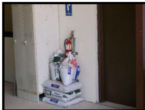
Materials stacked in front of fire extinguisher would not meet desired maintenance conditions.
