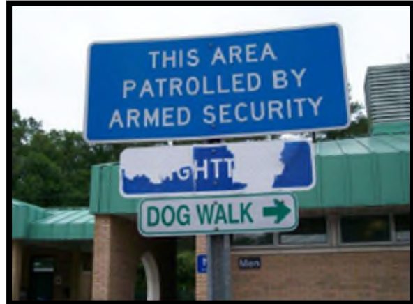
This sign is peeling and would not meet the desired maintenance conditions.
