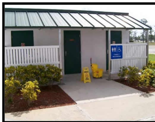
Example of a family restroom with equipment not stored in its proper place. This would not meet the desired maintenance conditions.
