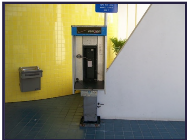
Example of phone that has been removed in an unacceptable method. This example would not meet the desired maintenance conditions.
