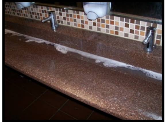
The water is not draining properly and would not meet desired maintenance conditions.
