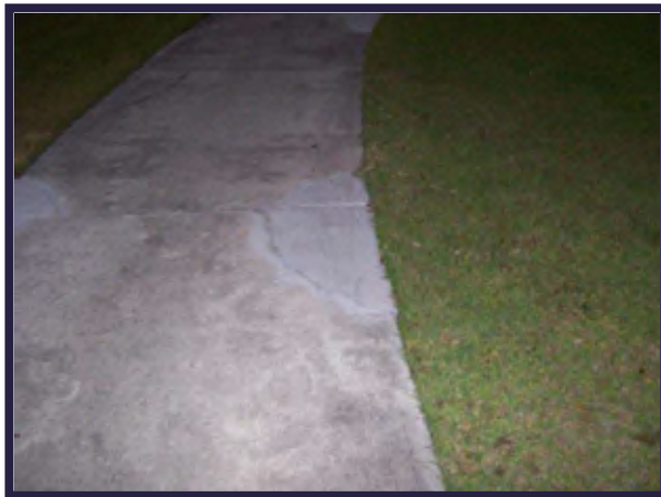
Sidewalk repaired. This meets desired maintenance conditions.
