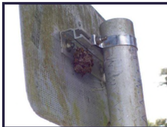
Example of wasp nest. If wasps are present this would be considered active and would not meet the desired maintenance conditions.
