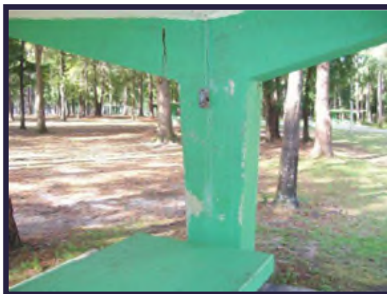
Exposed wires in conduit box would not meet desired maintenance conditions.
