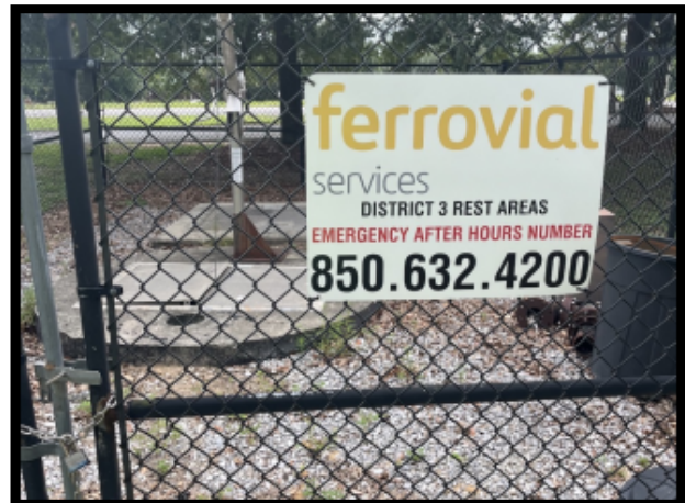
Wastewater treatment facility with signs in place. If information on sign is current, this would meet desired maintenance conditions.
