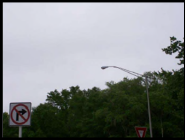
This light is not working. Count the total number of highway lights in the facility to determine if it is more than 90%.
