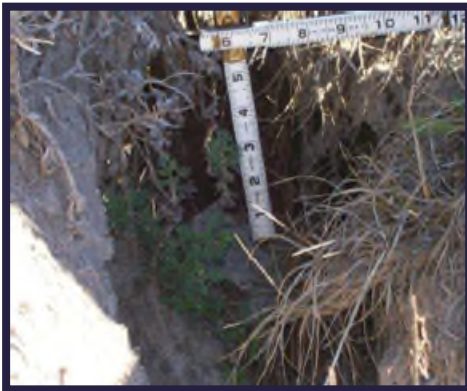
Large hole six (6) inches deep in the common and picnic area grounds this would not meet the desired maintenance conditions.
