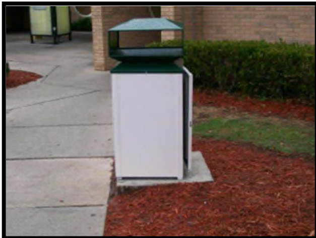
Access door not secured; this would not meet desired maintenance conditions.
