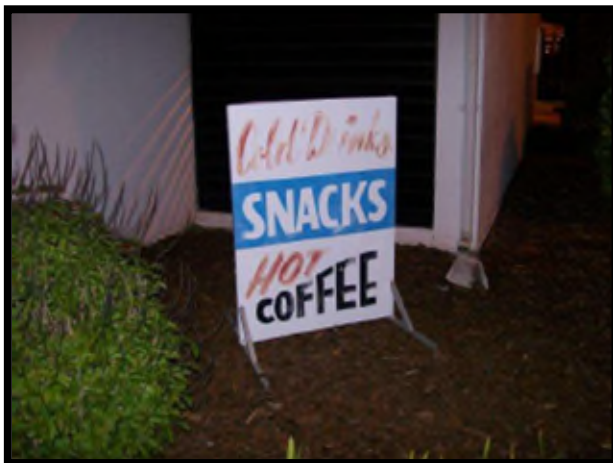
The sheathing with the message is delaminating and would not meet desired maintenance conditions.
