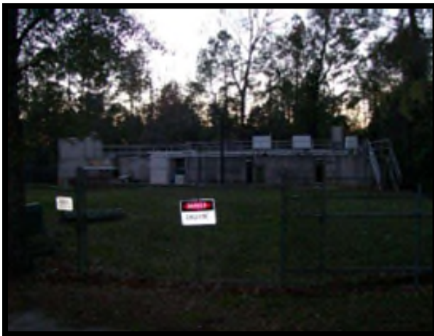
Photo of wastewater treatment facility that appears to meet desired maintenance conditions.
