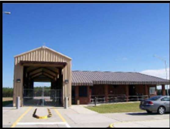
Inspection barn at a truck comfort station.
