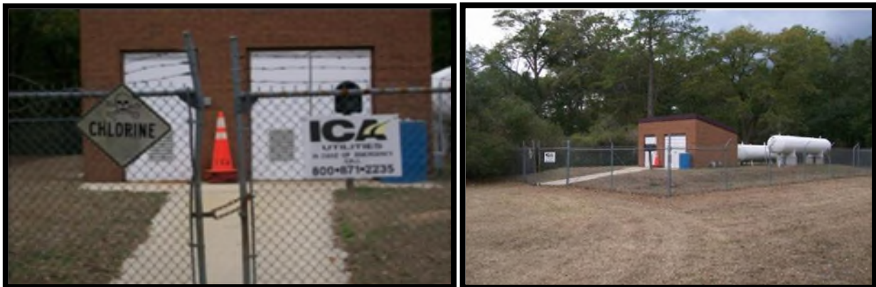
Examples of water treatment facilities with signs in place and secured, meeting the desired maintenance conditions.
