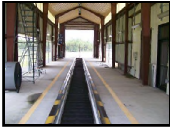
Clean orderly inspection bay and pit.
