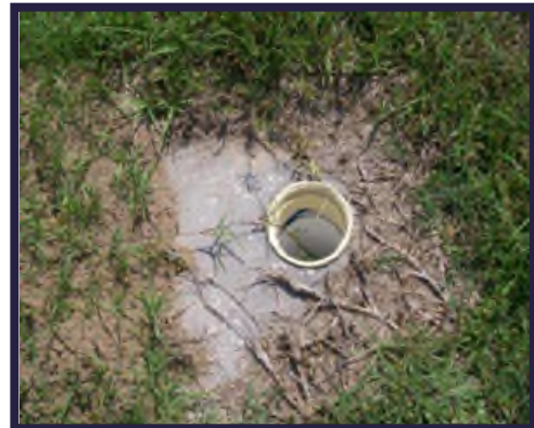
Missing valve cover in the common area this would not meet the desired maintenance conditions.
