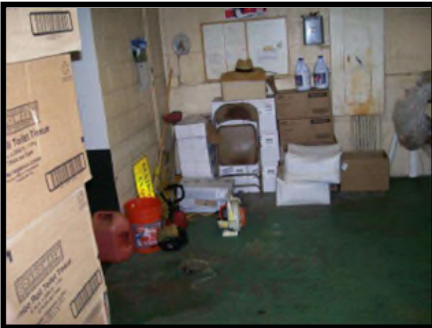
Gas can and gas equipment should not be stored in main building. This would not meet desired maintenance conditions.
