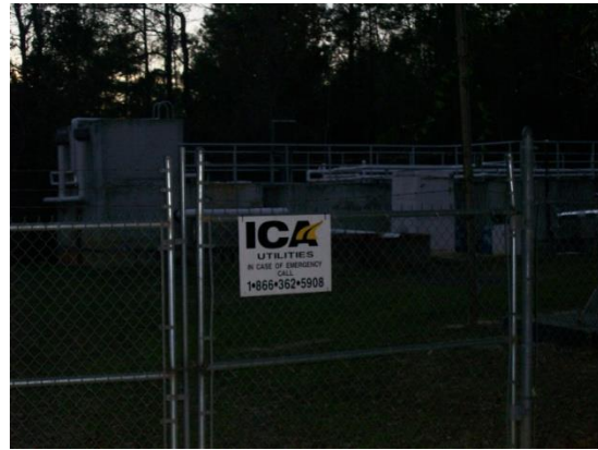
Waste water treatment facility with signs in place, this would meet desired maintenance conditions.
