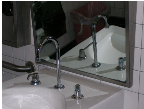
This sink appears to meet conditions.
