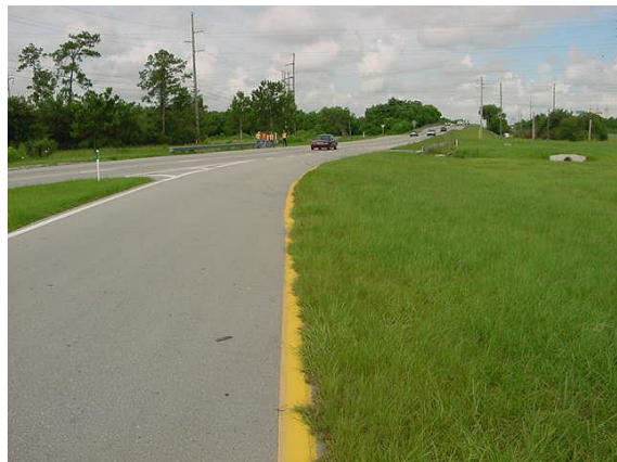
Example of edge line covered with grass, if the striping covered in grass is more than 52 continuous feet in length and not the proper width 5.6 inches?; this would not meet desired maintenance conditions.
