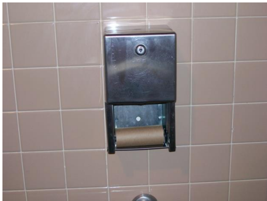
This dispenser is out of paper and would not meet desired maintenance conditions.
