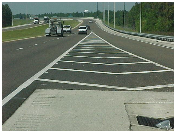
Example of symbol on roadway / ramp areas.
