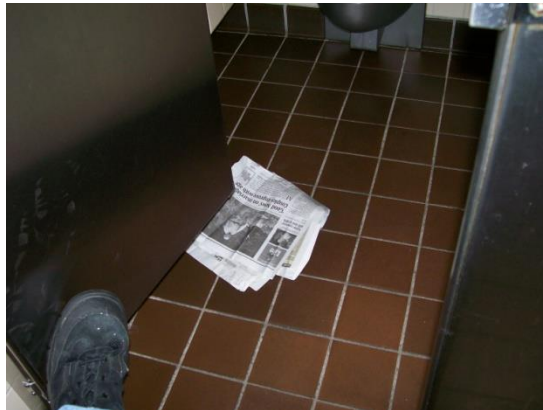
Trash and debris on floor may create a tripping hazard and would not meet desired maintenance conditions.
