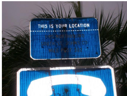
This sign would not meet the desired maintenance conditions.
