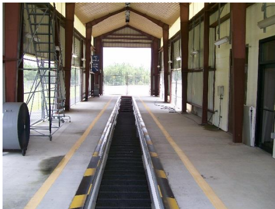
Clean orderly inspection bay and pit.
