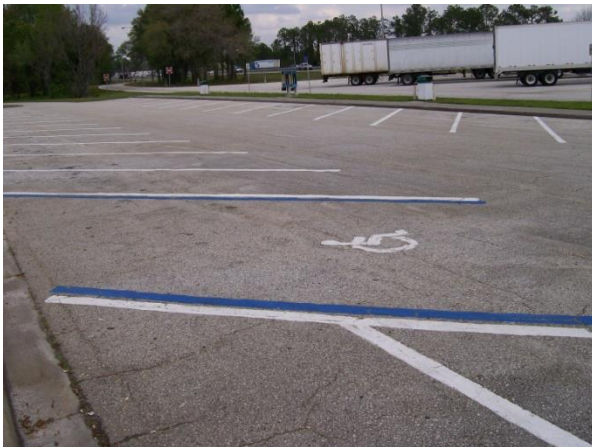
Example of striping in parking area.
