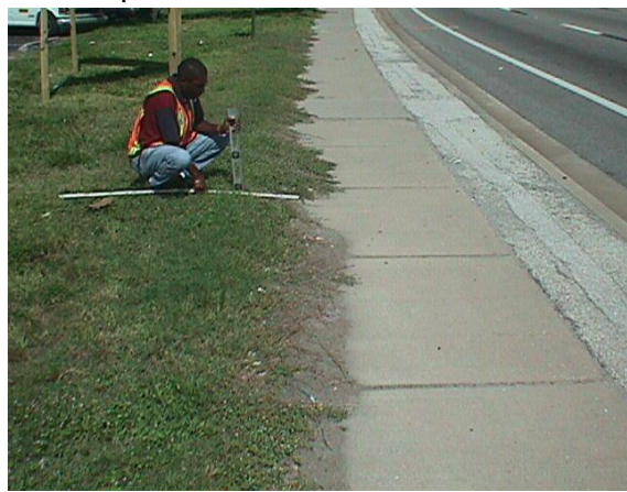
Encroachment is greater than 6 inches from the edge of sidewalk.
