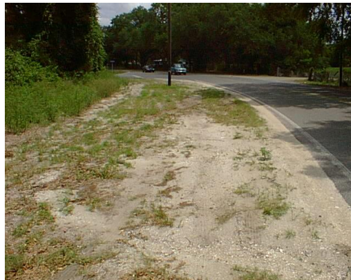
Example of more than 5 square feet of bare ground, this would not meet desired maintenance conditions.
