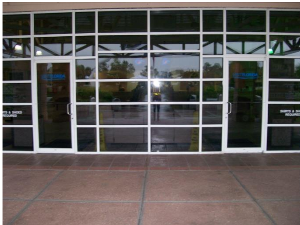
Clean windows in good working order.
