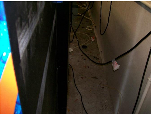
Behind vending machines should also be cleaned.
