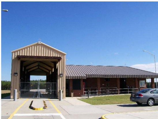
Inspection Barn at Truck Comfort Station.
