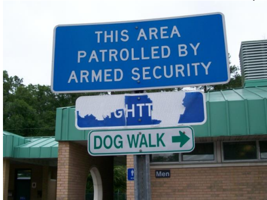
The sheathing with the message is delaminating and would not meet desired maintenance conditions.
