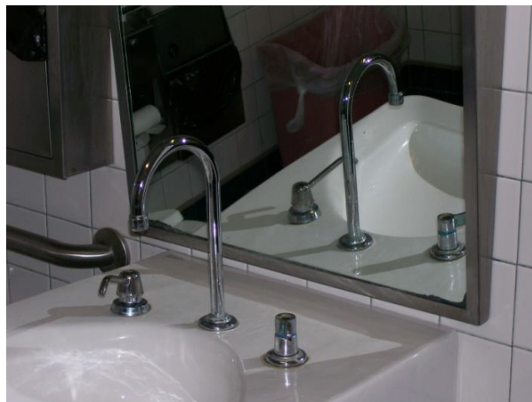
This sink appears to meet conditions.
