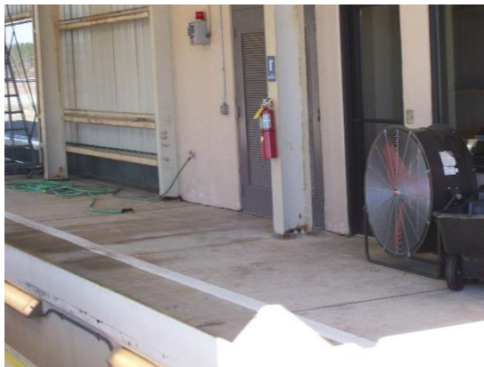
Hose on floor of inspection bay would not meet desired maintenance conditions.
