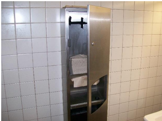
Cabinet door should be secured and function as intended, this would not meet desired maintenance conditions.
