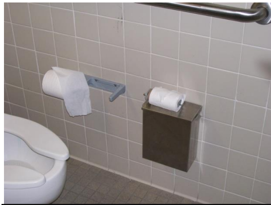
This dispenser is not in working order and would not meet desired maintenance conditions.
