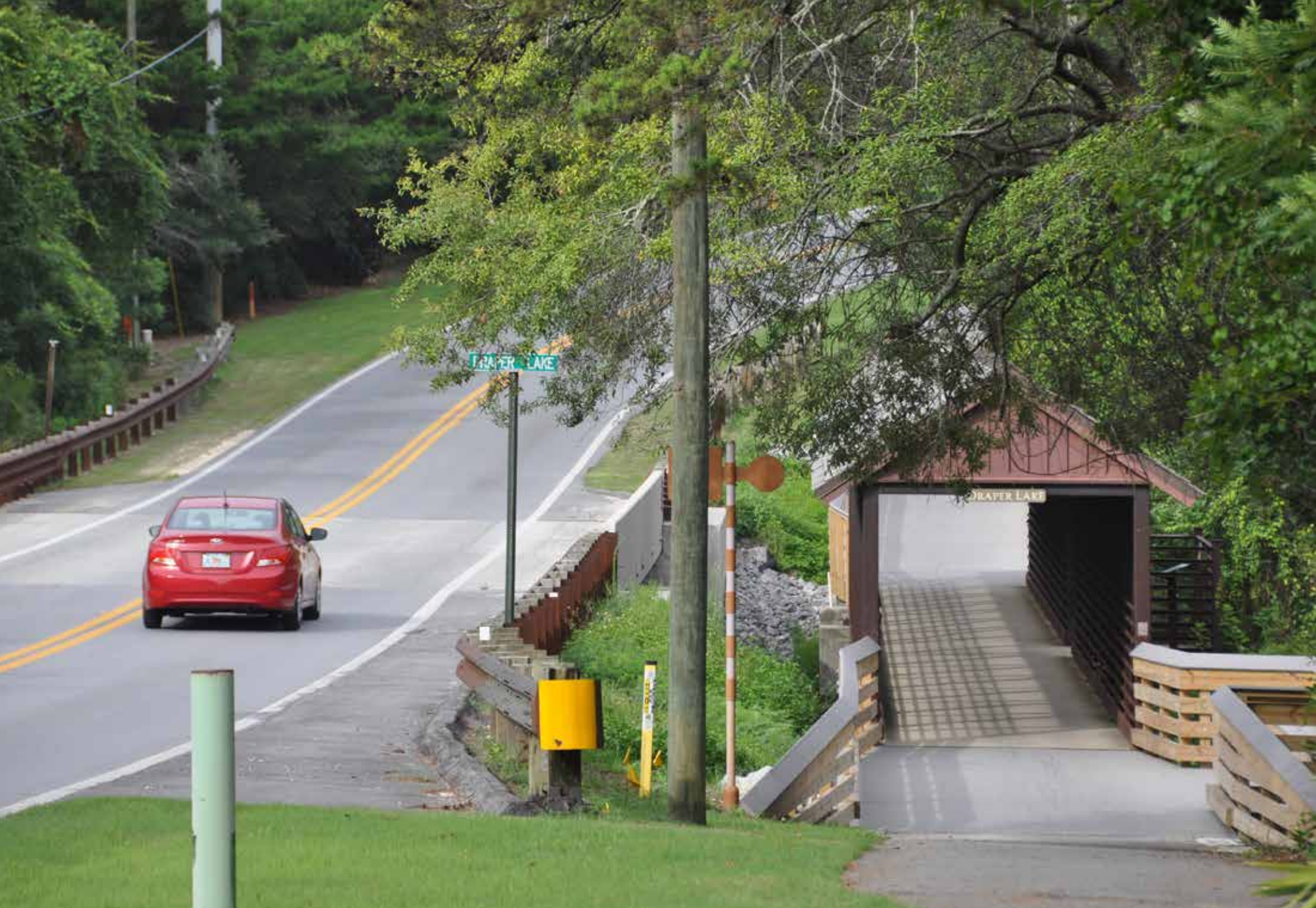
Scenic Highway 30A by FDOT
