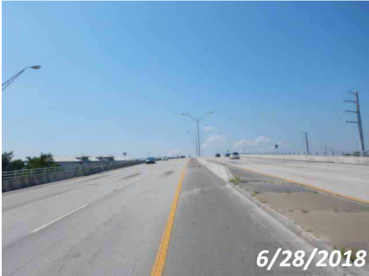
North Approach Looking South
