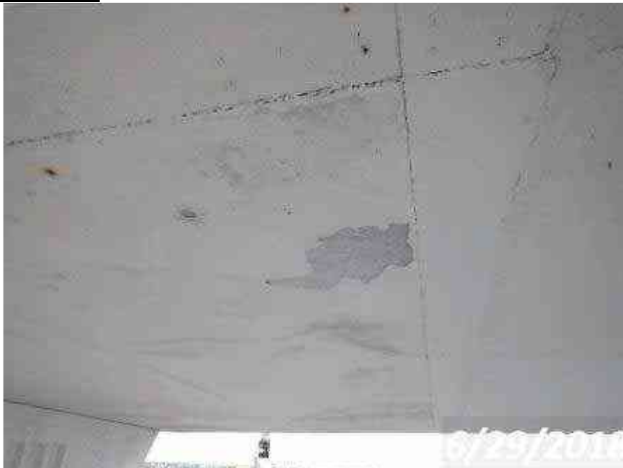
Photo 104-S07 (Unit 0: Pre Clsd Box Girder)
