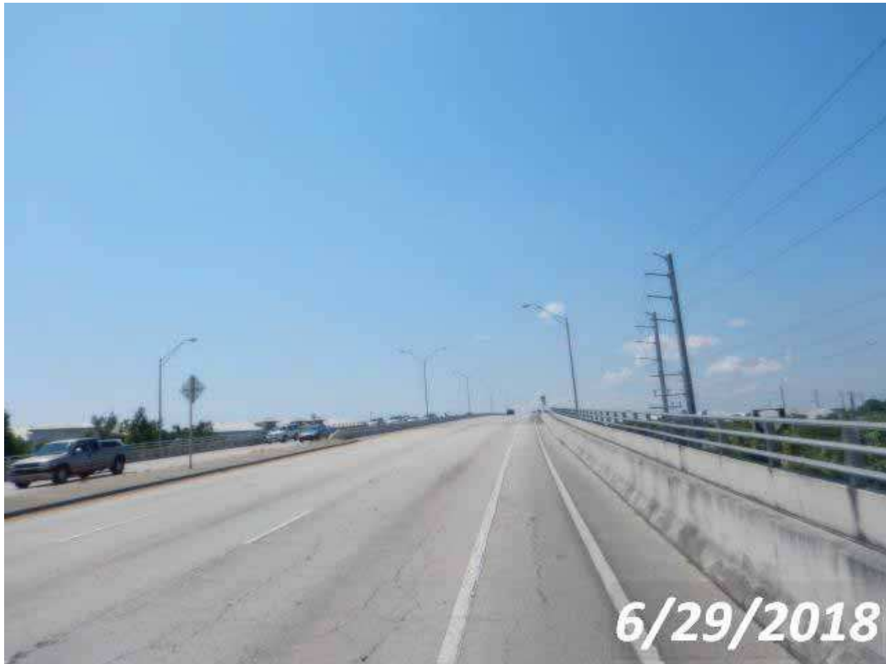
North Approach Looking South
