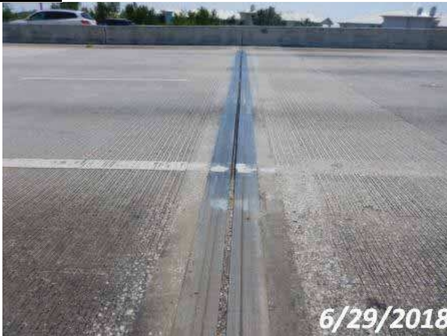
Photo 300-S01 (Unit 0: Strip Seal Exp Joint)
