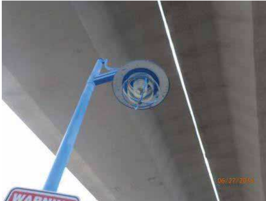
Inspection Notes Photo 3
