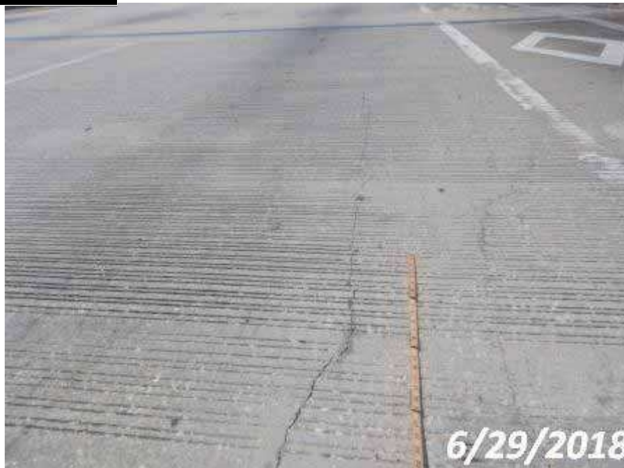
Photo 321-S01 (Unit 0: Re Conc Approach Slab)
