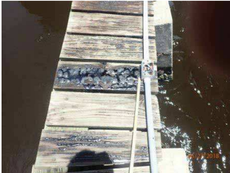
Photo 8387-U01 (Unit 0: PS Fender/Dolphin)
