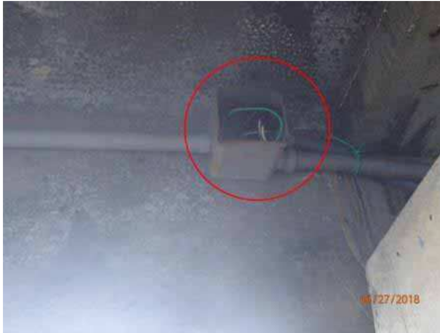
Inspection Notes Photo 5
