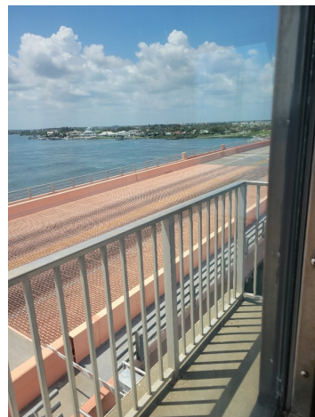
New Smyrna Beach Bridge and the tender box
