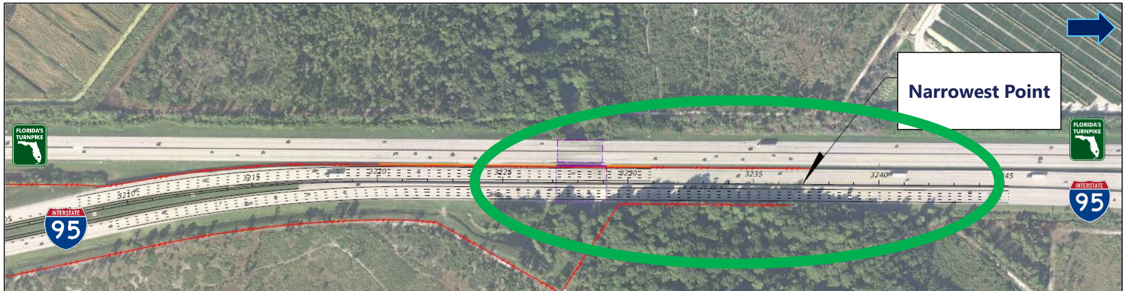
I-95 north of Indiantown Road Interchange
