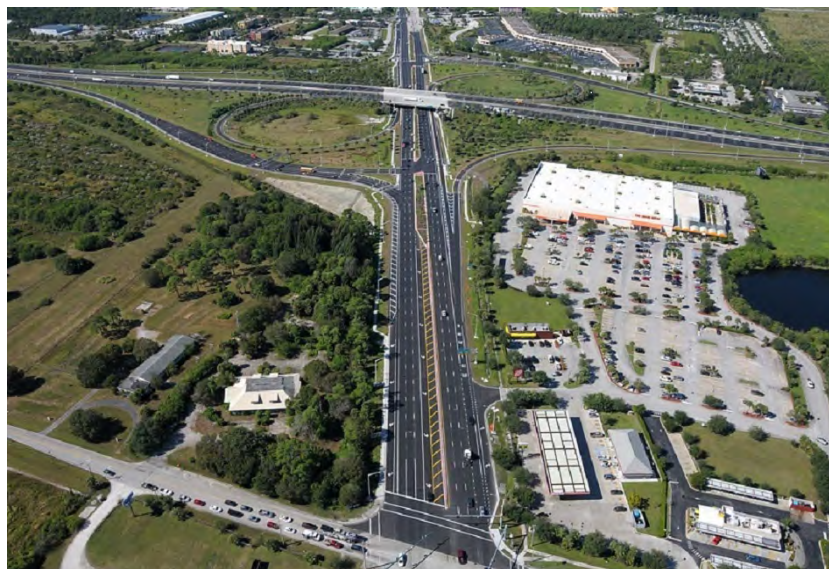
Exhibit 3: SR-70 at I-95 Interchange (facing west), St. Lucie County
