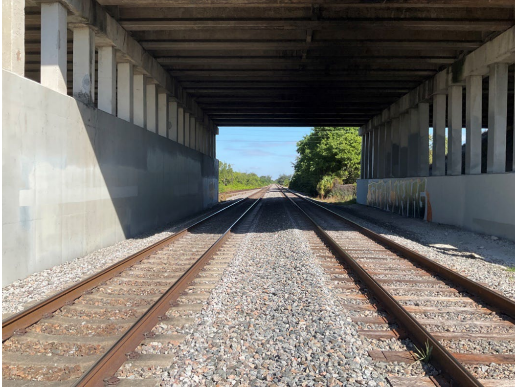
Figure 40. Photograph of 8BD04649-1, facing north.
