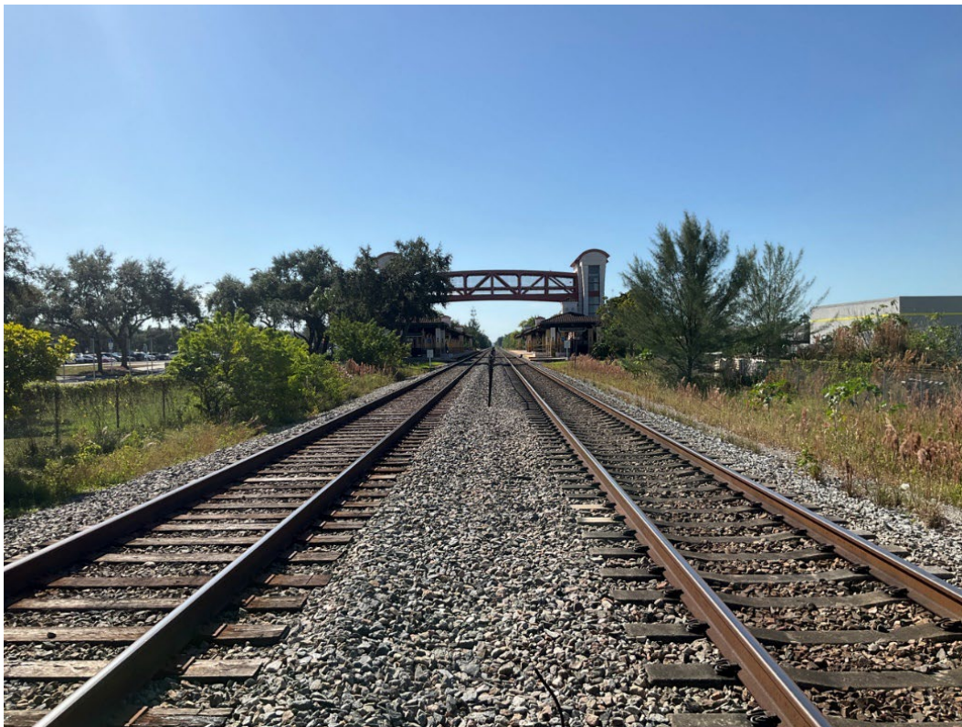
Figure 41. Photograph of 8BD04649-2, facing south.
