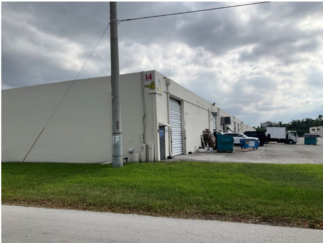
Figure 58. Photograph of 8BD09441-4, facing southeast.
