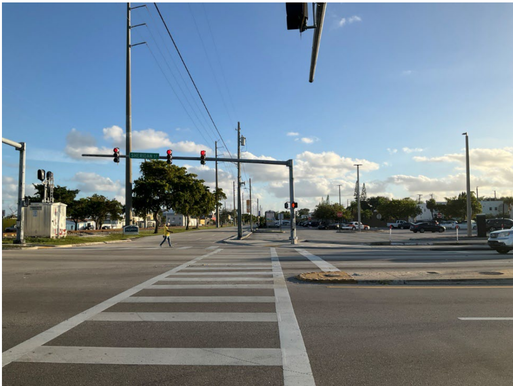
Figure 45. Photograph of 8BD04227-2, facing south.
