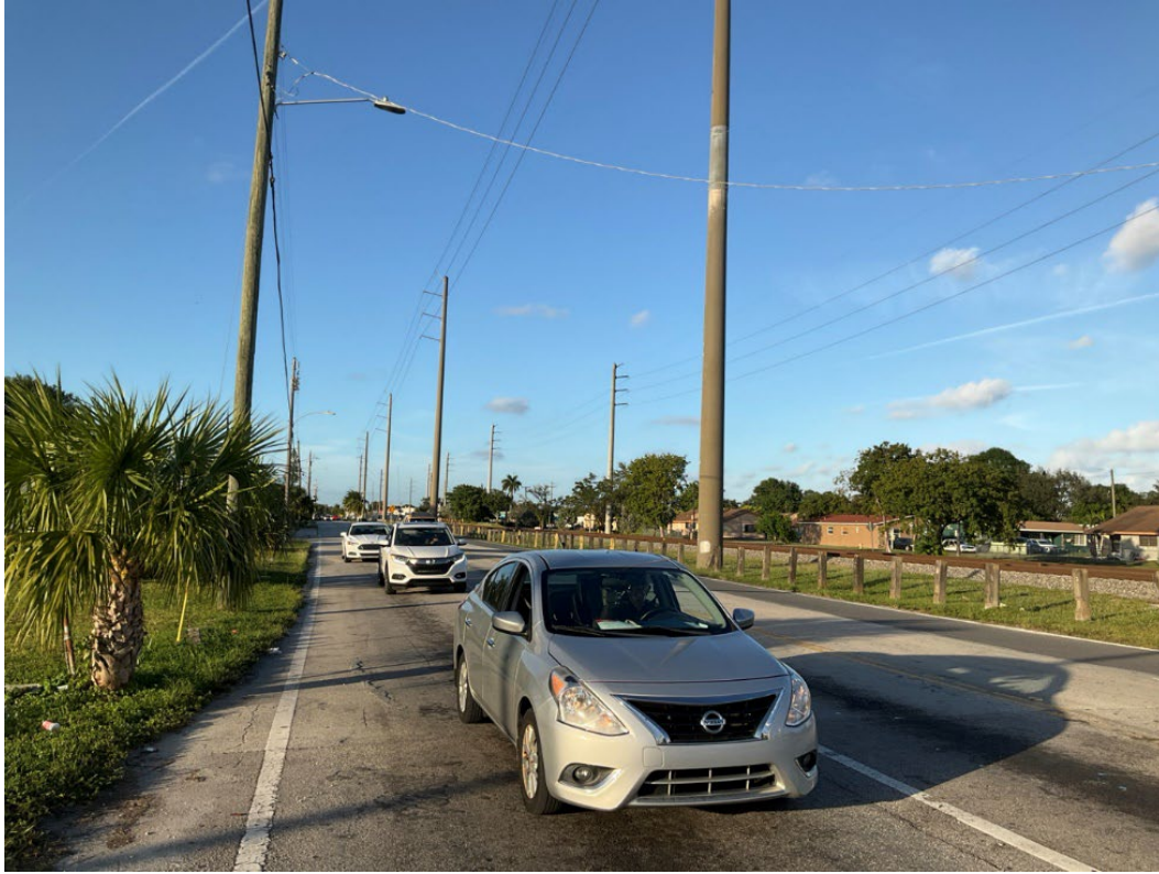
Figure 44. Photograph of 8BD04227-1, facing north.
