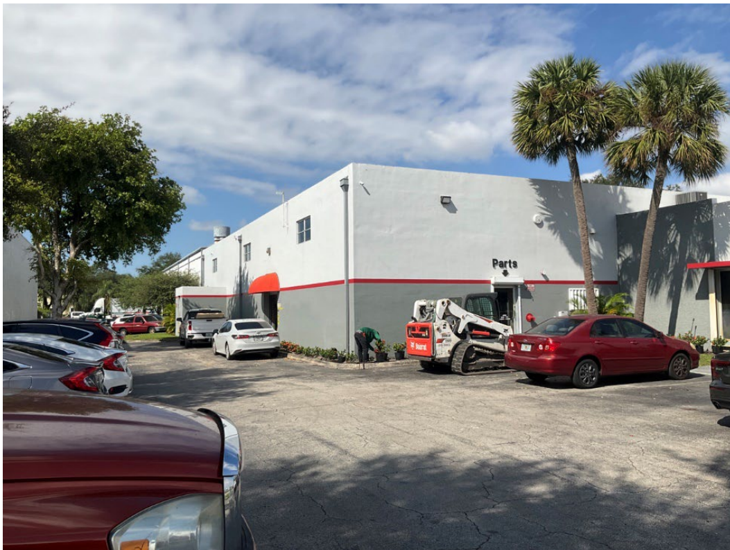
Figure 73. Photograph of 8BD09444-3, facing northwest.
