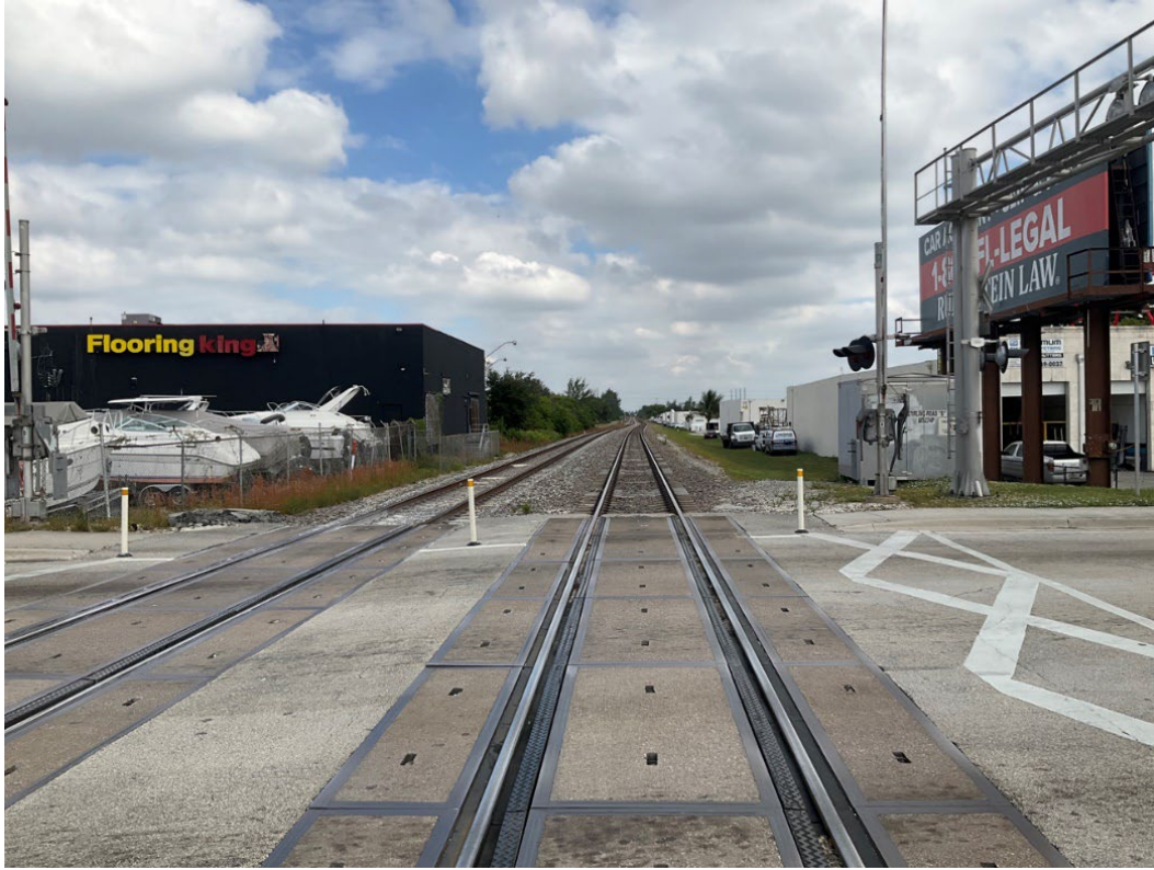
Figure 42. Photograph of 8BD04649-3, facing north.
