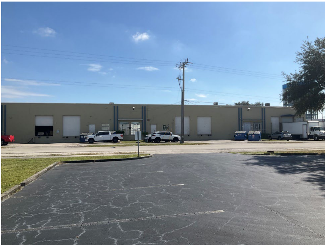
Figure 69. Photograph of 8BD09443-4, facing south.
