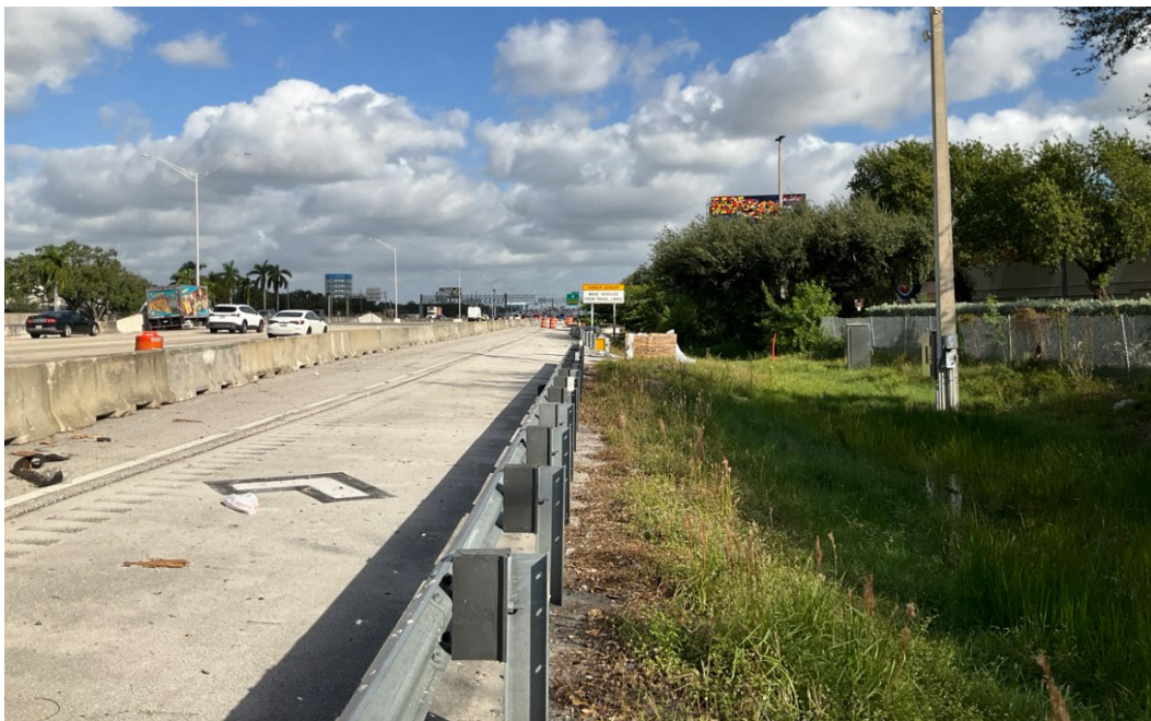
Figure 23. Overview of the APE along S.R. 9/I-95 facing north. Note drainage ditch and subsurface utilities along I-95 in right of frame.
