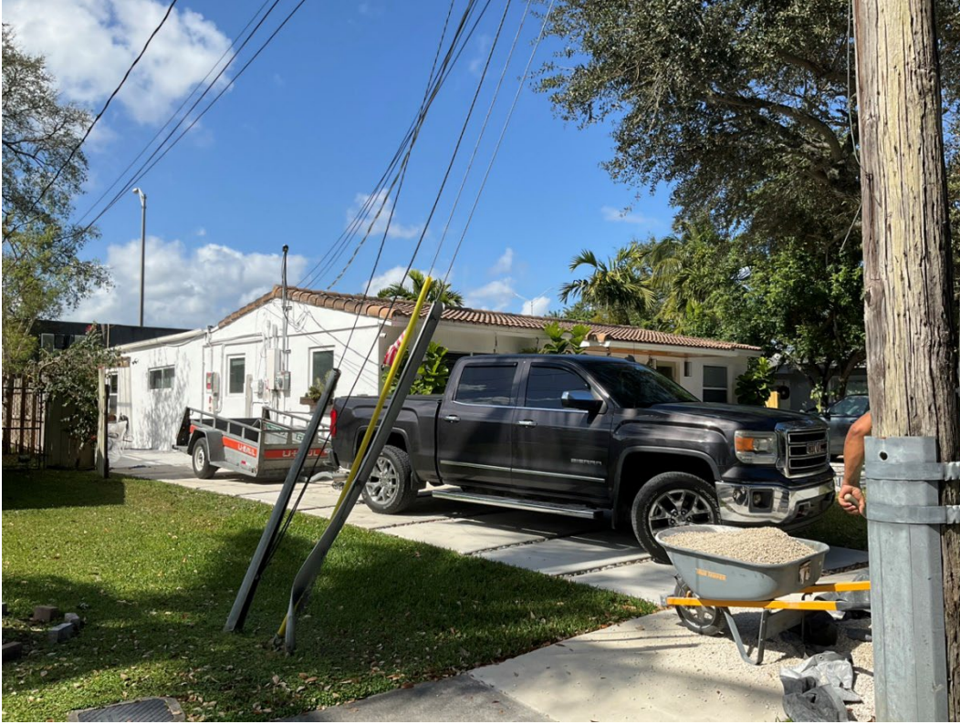
Figure 141. Photograph of 8BD11296, facing north.
