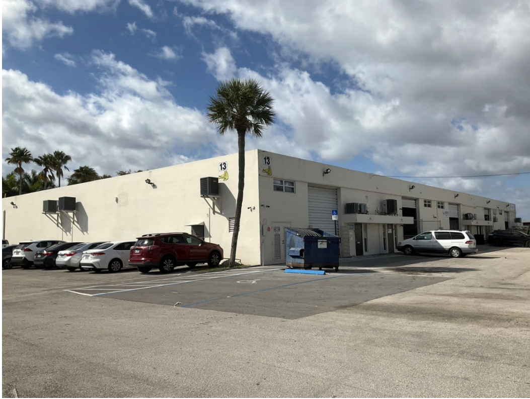
Figure 297. Photograph of 8BD11321, facing southwest.
