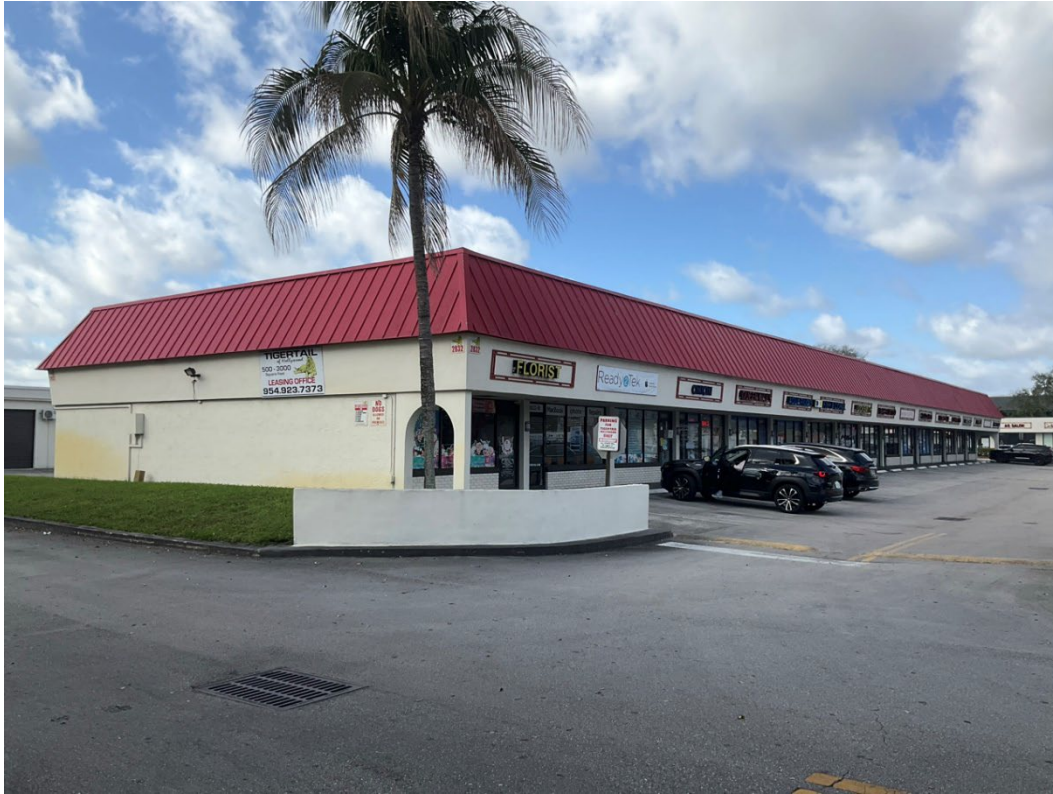
Figure 273. Photograph of 8BD11320, facing southwest (2 of 3).
