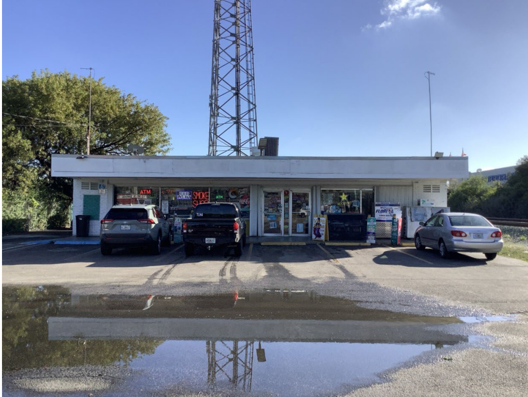
Figure 279. Photograph of 8BD10963, facing east.
