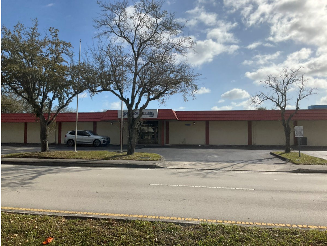
Figure 223. Photograph of 8BD11315, facing east.
