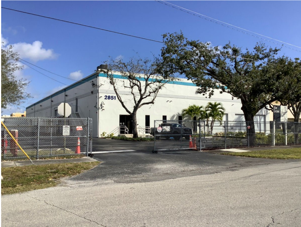
Figure 241. Photograph of 8BD11318, facing northeast.
