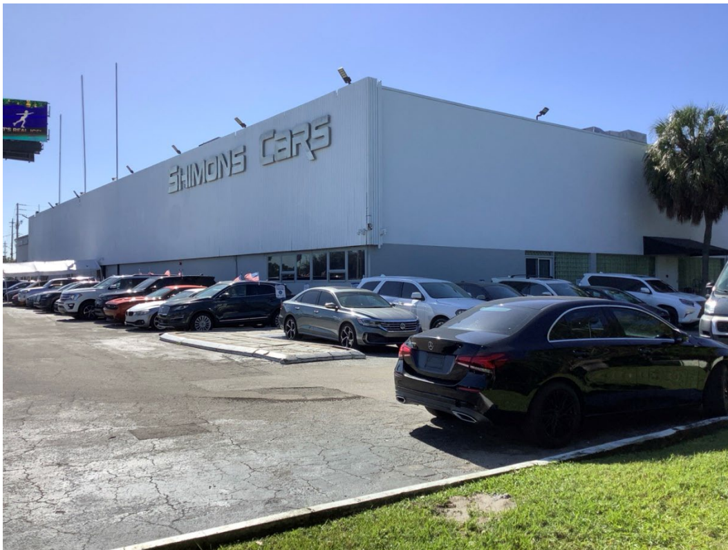
Figure 244. Photograph of 8BD10960, facing southwest (1 of 2).
