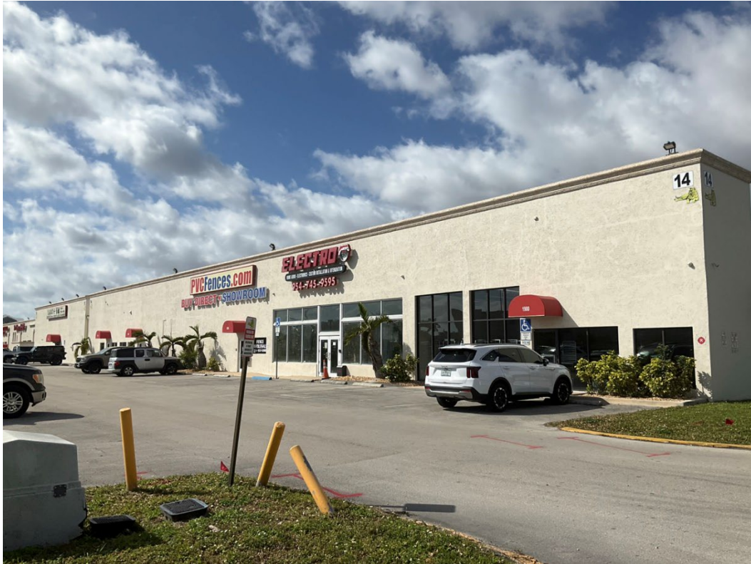
Figure 284. Photograph of 8BD09441, facing southwest.
