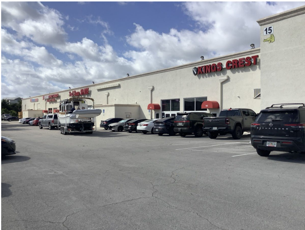
Figure 292. Photograph of 8BD09442, facing southwest.
