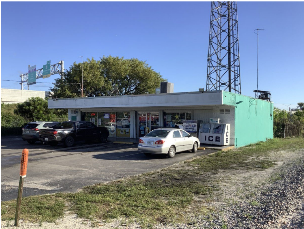
Figure 280. Photograph of BD10963, facing northeast.
