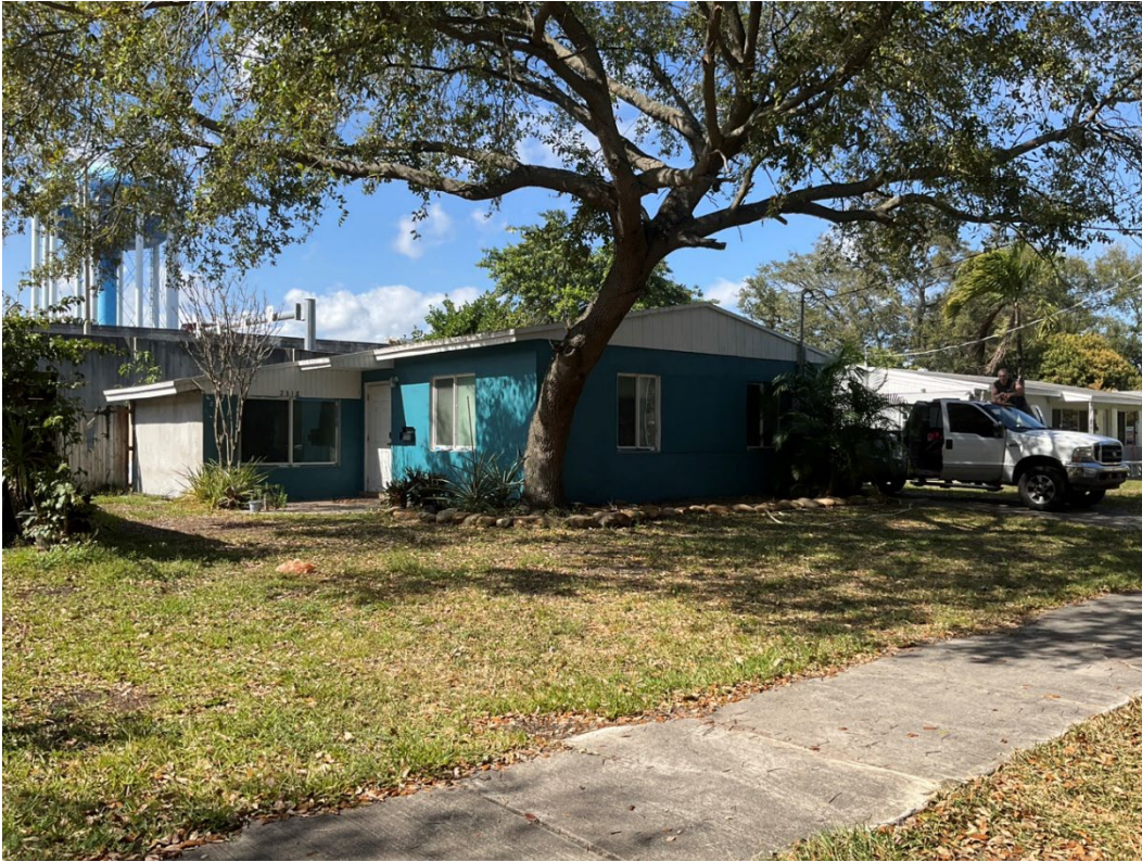
Figure 180. Photograph of 8BD11306, facing north.
