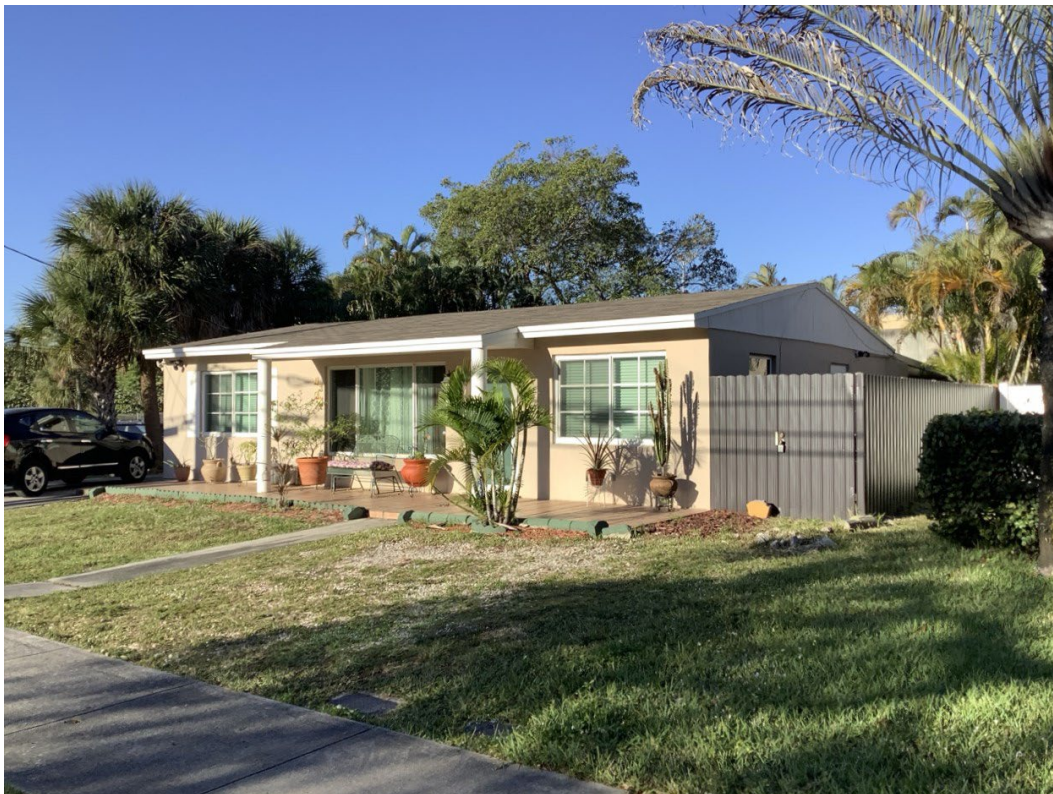
Figure 72. Photograph of 8BD10964, facing southwest.
