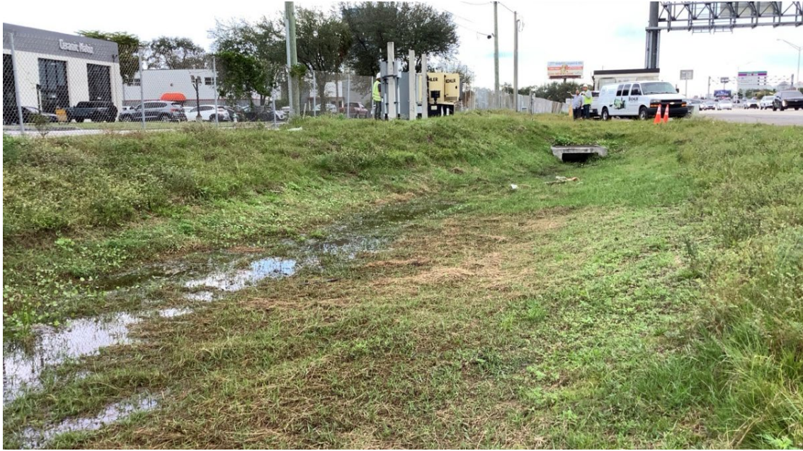
Figure 41. Overview of the APE facing northwest from STP 23 showing flooded drainage and subsurface utilities.
