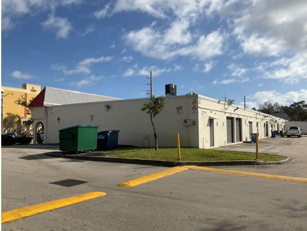
Figure 265. Photograph of 8BD11320, facing northeast.
