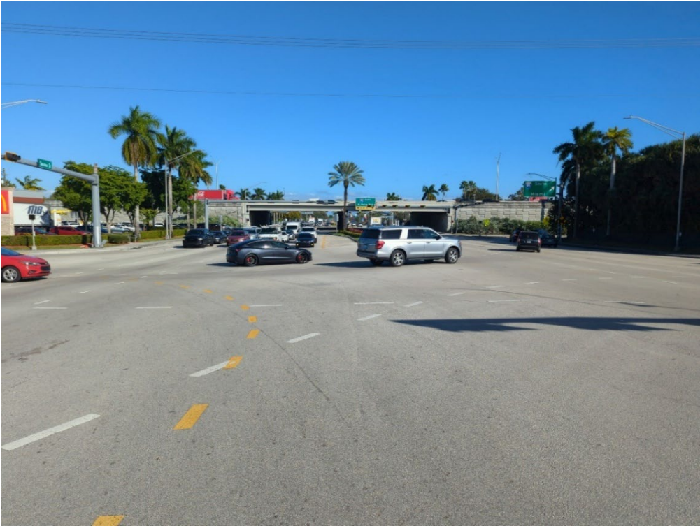
Figure 65. Photograph of 8BD07583, facing east.
