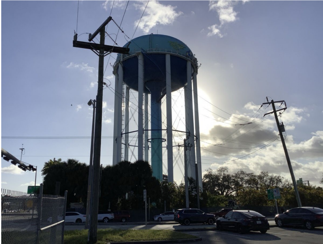
Figure 258. Photograph of 8BD11319, facing east.
