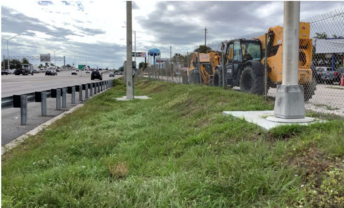
Figure 40. Overview of the APE near STP 32 facing south showing existing paved surfaces and buried utilities in the APE.
