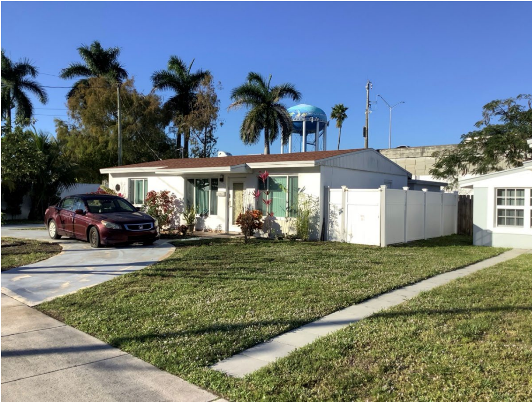
Figure 200. Photograph of 8BD10961, facing southwest.
