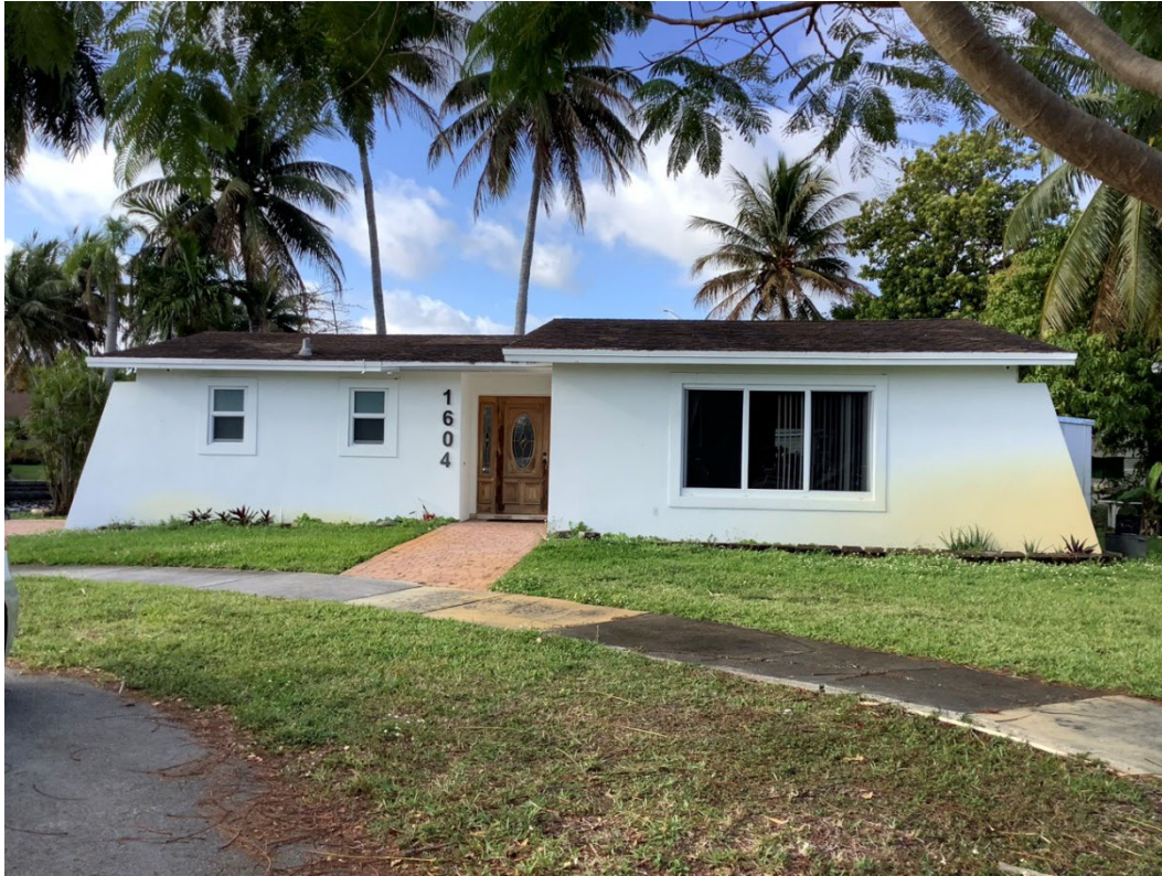
Figure 236. Photograph of 8BD11317, facing southwest.
