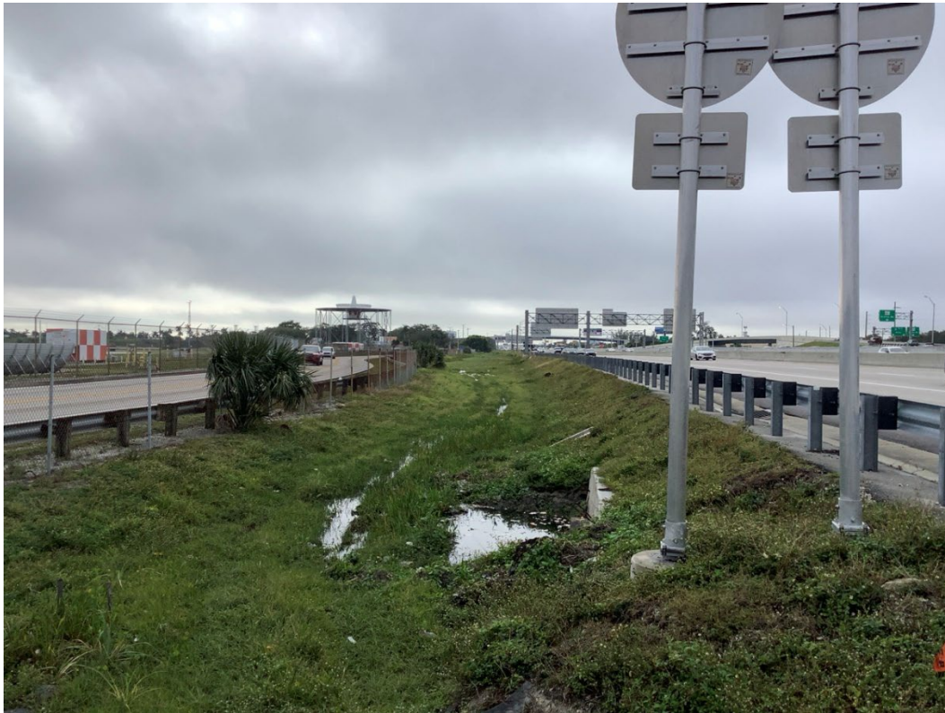
Figure 4. Northern end of the APE along West Perimeter Road, south of S.R. 595, facing south showing I-95 and roadside drainage.
