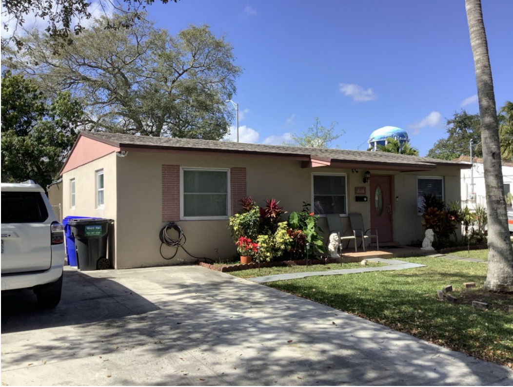
Figure 136. Photograph of 8BD11295, facing north.
