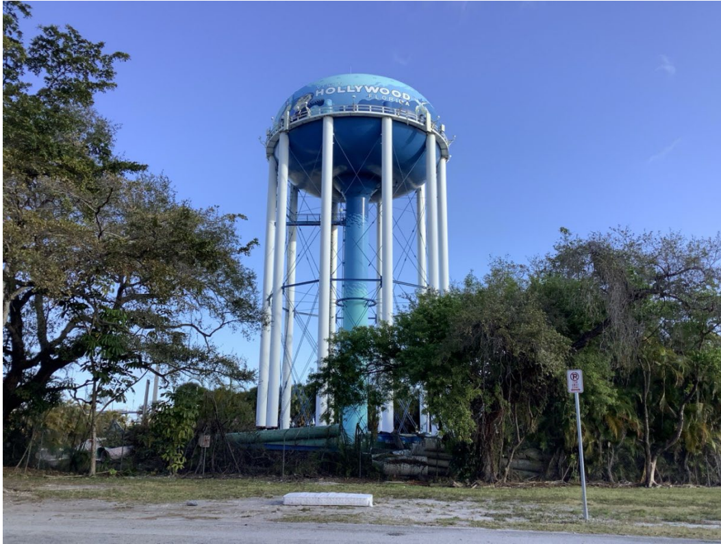
Figure 260. Photograph of 8BD11319, facing southwest.
