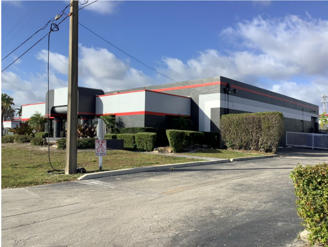
Figure 212. Photograph of 8BD11313, facing southwest.
