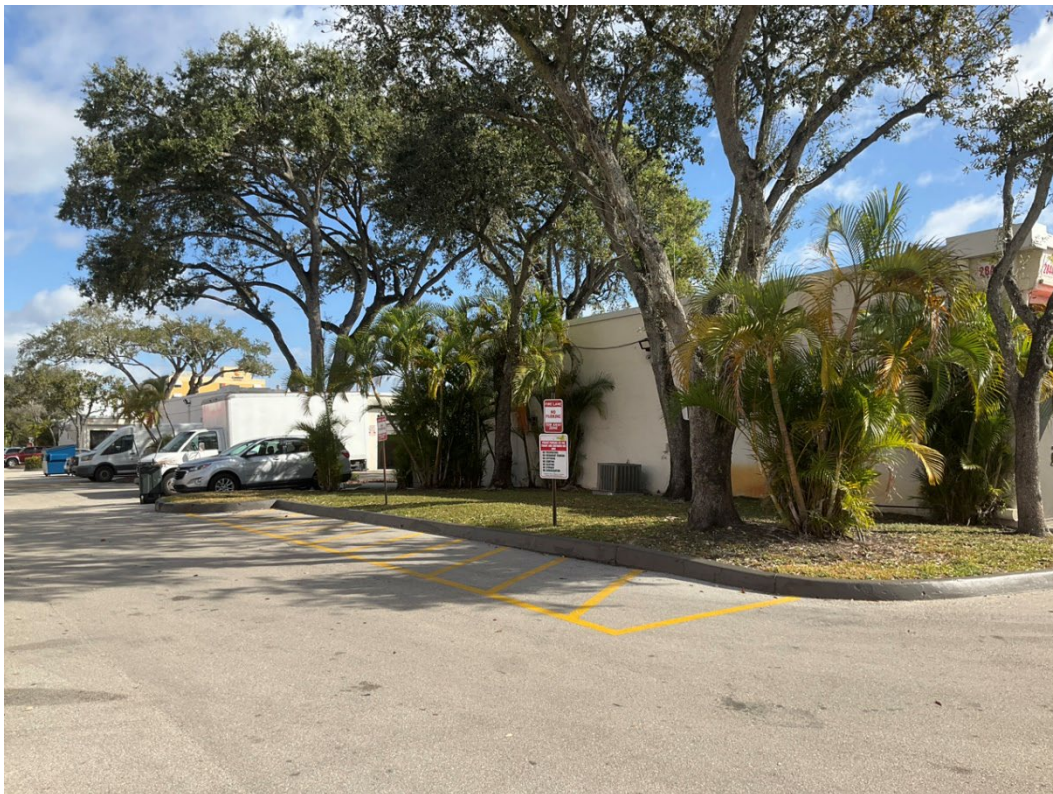
Figure 272. Photograph of 8BD11320, facing southwest (1 of 3).
