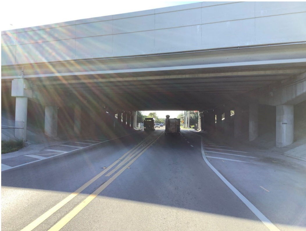
Figure 70. Photograph of 8BD10965, facing east.
