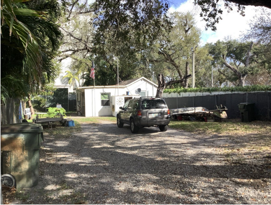
Figure 261. Photograph of 8BD08250, facing northeast.
