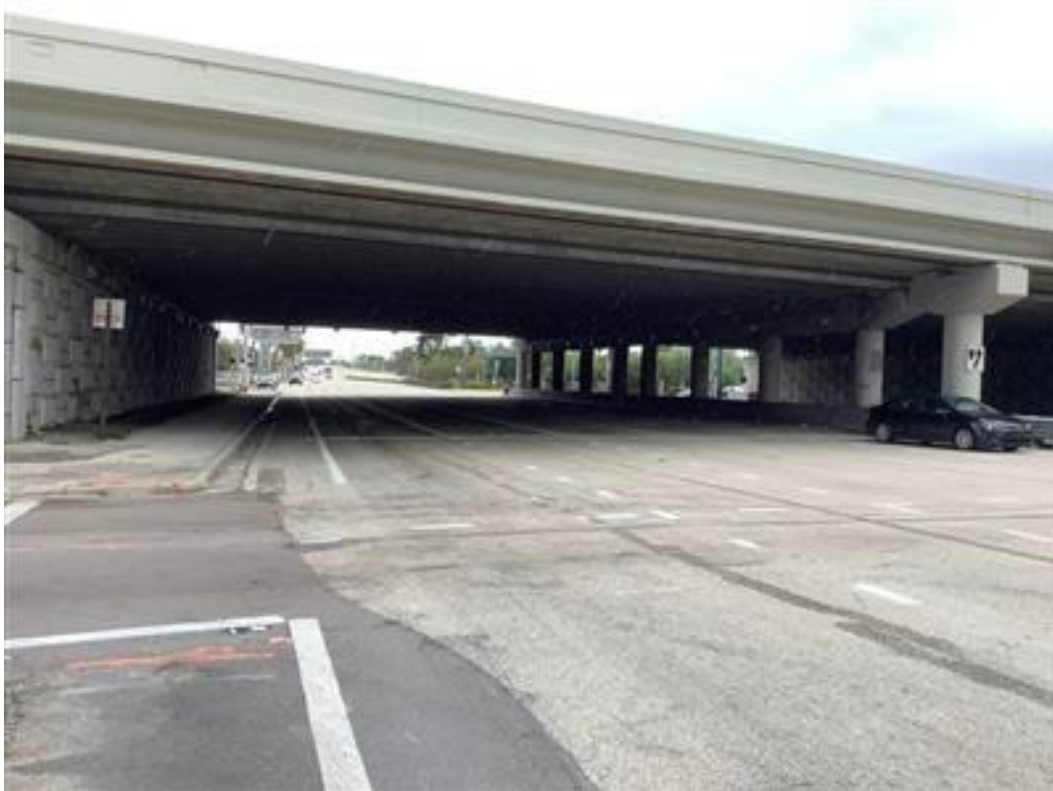
Figure 55. Photograph of 8BD04432, facing east.
