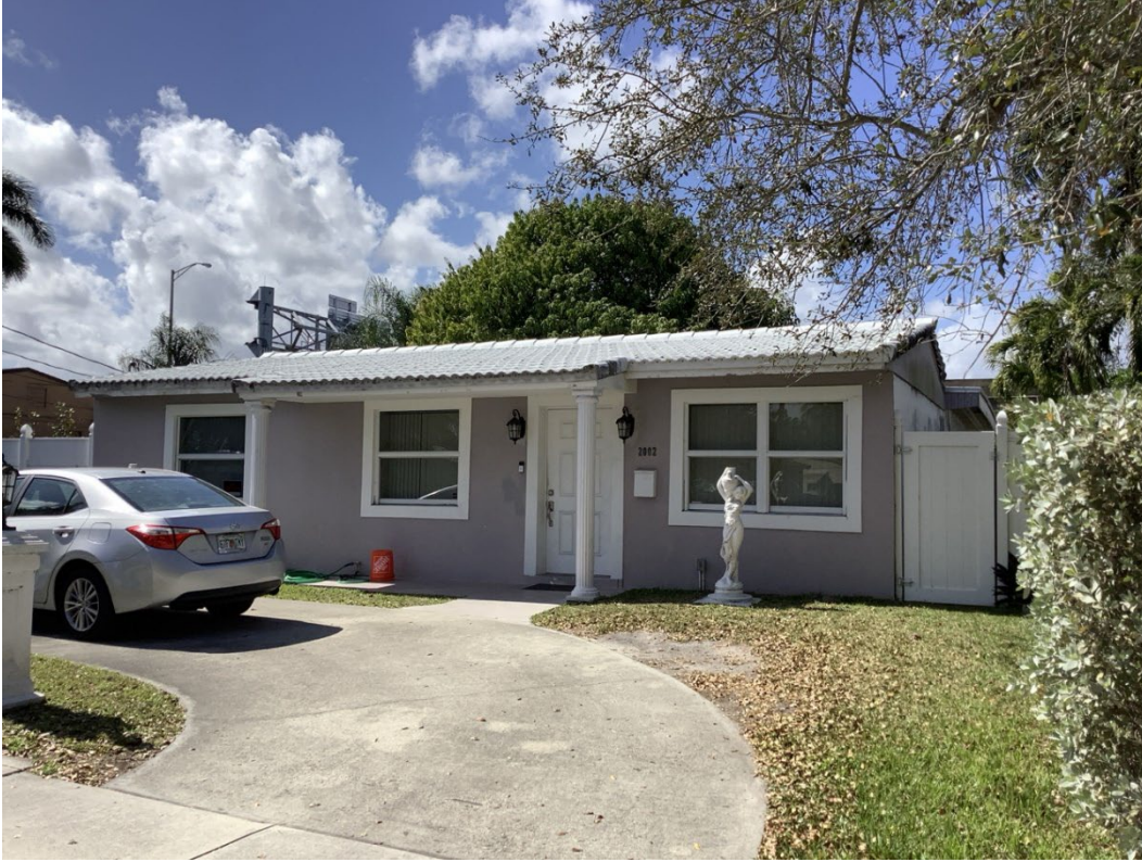
Figure 96. Photograph of 8BD11295, facing southwest.
