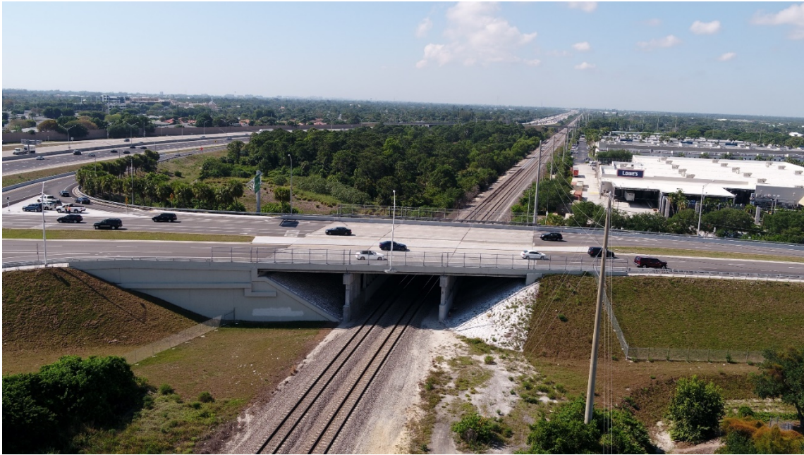
Figure 2-13: View looking South – Woolbright Road over SFRC (Bridge # 930300)
