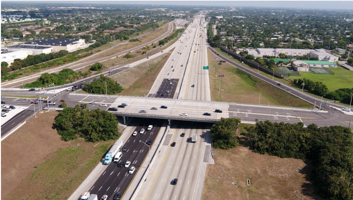
Figure 2-12: View looking North – Woolbright Road over I-95 (Bridge # 930301)
