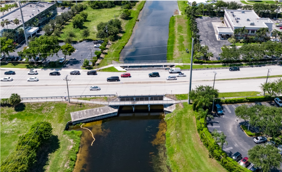
Figure 2-14: View looking South – Woolbright Road over E-4 Canal (Bridge #934461)
