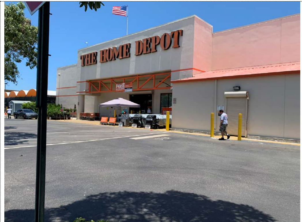
Photo 2 – View of Home Depot #6309, 1500-1520 SW 8th St., facing northeast.
