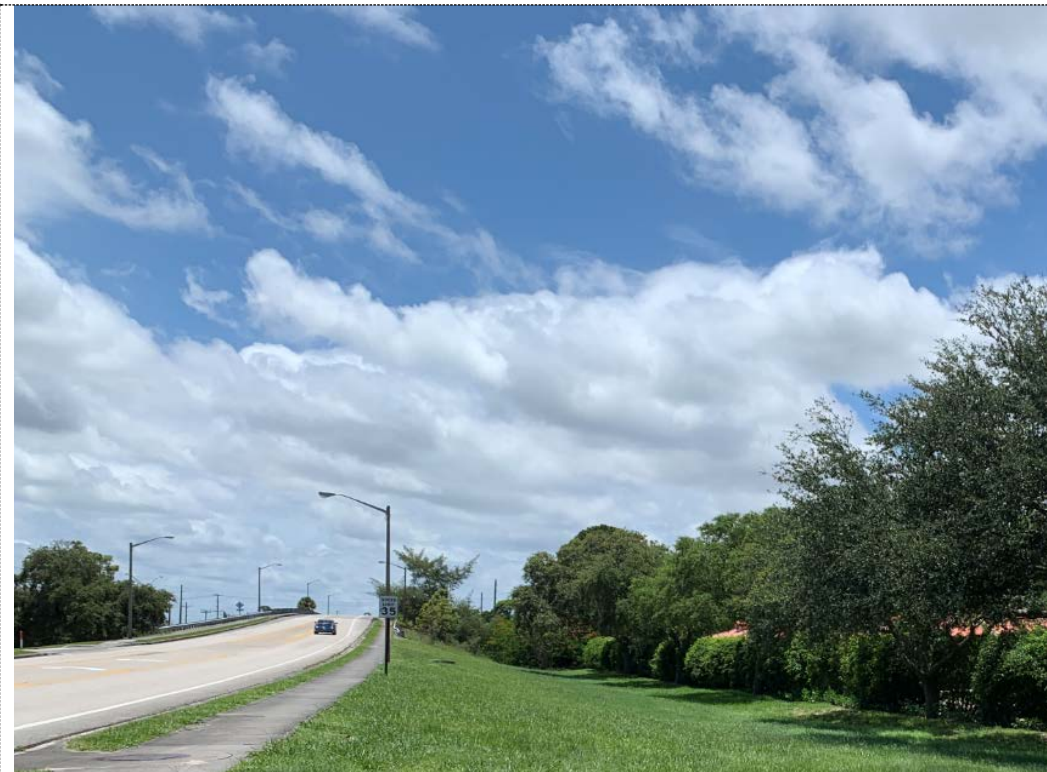
Photo 6 – View of Direct Transport-Delray Spill Atlantic Avenue & Woolbright Rd. site, facing west, showing SW 23 rd Street overpass over SR 9/I-95.
