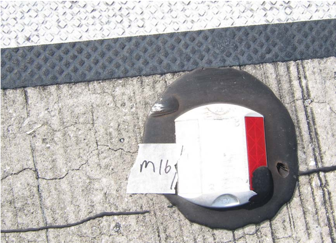
Upper Photo: Black Bitumen Sealant - Deck
