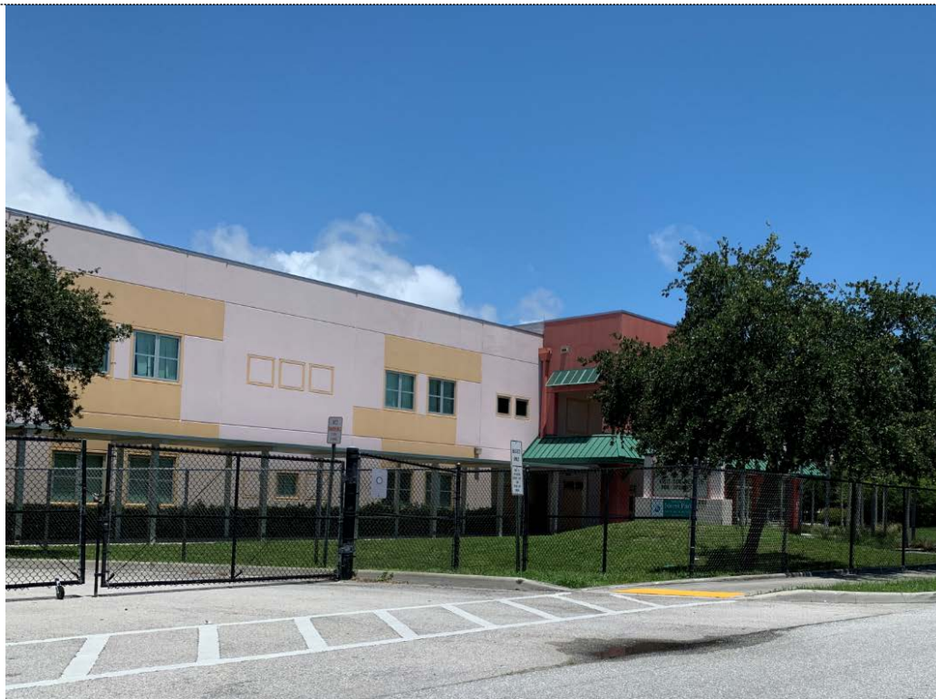
Photo 4 – View of Forest Park Elementary School, 1201 SW 3rd St., facing northwest.
